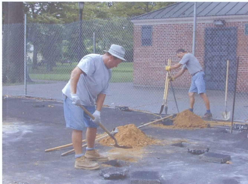
Wayanda Park – I footings excavations – note the clean fill
