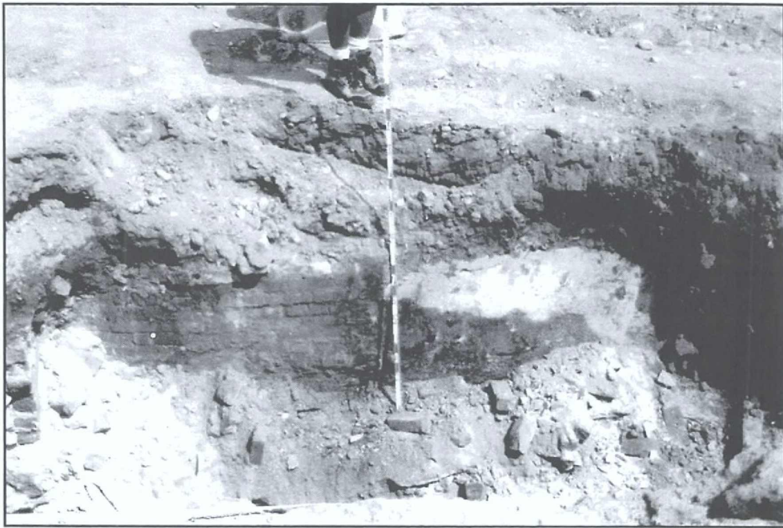
PLATE 1 - Trench 1, Brick and Mortar Foundation at the Back of the House on Lot 16, Facing North
