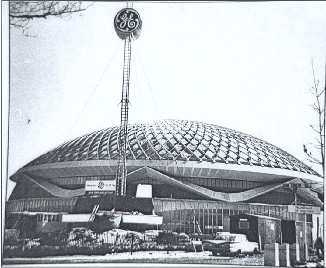
Figure 63. General Electric Pavilion, 1964 World's Fair. Flushing Bay Ecosystem Restoration Project, Queens County, New York (Bletter 1989).
