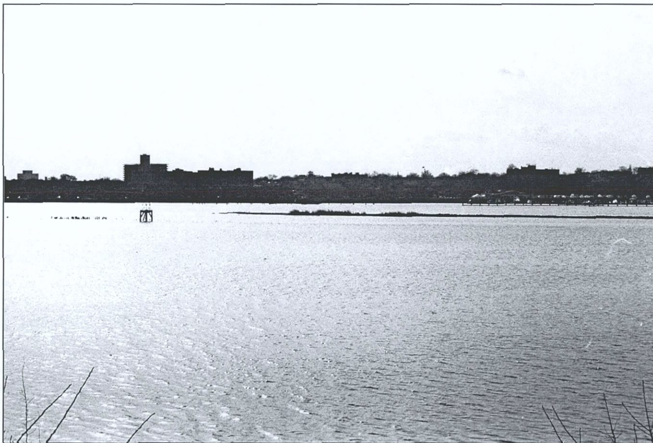
Figure 80. Possible remains of flushing bay dike (left center), southern end of LaGuardia Airport Dike (in center background), facing west. Flushing Bay Ecosystem Restoration Project, Queens County, New York (Pickman 2001).
