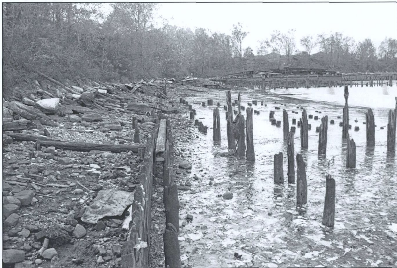
Figure 96. Shipyard Feature K (remains of wharf bulkheading at left) and Feature D (at right) from Figure 95, facing west. Note embankment at top left. Flushing Bay Ecosystem Restoration Project, Queens County, New York (Pickman 2002).
