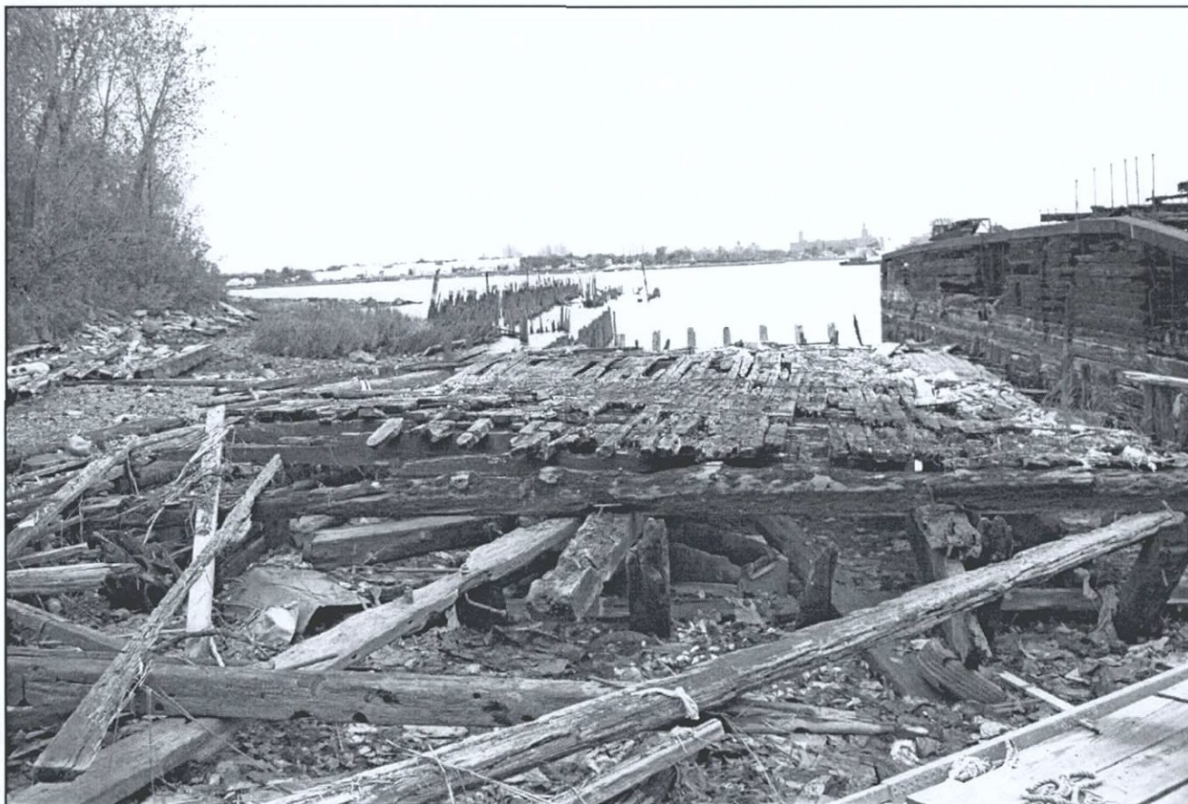
Figure 108. Shipyard Feature G1 (foreground), portion of Feature G (at right), and Features H and H1 (in background), facing north. Flushing Bay Ecosystem Restoration Project, Queens County, New York (Pickman 2002).
