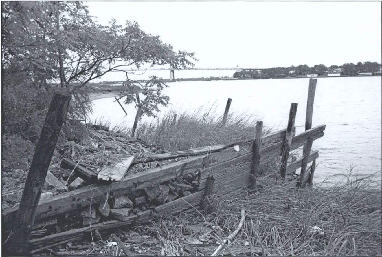
Figure 122. Remains of pier along west shoreline of Powell's Cove, facing northeast. Flushing Bay Ecosystem Restoration Project, Queens County, New York (Pickman 2002).
