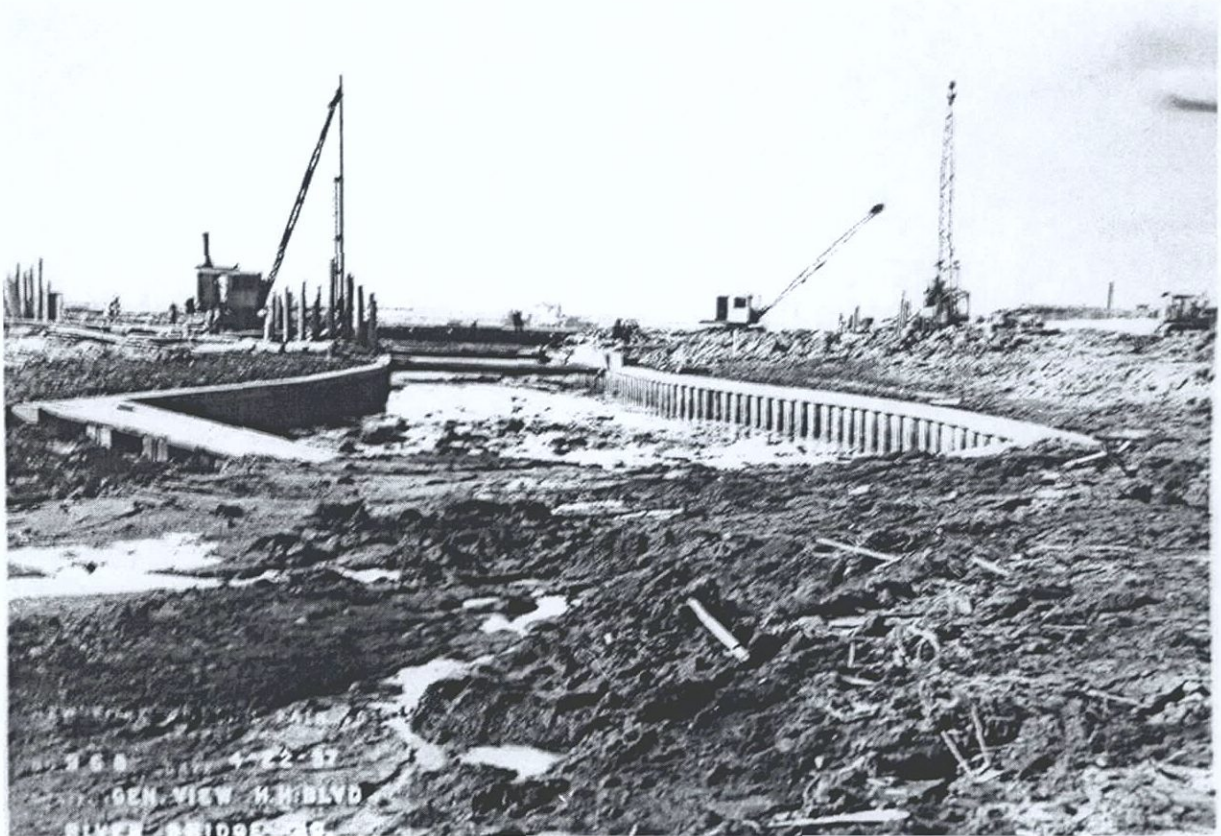
Figure 67. Construction of Meadow Lake Outlet. Flushing Bay Ecosystem Restoration Project, Queens County, New York ( World's Fair 1939/40 Corporation 1937b ).
