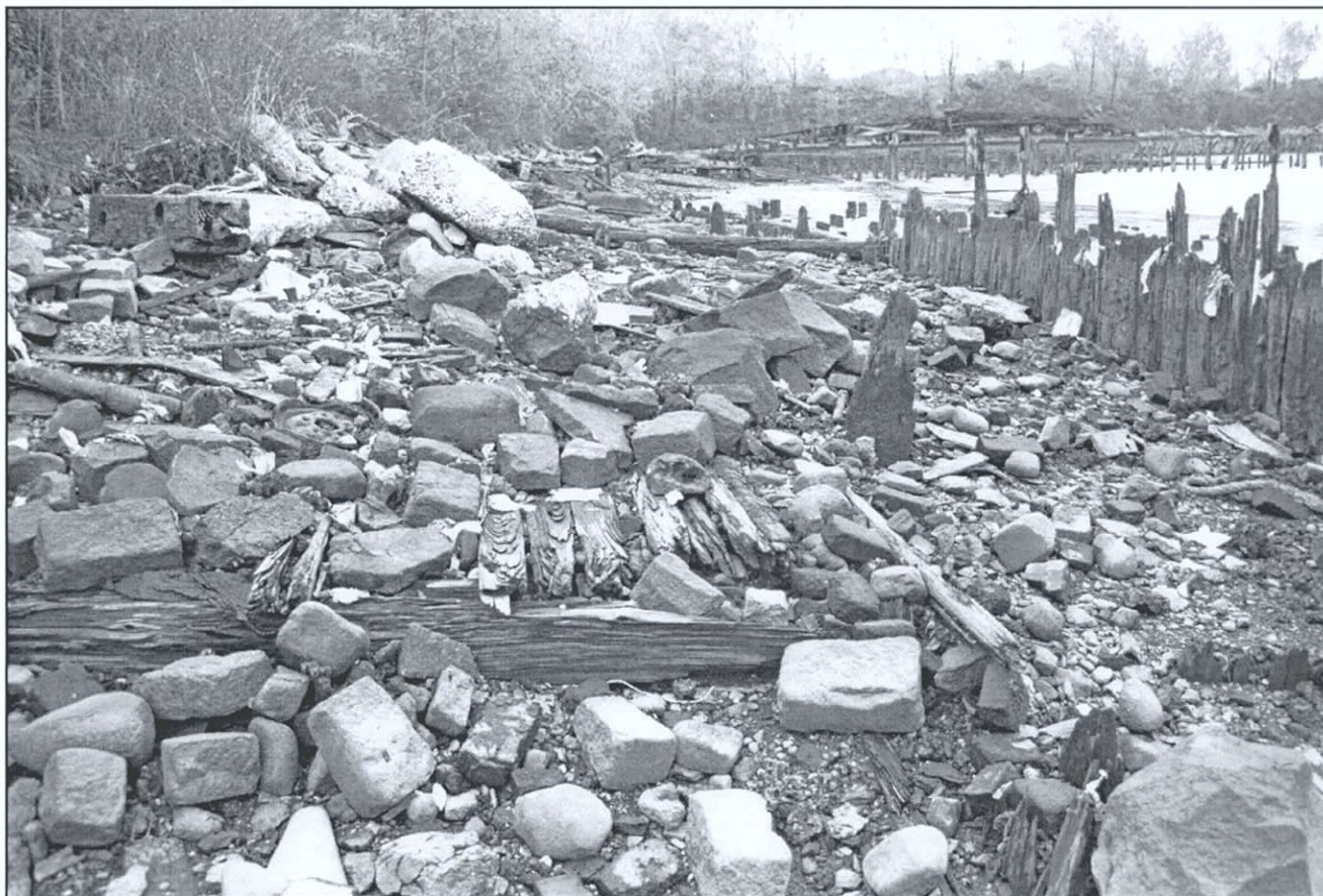
Figure 105. Shipyard Feature K, remains of wharf cribbing and bulkheading, facing west. Flushing Bay Ecosystem Restoration Project, Queens County, New York (Pickman 2002).
