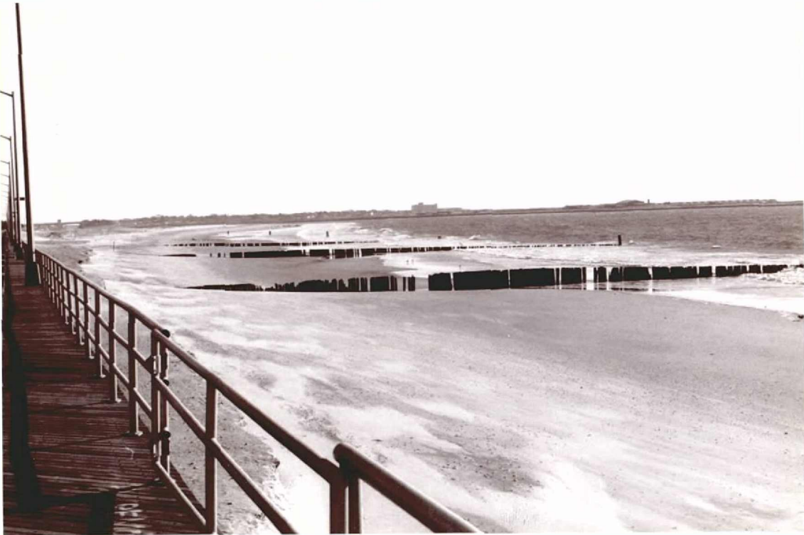
Figure 28. Remains of wooden groins, facing east from vicinity of Beach 35th Street. Cultural Resources Assessment of T-Groin Placement, Queens County, New York ( Pickman 1999 ).
