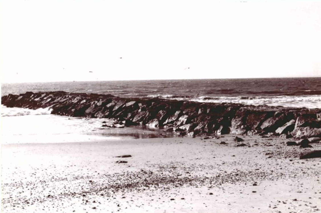
Figure 32. Rubble mound groin in the vicinity of Beach 36th Street, facing southwest. Cultural Resources Assessment of T-Groin Placement, Queens County, New York (Pickman 1999).
