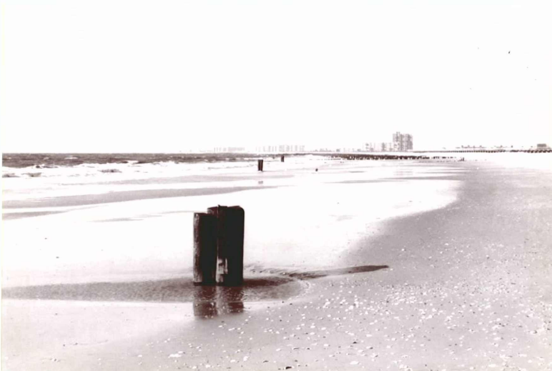
Figure 31. Pilings at the end of the buried wooden groins, facing west from vicinity of Beach 26th Street. Cultural Resources Assessment of T-Groin Placement, Queens County, New York (Pickman 1999).
