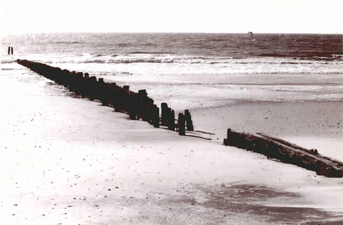
Figure 29. Remains of wooden groin, facing southwest between Beach 32nd and Beach 33rd Streets. Cultural Resources Assessment of T-Groin Placement, Queens County, New York ( Pickman 1999 ).
