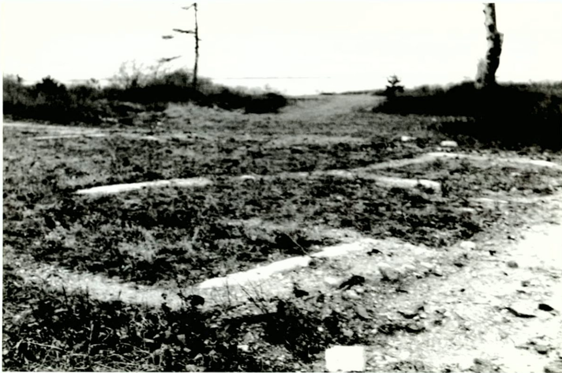
Figure 113. Foundation of Boissert/Heinsheimer House, facing northwest. Jamaica Bay Restoration Project, Kings, Queens and Nassau Counties, New York (Pickman 1999).
