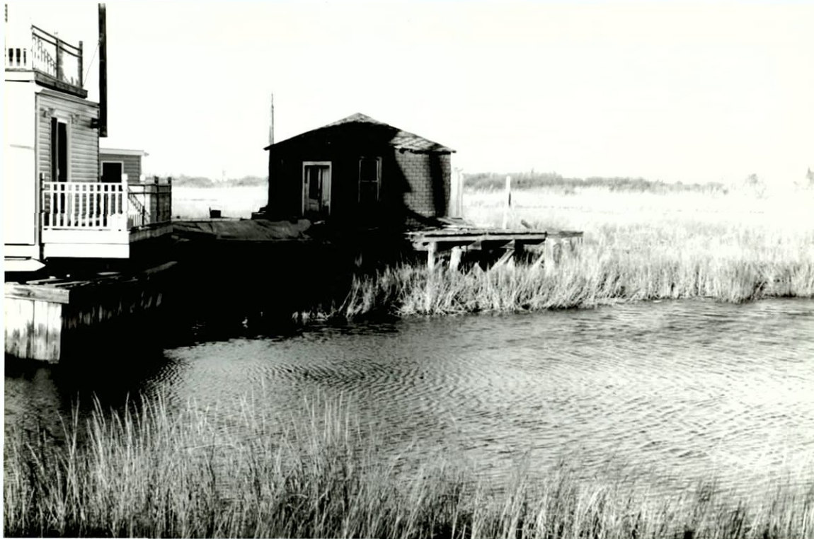
Figure 142. Structures on pilings east of Cross Bay Boulevard and south of the culvert, facing north. Jamaica Bay Restoration Project, Kings, Queens and Nassau Counties, New York (Pickman 1999).
