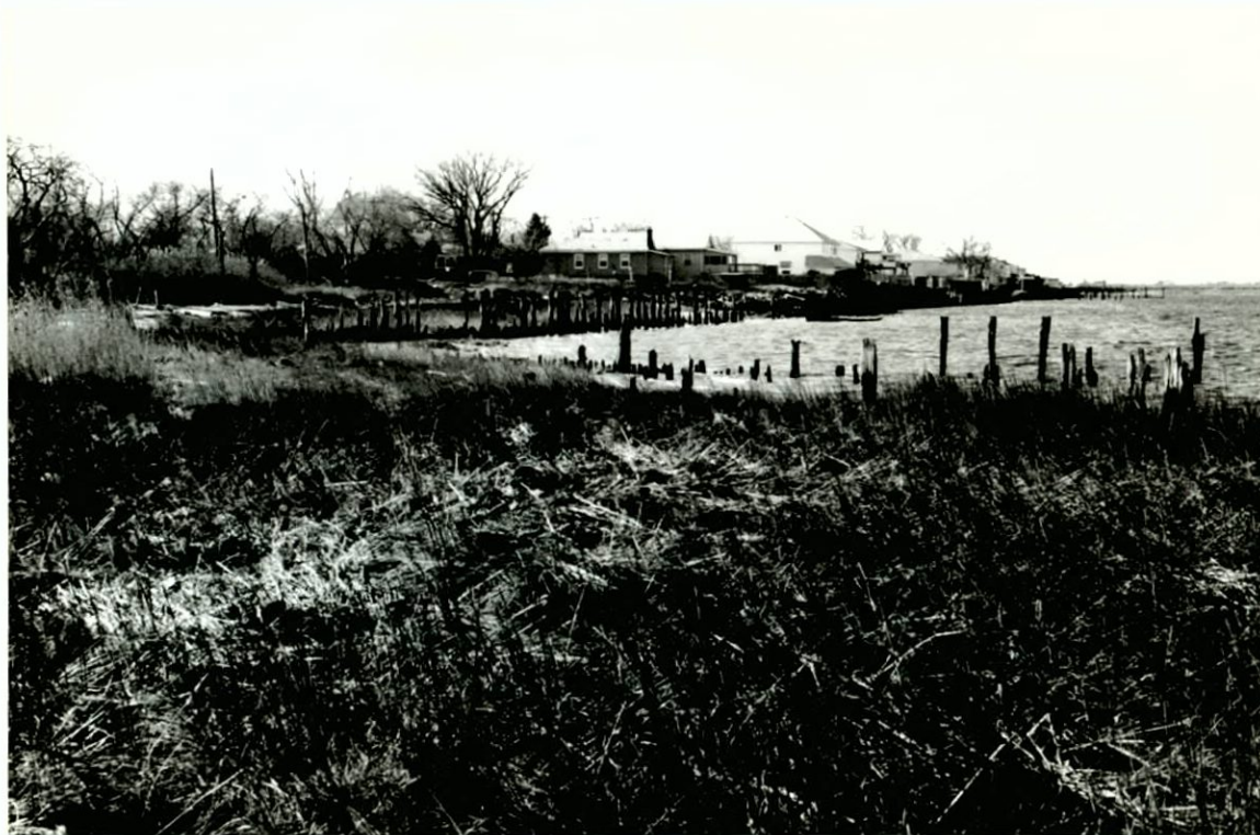
Figure 127. Remains of wooden bulkheading at Dubos Point, facing southwest. Jamaica Bay Restoration Project, Kings, Queens and Nassau Counties, New York (Pickman 1999).
