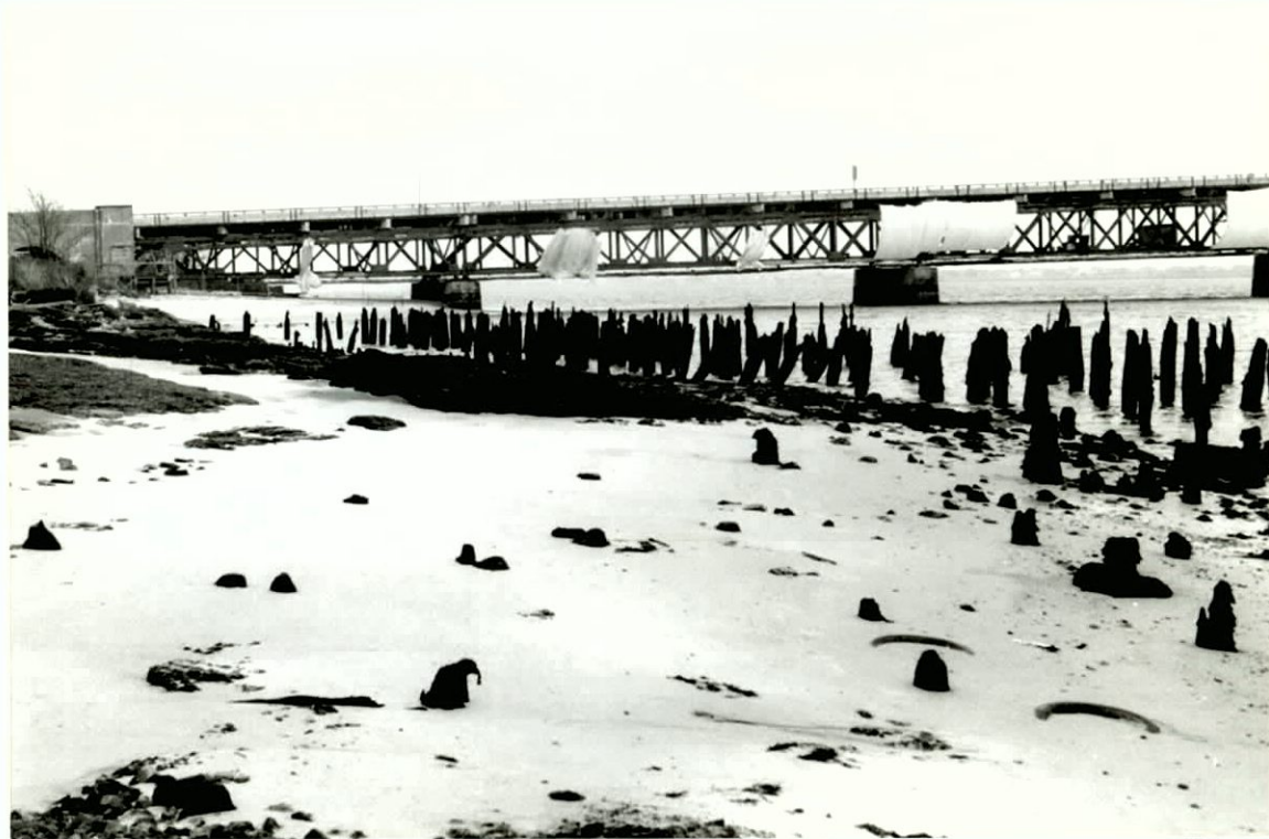
Figure 45. Remains of bulkheading on south shore of Barren Island, near the White factory site, facing east. Jamaica Bay Restoration Project, Kings, Queens and Nassau counties, New York (Pickman 1999).
