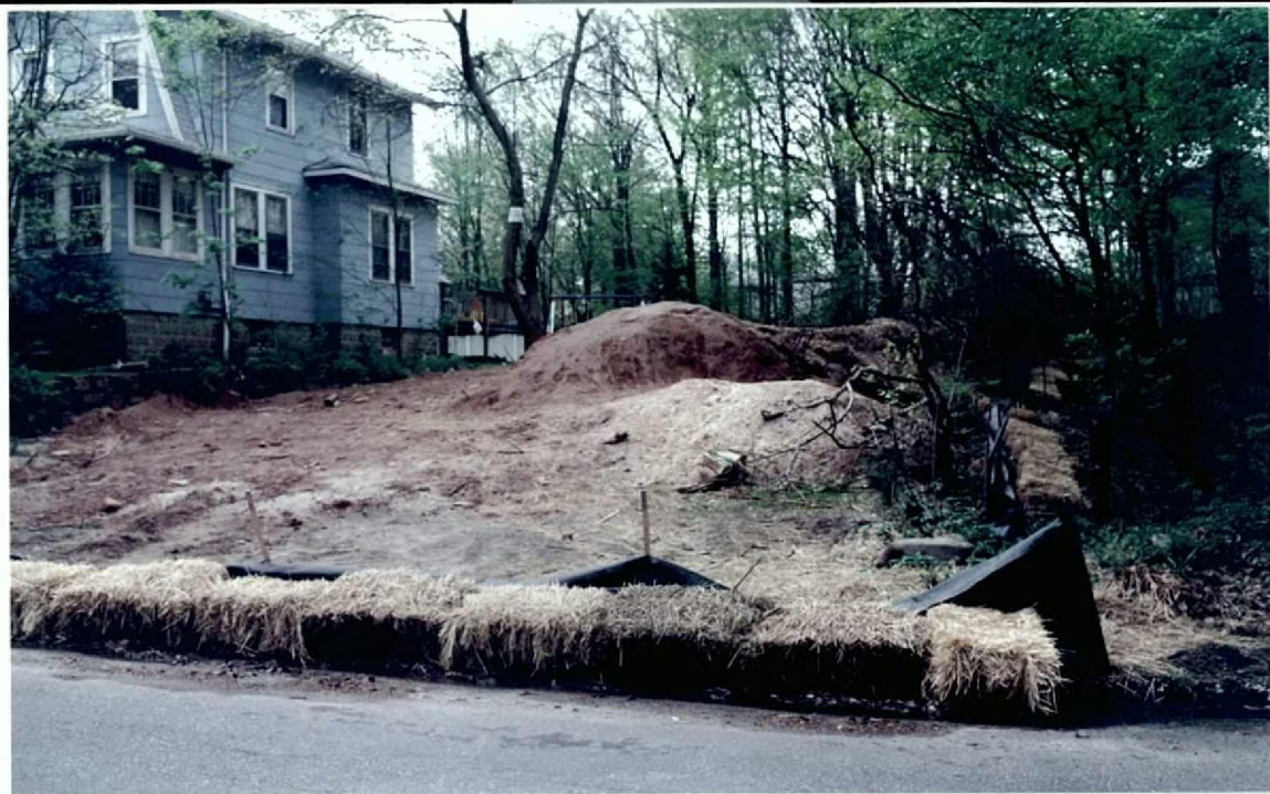
Photo 2: Fill has been deposited on a portion of the site for the septic system. Silt fence in foreground. View to northeastern corner of lot. Stream is to right in photo.
