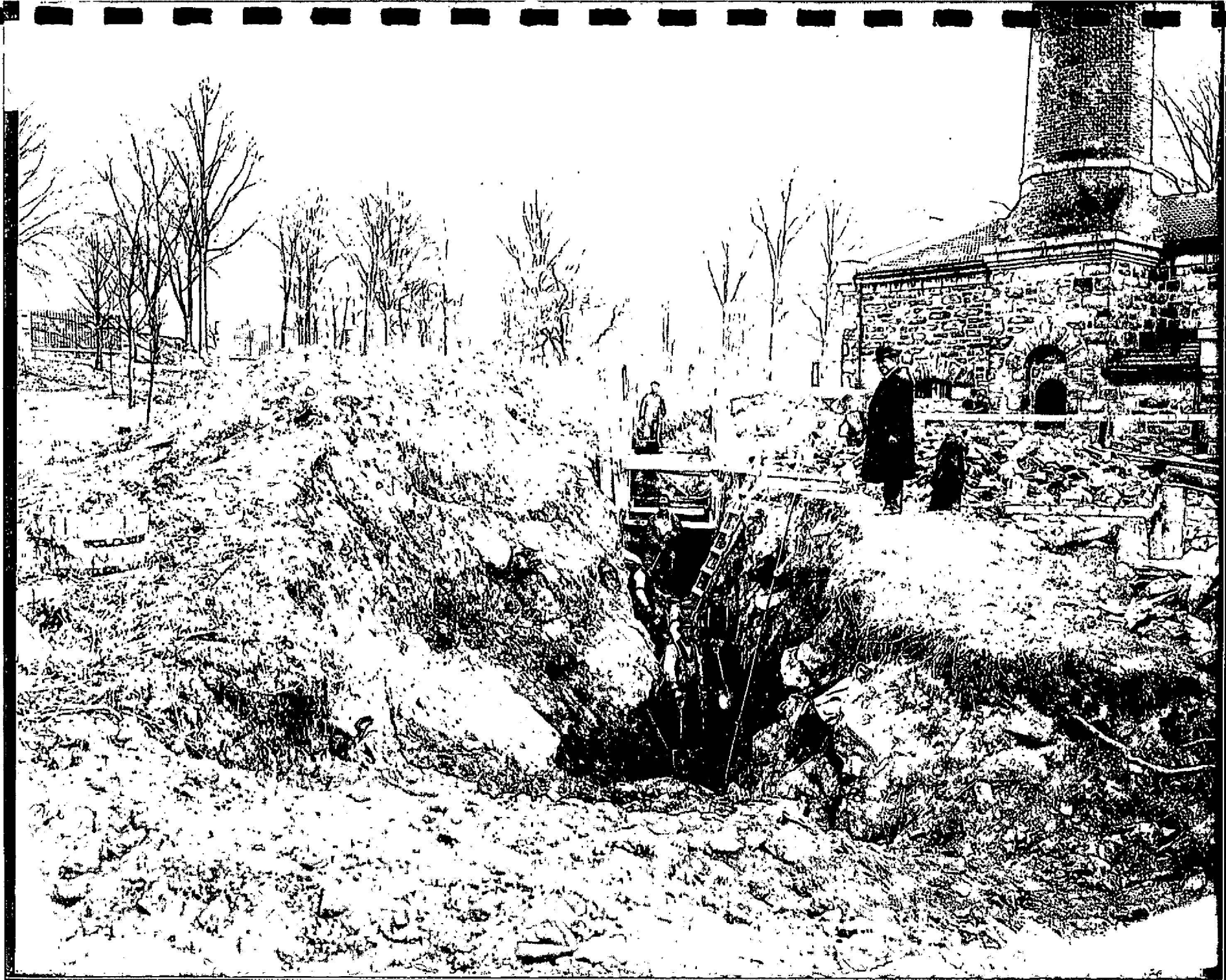
ILLUSTRATION 2: Trench for power line connection, powerhouse to conservatory. NYBG Negative N2969, 1915.
