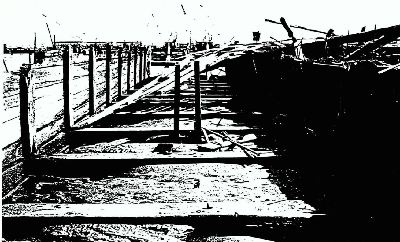
PHOTO AA: Vessel 24, view east along the centerline of the vessel toward its stern. At the sides of the picture are two longitudinal bulkheads which formed part of the hull structure, about halfway between the centerline and the sides of the hull. These bulkheads consist of thick timbers piled on each other; they are bolted to each other and to the vertical posts alongside. The two vertical posts in the center of the photo helped steady a vertical post (now entirely missing) that extended up to the roof of the deckhouse. (Neg. 404-15)
