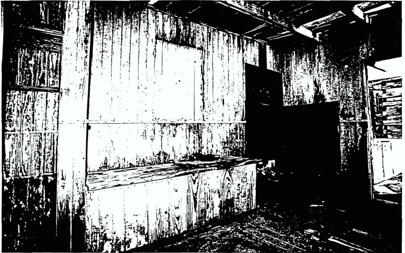
PHOTO D: Vessel 1, view northeast, showing interior of cabin. The wall on the left backs onto the covered cargo space. Just right of center is the space for the stove, with wall protected by metal. Left of center is the coal bunker, also used as a bench. To right is the doorway to the bedroom. The walls are faced with vertical tongue-and-grove boards. (Neg. 401-25)
