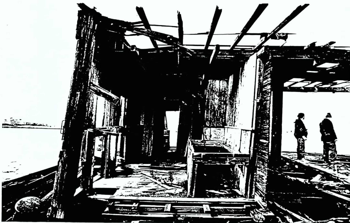
PHOTO E: Vessel 1, view northwest, showing interior of cabin as seen from vessel 2. The southeast (starboard) wall of the cabin is entirely missing, allowing the camera to look directly into the cabin from outside, and showing how the cabin was built within the barge's deckhouse, with the cabin's ceiling located about 2.5 ft. below the crossbeams of the deckhouse roof. To the right is a bunk attached to the wall. The two members of the survey team are standing in the former cargo space of the deckhouse. (Neg. 101-15)
