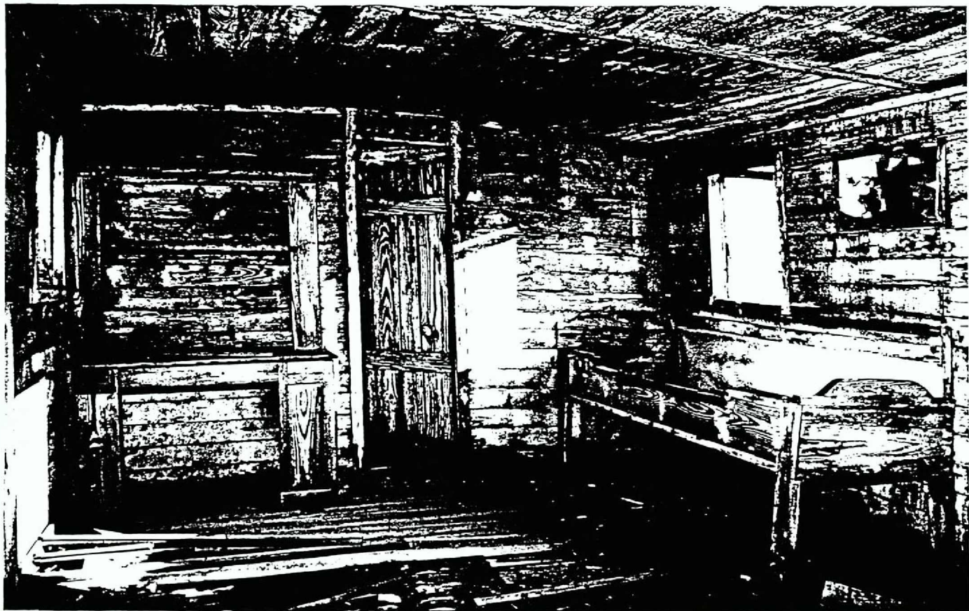
PHOTO N: Vessel 7, view south, showing interior of north room of cabin. To the right is a carved wooden bunk. Unlike other cabins, the wall lining here consists of horizontal boards. (Neg. 402-27)
