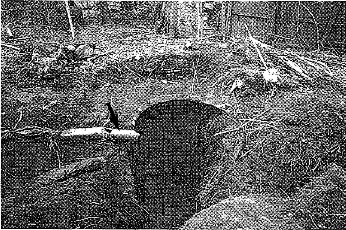
11 Beehive-domed, mortared brick cesspool with a terra-cotta-pipe (arrow), broken by the backhoe but in place, discovered in TT1. Although the brick dome was broken, the open-bottomed feature was well made. The backhoe broke away the western brick wall to test the deposit inside which was virtually sterile fill. (3/18/97)
