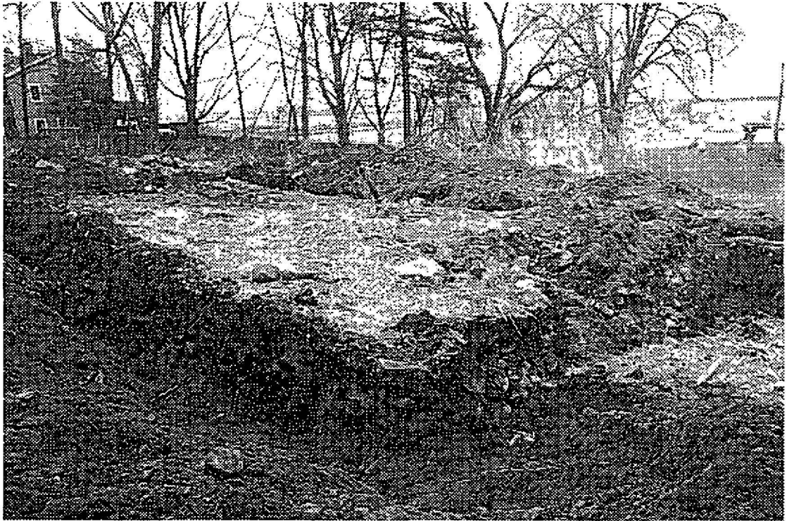
4 Northwest corner of the original Poillon house foundation exposed in foundation trench 1 (FT1) on the right and 4 (FT4) on the left. The view is south toward Great Kills harbor. (3/17/97)
