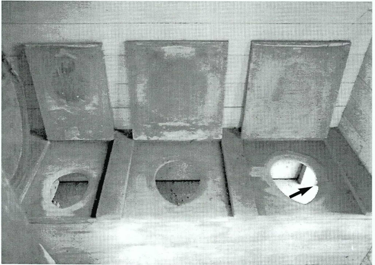
24 Indoor privy in the Gericke (Winant) farm carriage house. The "three seater" appears to accommodate adults and children (the seat on the left is noticeably smaller than the other two). The light comes through an above-ground access hole (arrow) on the side of the building. This was undoubtedly a means of cleaning what appears to be a very shallow privy that may have accommodated a trough or tray that collected human waste for fertilizer. (Geismar 5/88)
