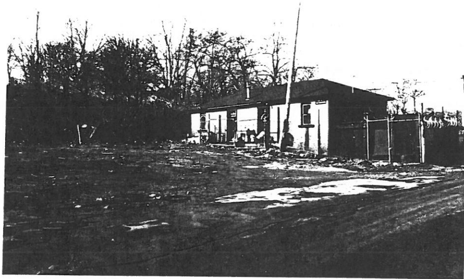
Plate 2 : View of former paint shop structure west of Edgewater Street looking northwest.
