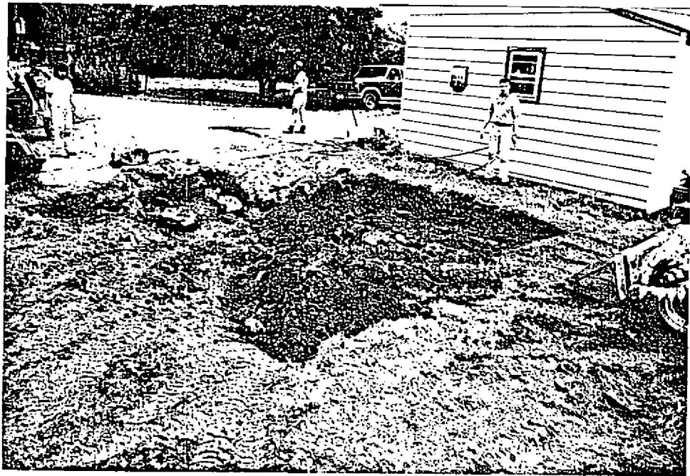
Plate 8 - Tests 3 and 4 after excavation, viewed from southeast
