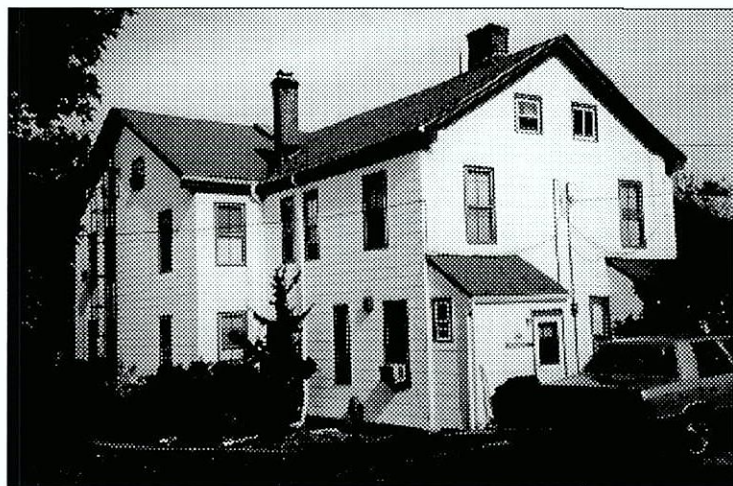
Figure 6.132 Typical rear facade of duplex. Note numerous electrical wires, window AC units, and inconsistency in window storm units.
