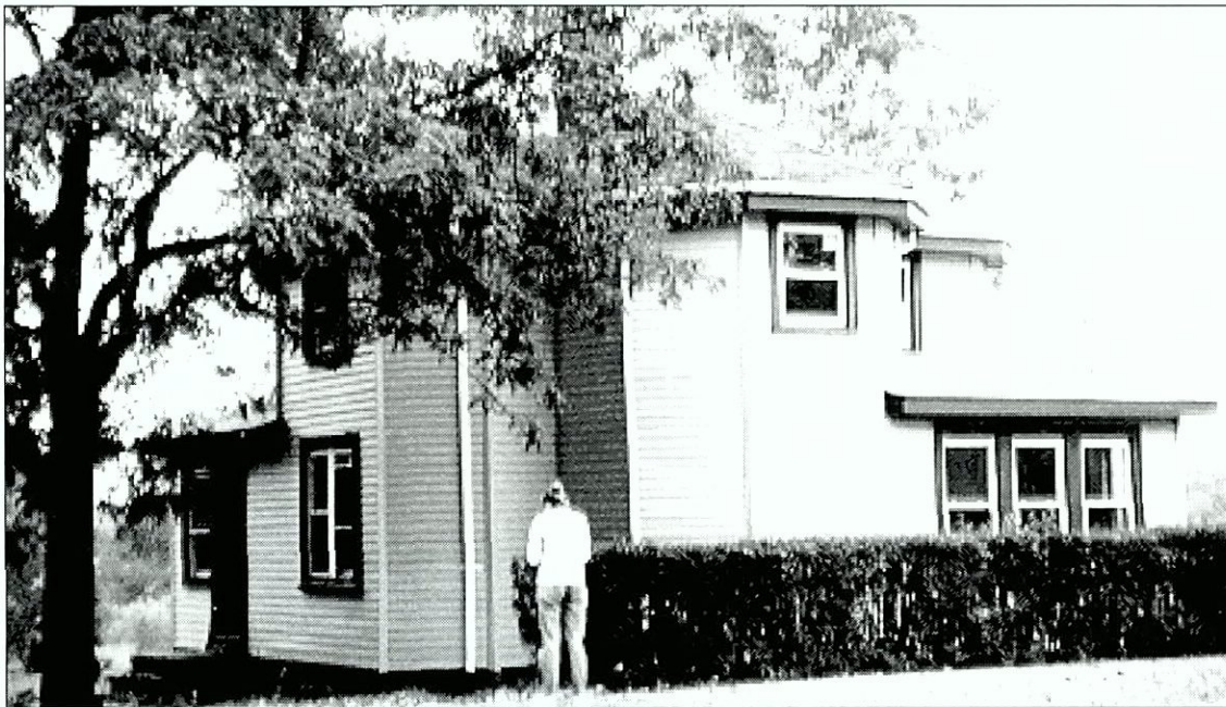
Figure 6.170 General view of building 406 showing the north and east elevations. Note enclosure of porches and the covering of windows with vinyl siding.
