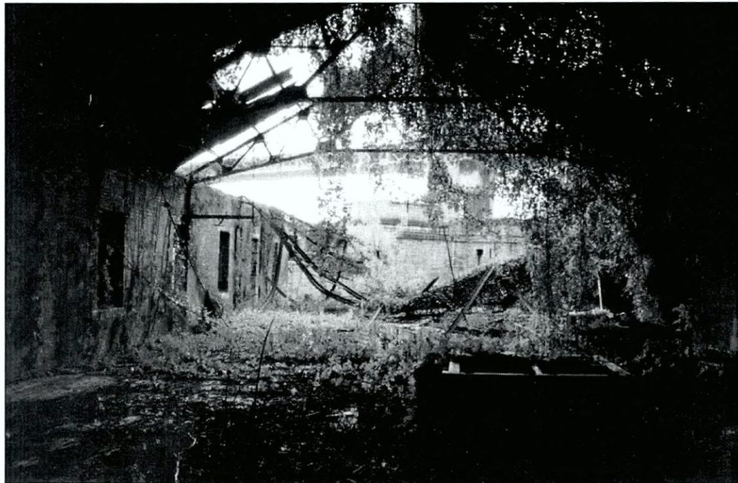
Figure 6.62 Interior of Torpedo Storage Building looking east out the fire-damaged portion of the building. Note the structural failure and collapse of steel roof trusses and the intrusion of ivy.
