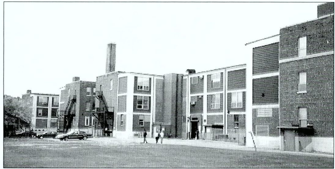
Figure 6.143 West facade of Building 210 showing enclosure of three-story open porch.
