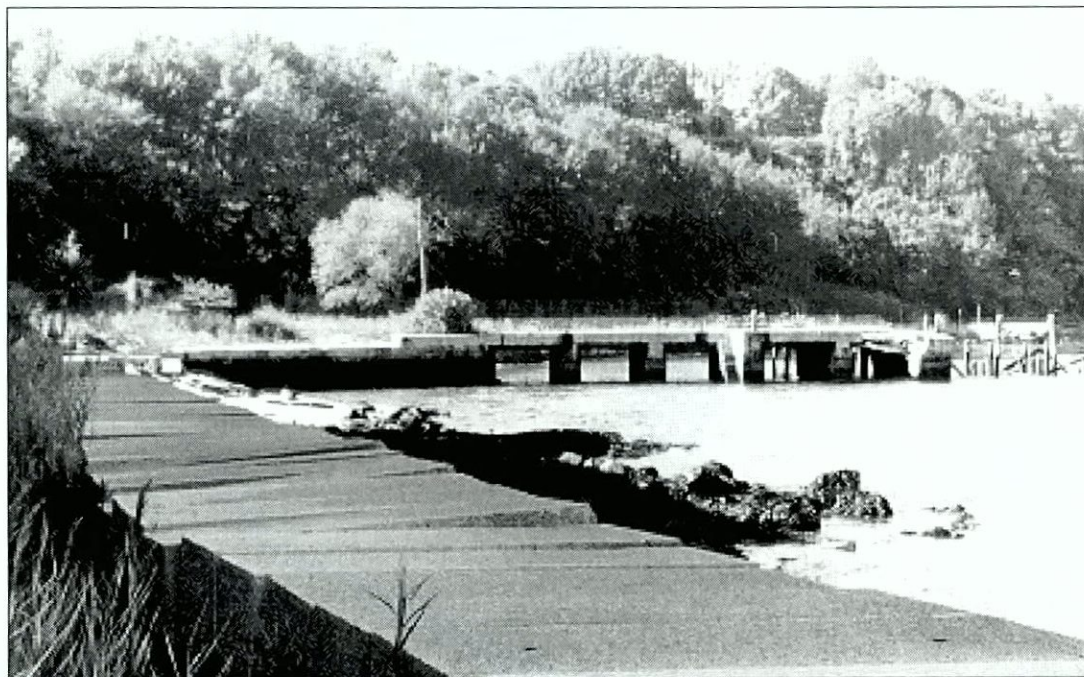
Figure 6.50 View of seawall with dock in the distance. Note undulating shifting of capstones caused by the constant impact of ocean waves.
