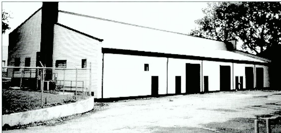
Figure 6.163 Building 301 showing the west and south facades.. Recent sheathing with vinyl siding has altered the original fenestration and stepped gable ends.
