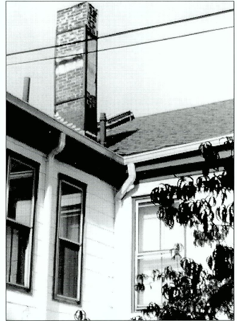
Figure 6.137 Poor repair of typical chimney resulting in poor repointing, patching, and structural bracing with corrosive metal angles. Inappropriate and inefficient placement of down spouts.
