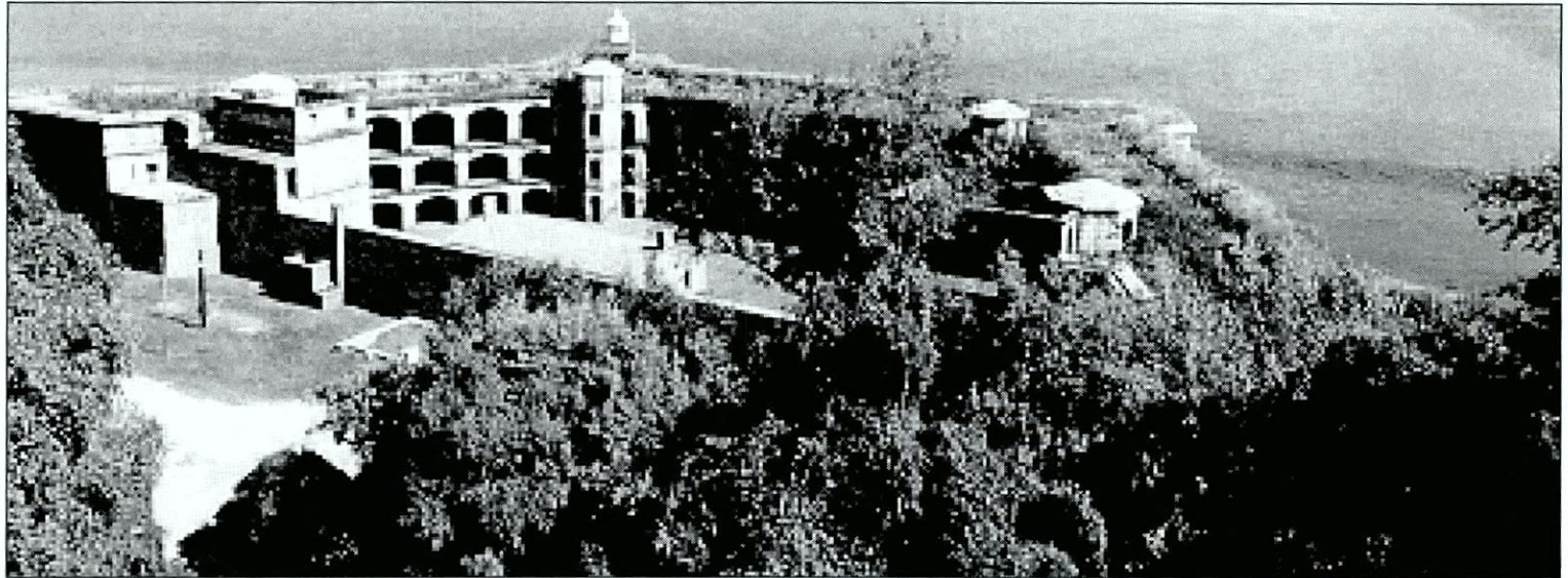
Figure 6.12 General view of Battery Weed
