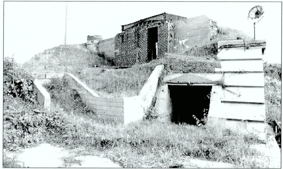
Figure 6.86 Look-out complex located at the southeast corner of Tompkins' barbette. Portion of building removed. General deterioration of concrete and brick. Vegetation entering interior through doorway.
