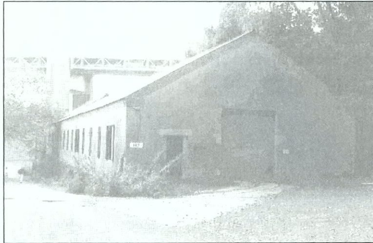
Figure 6.58 General view of Torpedo Storage Building showing north and west facades. Verrazano Narrows Bridge is in the background.
