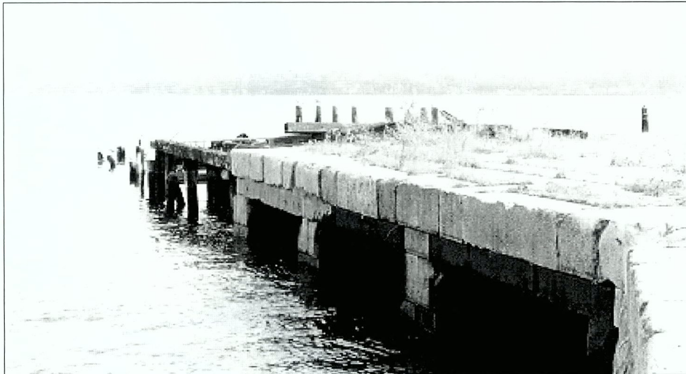
Figure 6.45 General view of North Dock showing deteriorated condition at the end and the intrusion of vegetation through the joints in the masonry deck.
