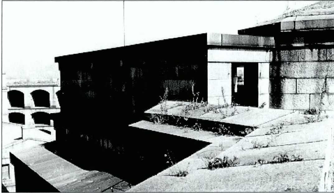
Figure 6.24 General view of granite copingstone at the southwest corner of Battery Weed. Volunteer vegetation growing out of vulnerable mortar joints throughout the parapet.
