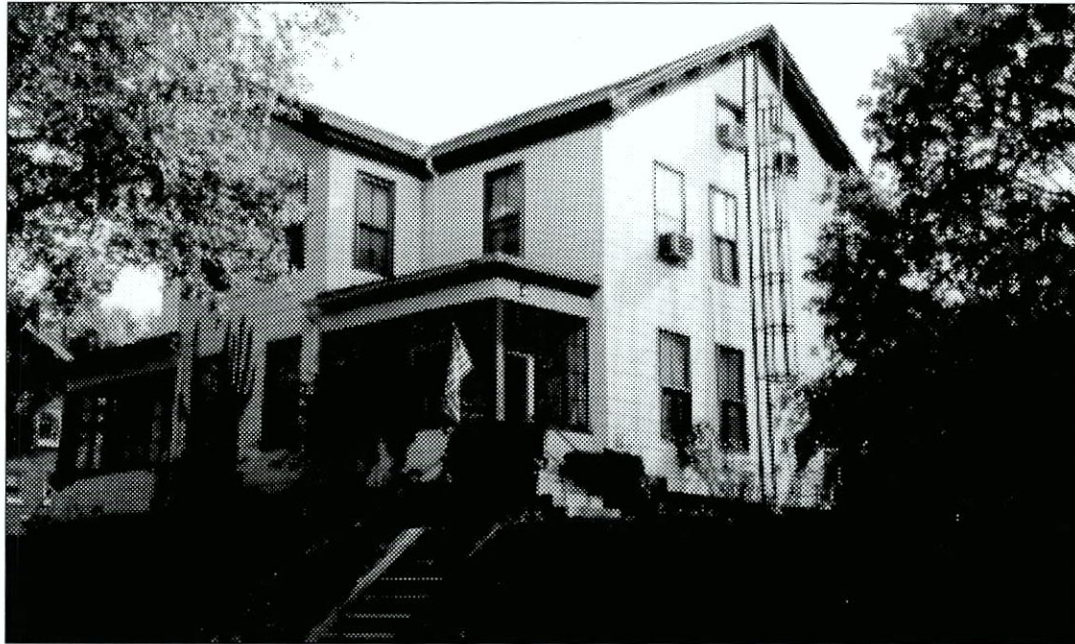
Figure 6.124 Building 114. By Cultural Resources Center, 1994.
