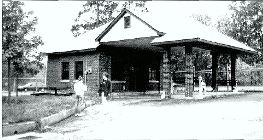
Figure 6.164 Building 303/304 showing the east and north facades. Recent vinyl siding in gables and asphalt shingle roof sheathing. Potential for buried fuel tanks.
