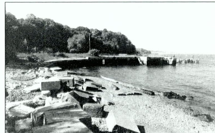
Figure 6.51 View of seawall near dock showing complete failure and collapse of the wall system.
