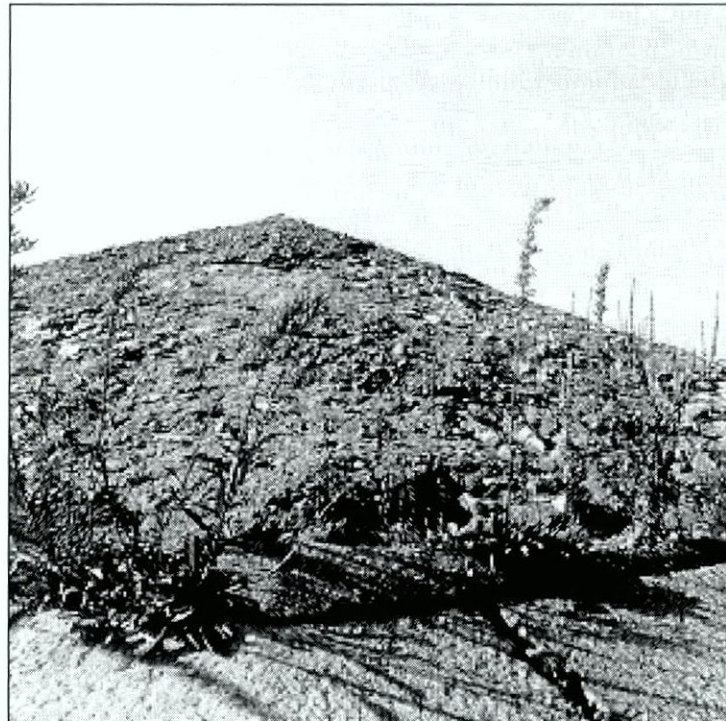
Figure 6.25 Detail showing general deterioration of cement caps at the stairtowers and the introduction of unwanted vegetation.
