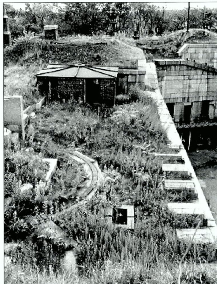
Figure 6.63 Fort Tompkins, barbette. Looking west.
