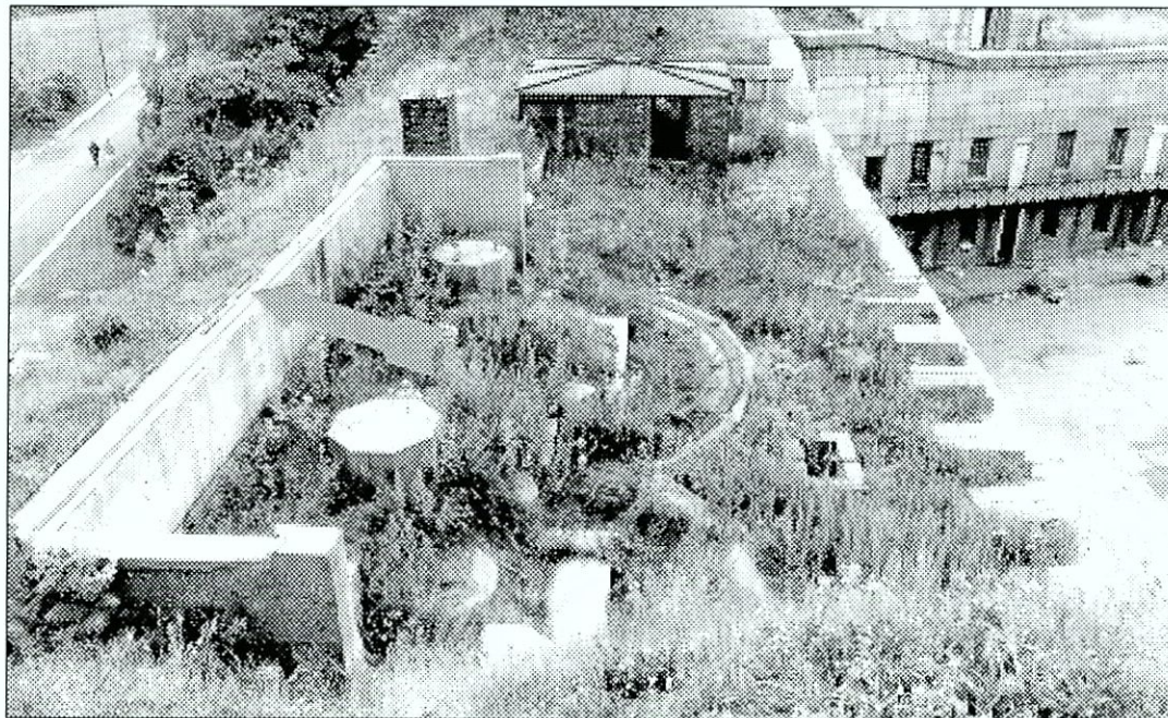
Figure 6.87 South barbette looking west. Gunmounts concealed by vegetation. Cracking of concrete throughout. Spalling of concrete (arrow) caused by ferrous corrosion of piperail.
