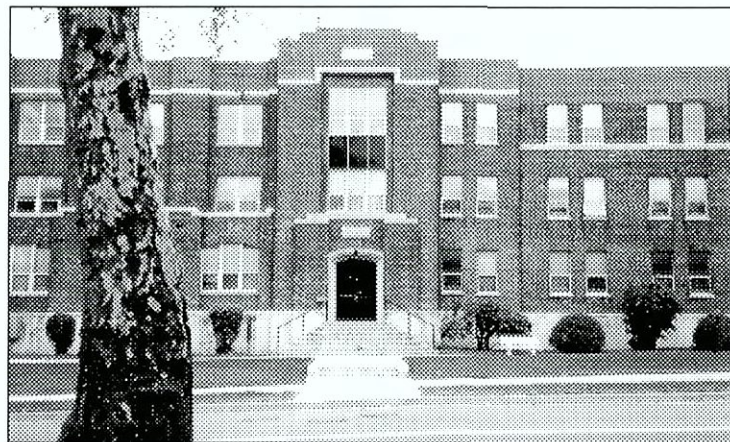
Figure 6.138 building 210, facade. By Cultural Resources Center, 1994.
