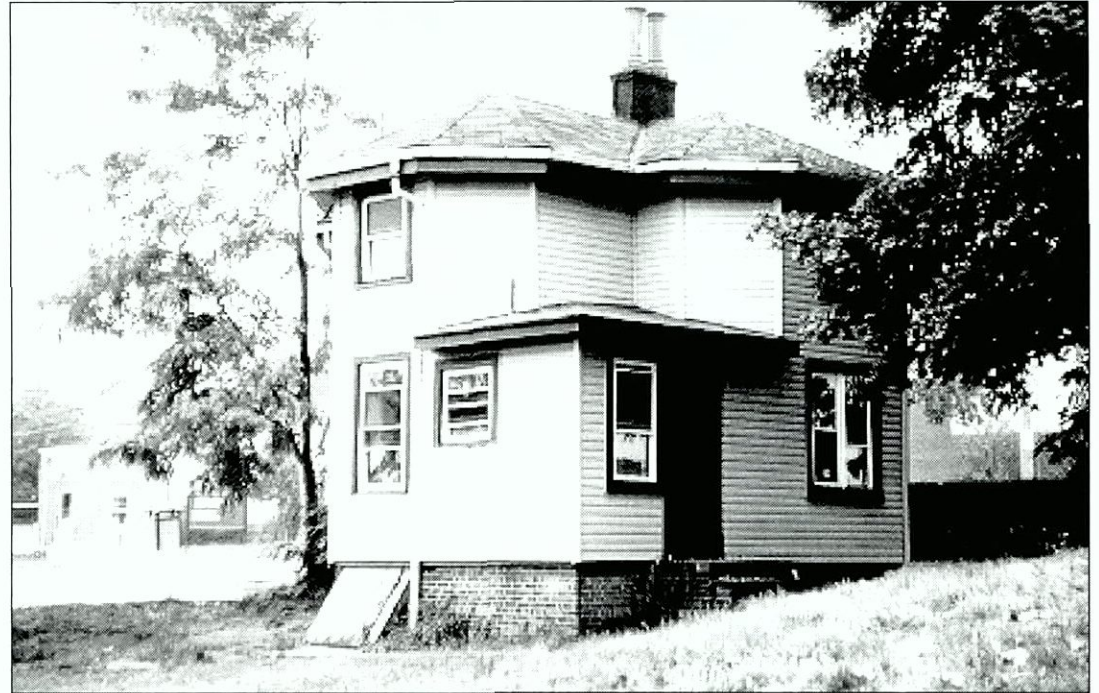
Figure 6.169 General view of building 406 (former residence) showing south and west facades. Note recent application of vinyl siding and replacement of window units.
