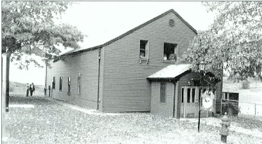
Figure 6.156 General view of Building 352 showing south and west facades. Recent addition of central-entry wing and replacement of all window units, new vinyl siding and asphalt shingle roofing.
