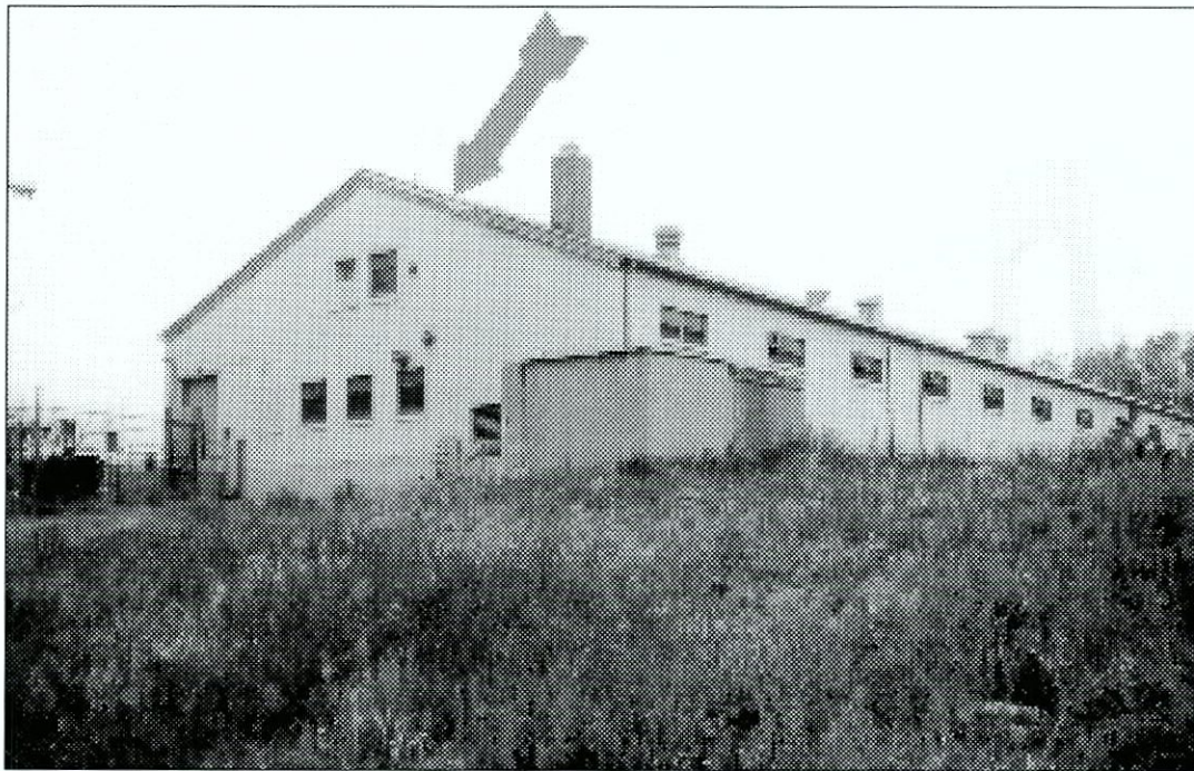
Figure 6.158 General view of Building 306 showing west and south facades. Arrow identifies failure of the vinyl sheathing at the raking eave.
