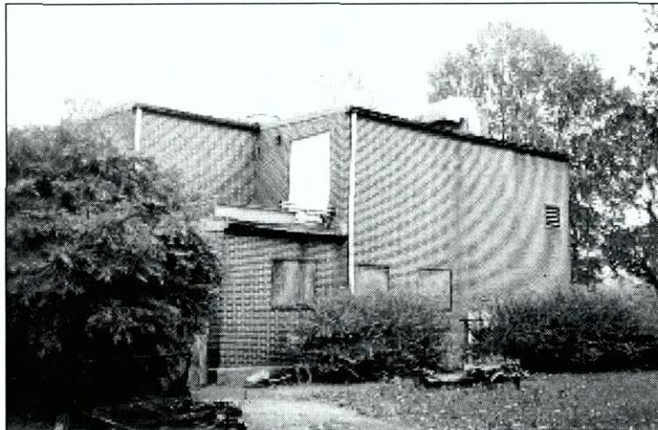
Figure 6.179 West (rear) elevation of the Theater showing boarded windows, staining on brick caused by faulty gutter.
