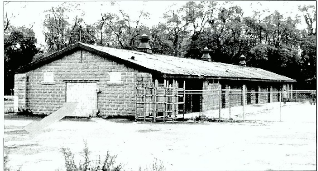
Figure 6.167 Building 309 showing north and west facades. K Arrow identifies in-fill of original garage opening with smooth-face concrete masonry units.
