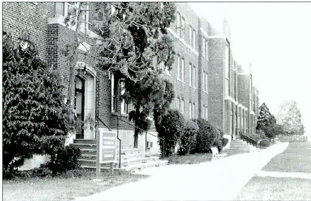
Figure 6.140 Building 210, facade, looking north. By Cultural Resources Center, 1994.
