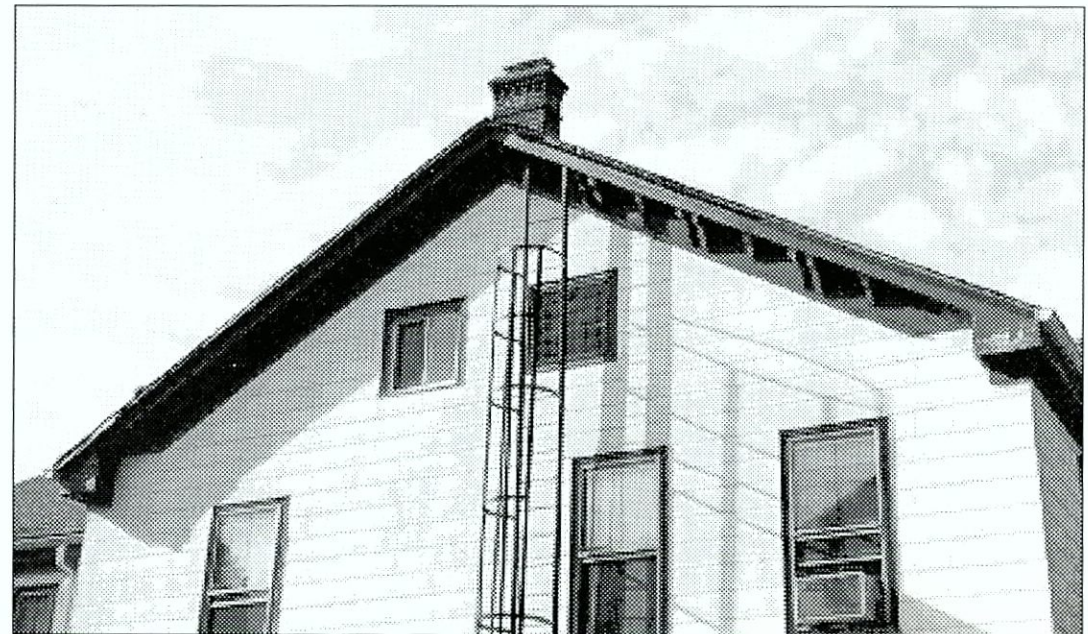
Figure 6.125 Typical rakeboard and chimney, Buildings 111-114. By Cultural Resources Center, 1994.
