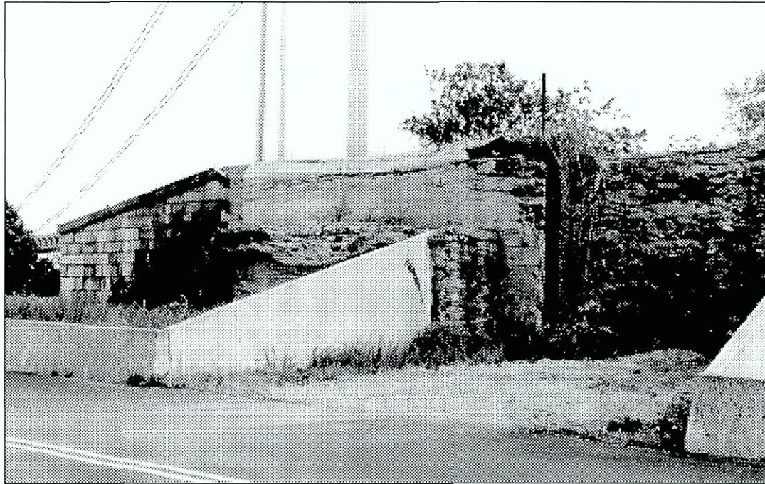
Figure 6.102 Battery Duane, north face at east corner. By Cultural Resources Center, 1994.
