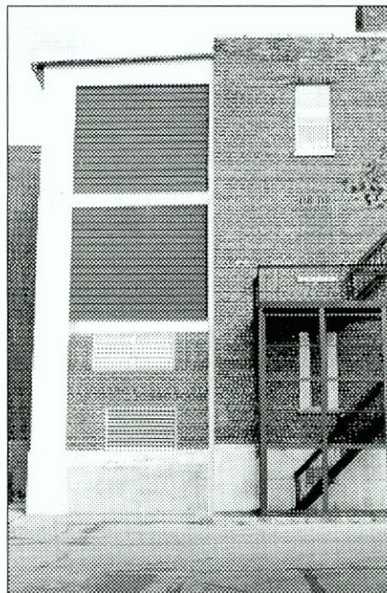
Figure 6.139 Building 210, rear addition. By Cultural Resources Center, 1994.
