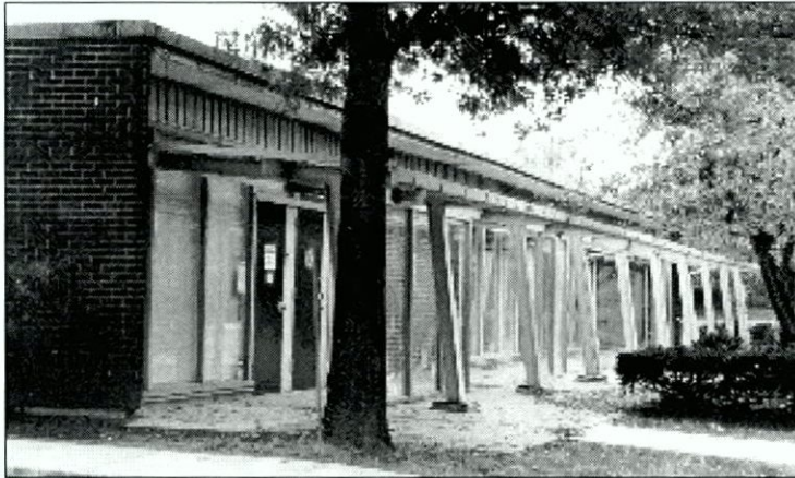
Figure 6.181 View of the north (main) facade of PX Building 206.6.182 View through covered walkway looking east. Awning originally had a roof to shed water away from the sidewalk and protect shoppers from rain.
