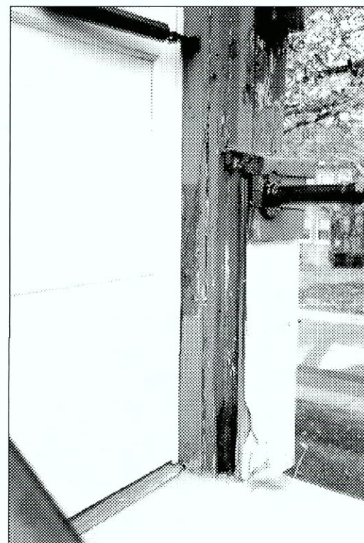
Figure 6.134 Detail of typical door at porch. Failed paint finish and deteriorating wood trim. Breakage of composite shingle is typical throughout duplex units. Note: newer aluminum porch doors alter original integrity.
