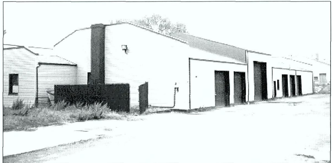
Figure 6.165 Building 302 showing east and north facades. K Note recent alteration of central bay to receive large trucks. Vinyl siding has covered original industrial windows.
