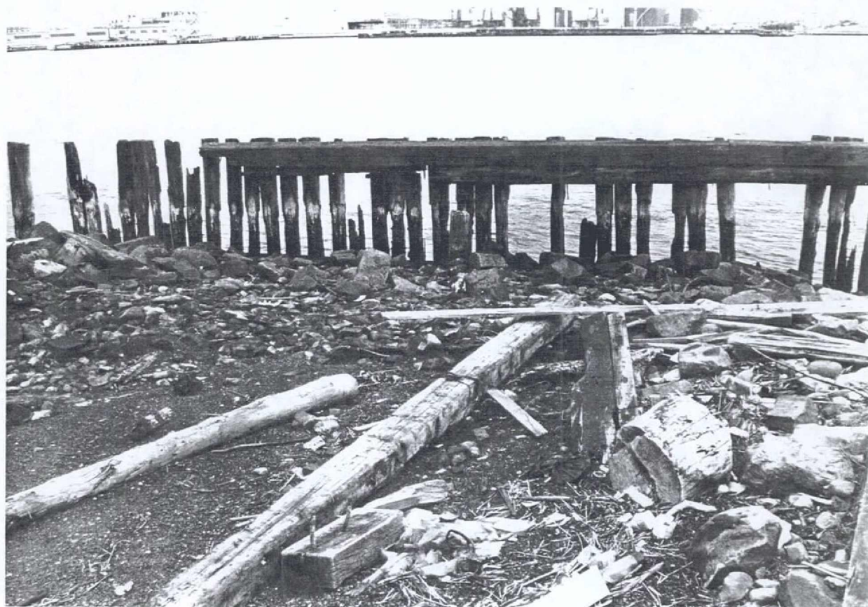
Figure 5:1 Present condition of seawall, stone rip-rap, and wooden bulkheads. (Photo: Carl Forster, 1986).
