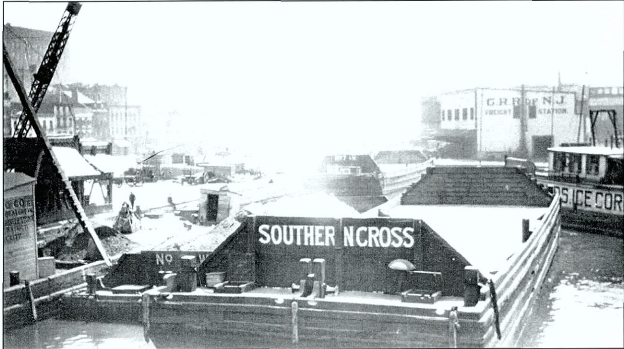
Figure 5. View of three rock scows in a turn-of-the-century photograph. Note the rock scow on the left being loaded with sand and rock by the crane barge. Also note how low in the water it sits compared to the two unloaded rock scows (courtesy of the South Street Seaport Museum).
