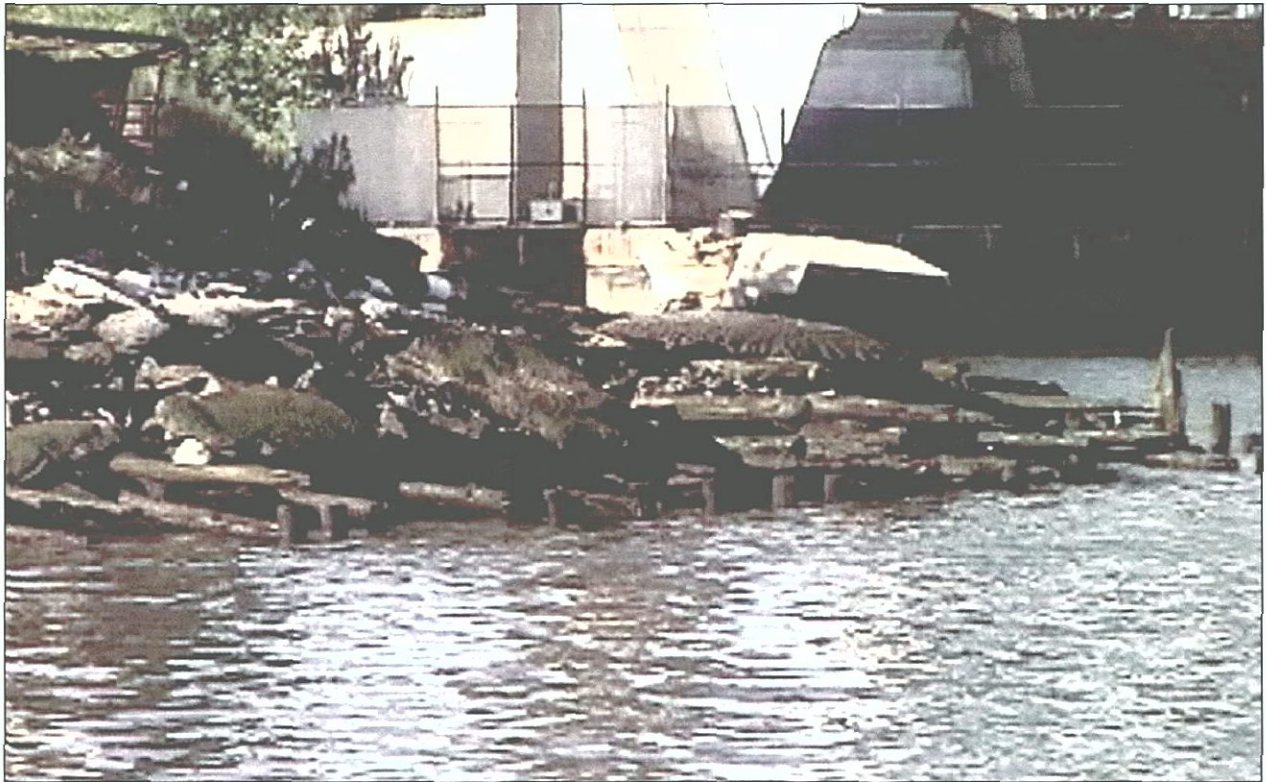
Figure 109. Photograph of Structure S107.
