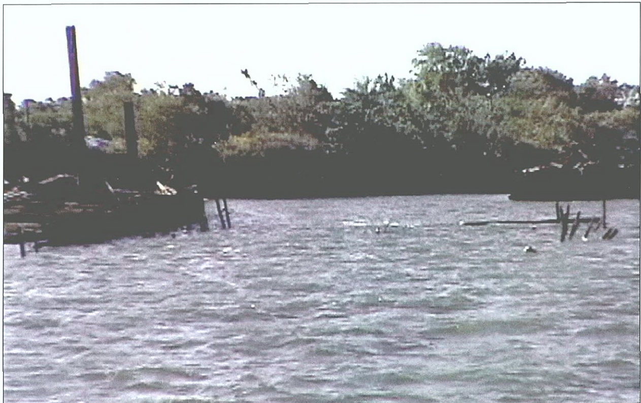
Figure 115. Photograph of V38 – floating drydock (mostly submerged).
