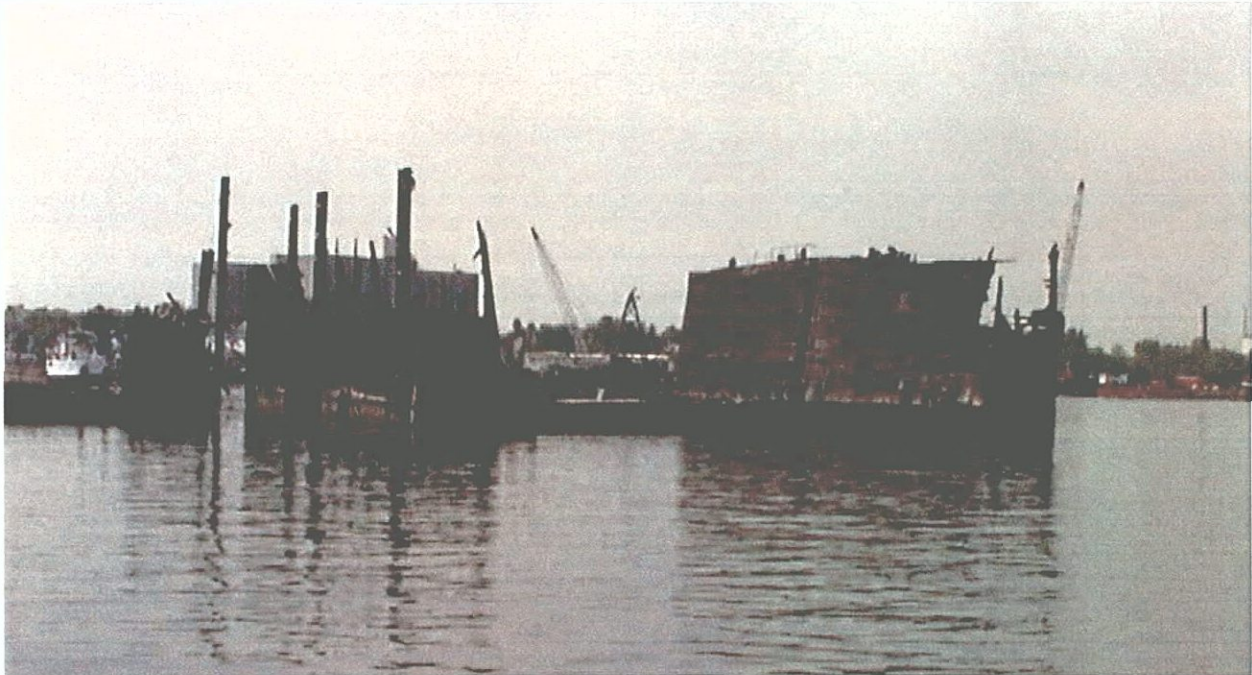
Figure 96. Photograph of Vessel V2 (foreground).
