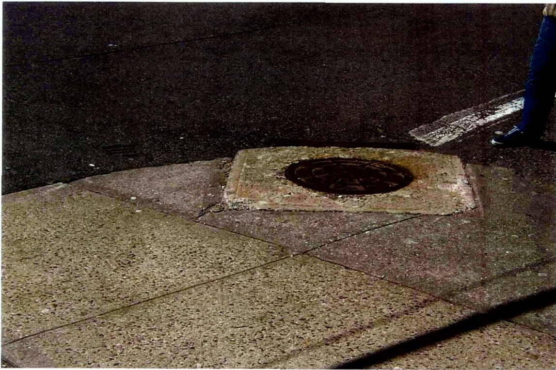
Photograph 22-1: Northeastern corner of West Fordham Road and Sedgwick Avenue, Shaft Site 22.
