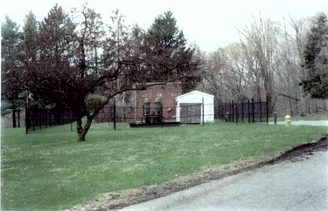
Photograph 6-1: Looking northwest, Shaft Site 6.
