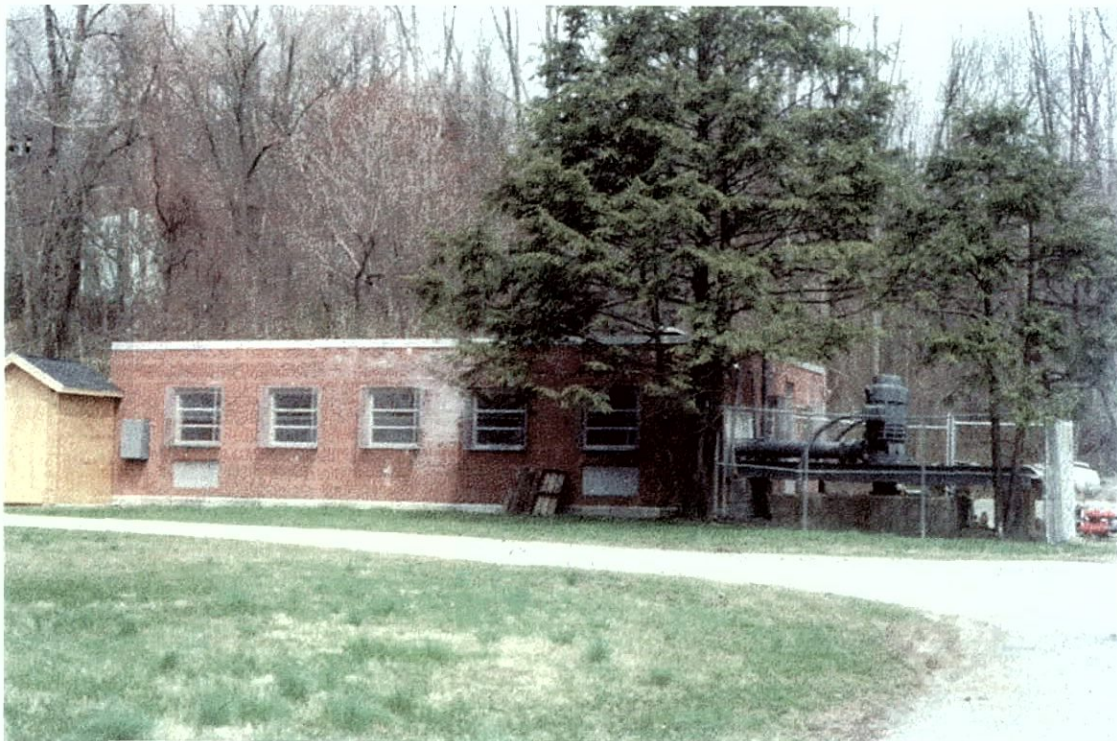
Photograph 4-2: Looking west, Shaft Site 4.
