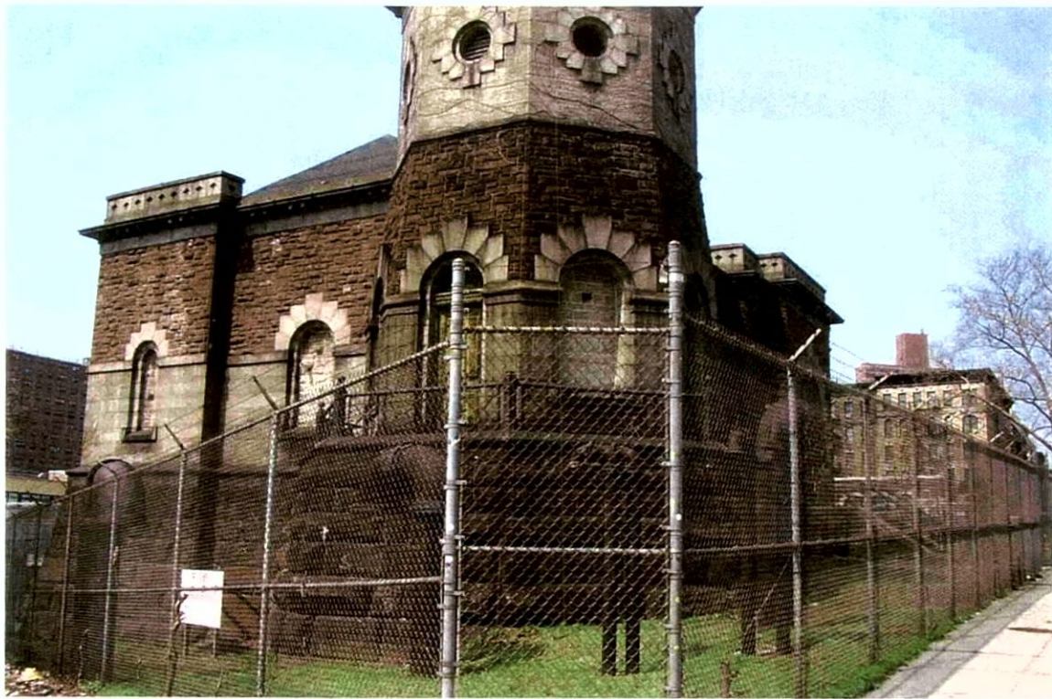
Photograph 33-1: Looking southwest, from southwest corner of Convent Avenue and 135 th Street, 135 th Street Gatehouse and Shaft Site 33.
