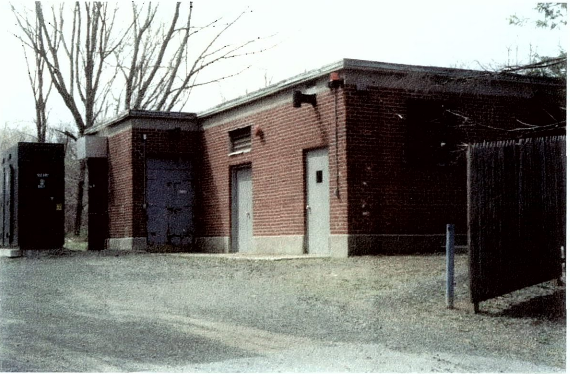
Photograph 3-2: Looking southwest, Shaft Site 3.
