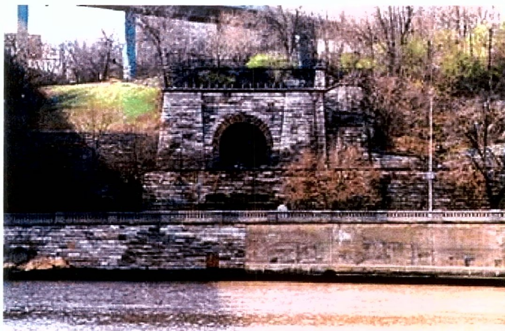
Photograph 25-1: Shaft No. 25. Facing west from the Harlem River. Source: Kornfeld 1998.
