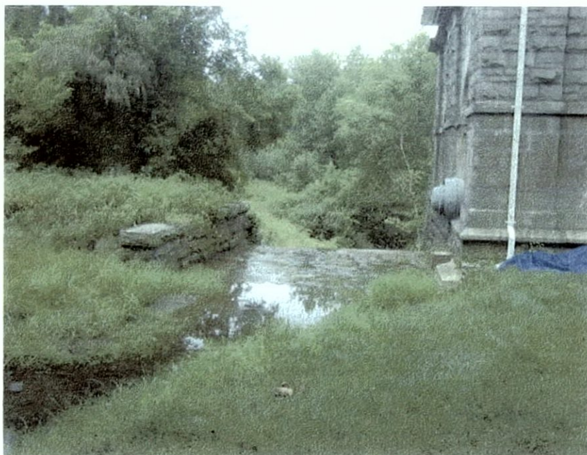
Photograph 9-2: Looking west, Shaft Site 9.
