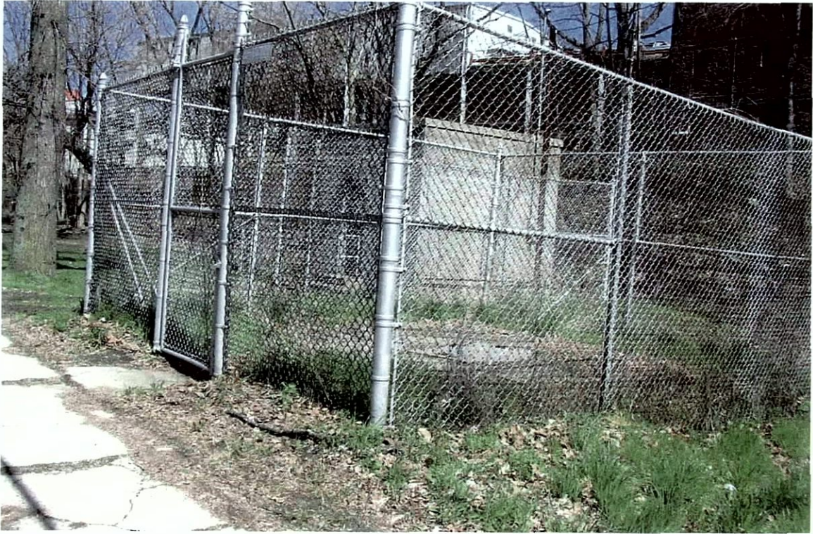
Photograph 18 1/4-1: Looking northeast, from Midland Avenue and the eastern edge of Tibbetts Brook Park, Shaft Site 18 1/4.
