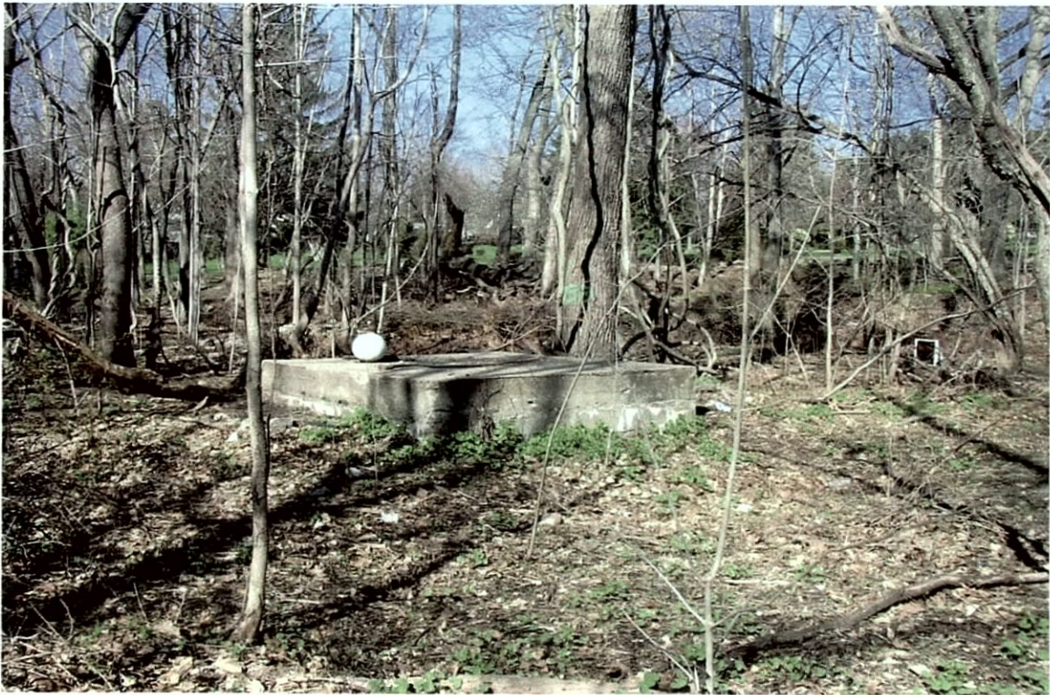
Photograph 13-2: Looking west, Shaft Site 13.
