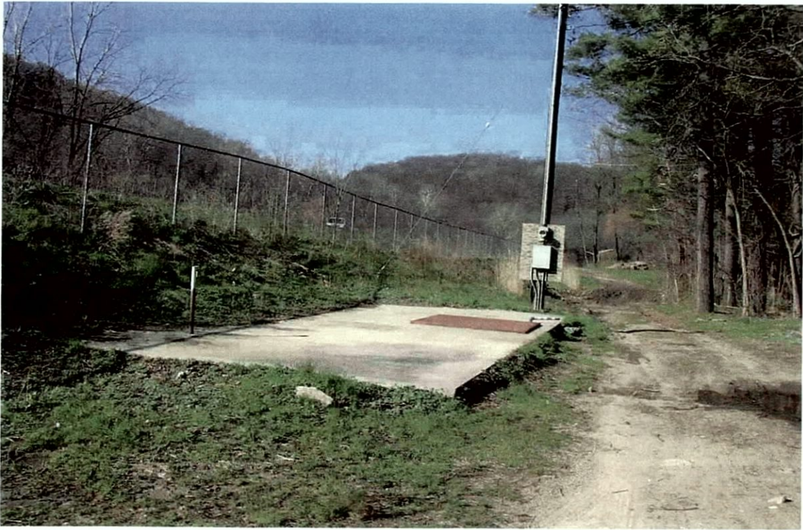
Photograph 12A-1: Looking northwest from Saw Mill River Road, Shaft Site 12A.
