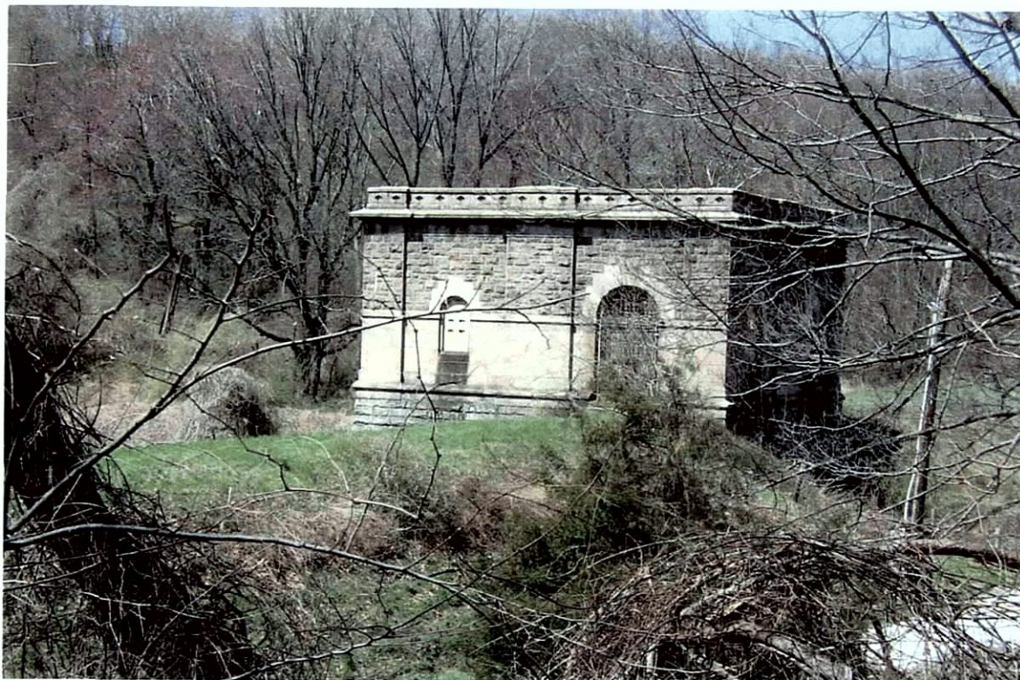
Photograph 18-1: Looking northwest from Rumsey Avenue, Shaft Site 18.
