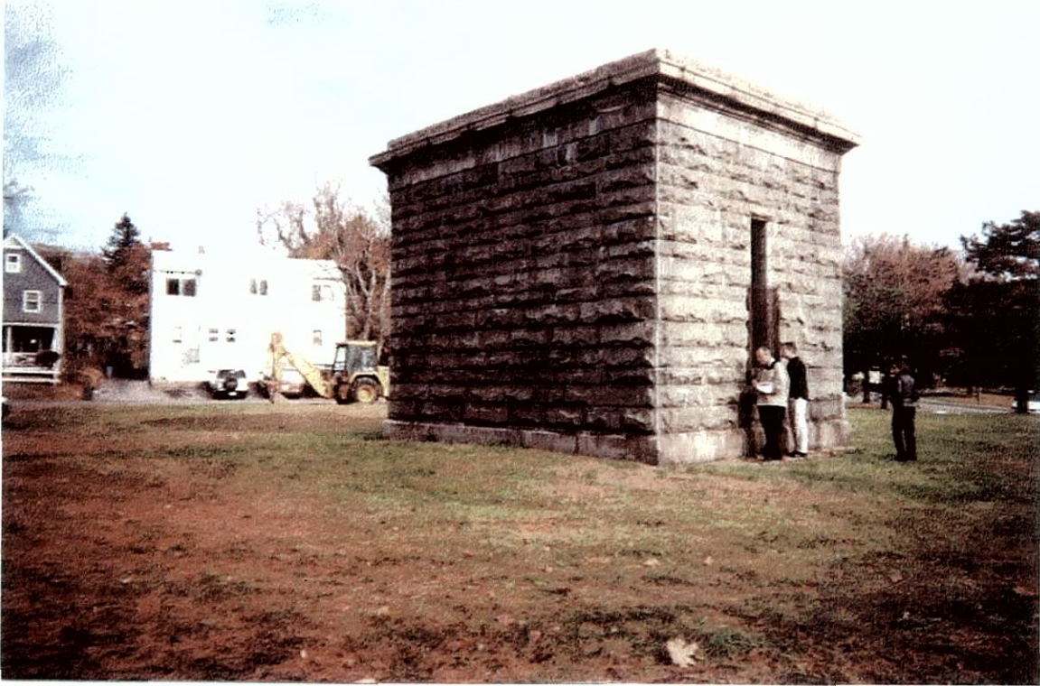
Photograph 11A-1: Looking northeast, Shaft Site 11A.
