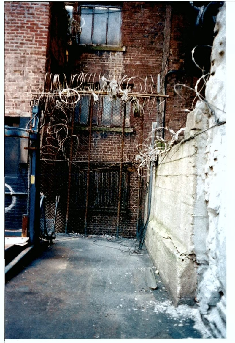
Facing south toward rear of lot. Foto III F-2
