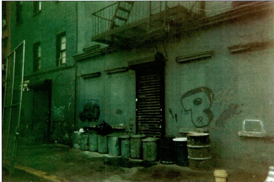
Facing southeast from West 38 th Street to building on Block 735, Lots 59 & 60 Photo IV A 10-1
