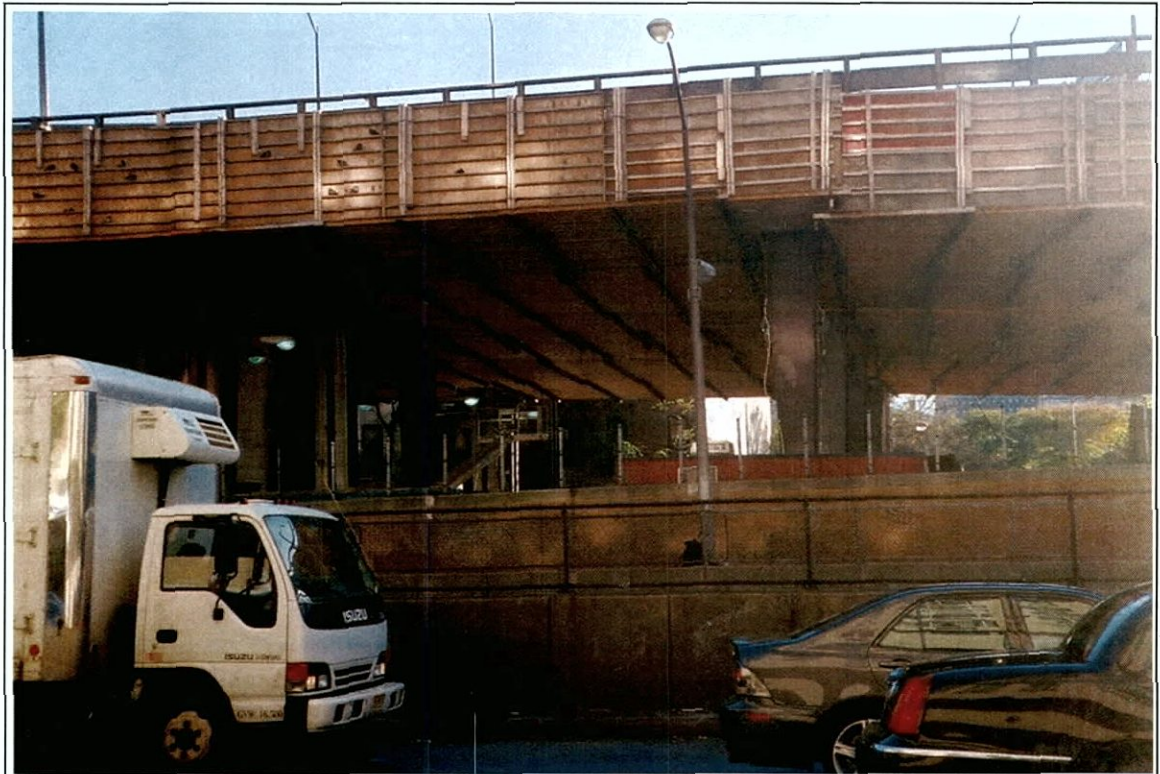
Facing east on West 41 st Street. Foto III F-4
