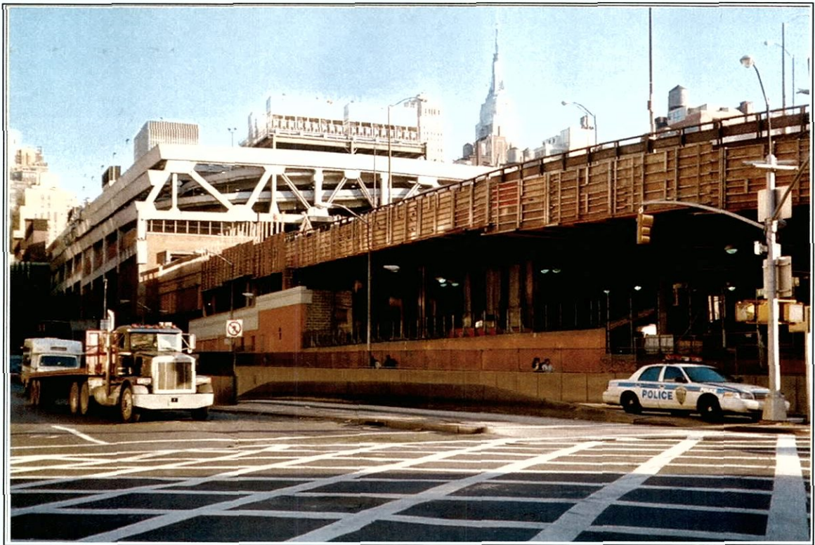
Facing east on West 41 st Street. Foto III F-3
