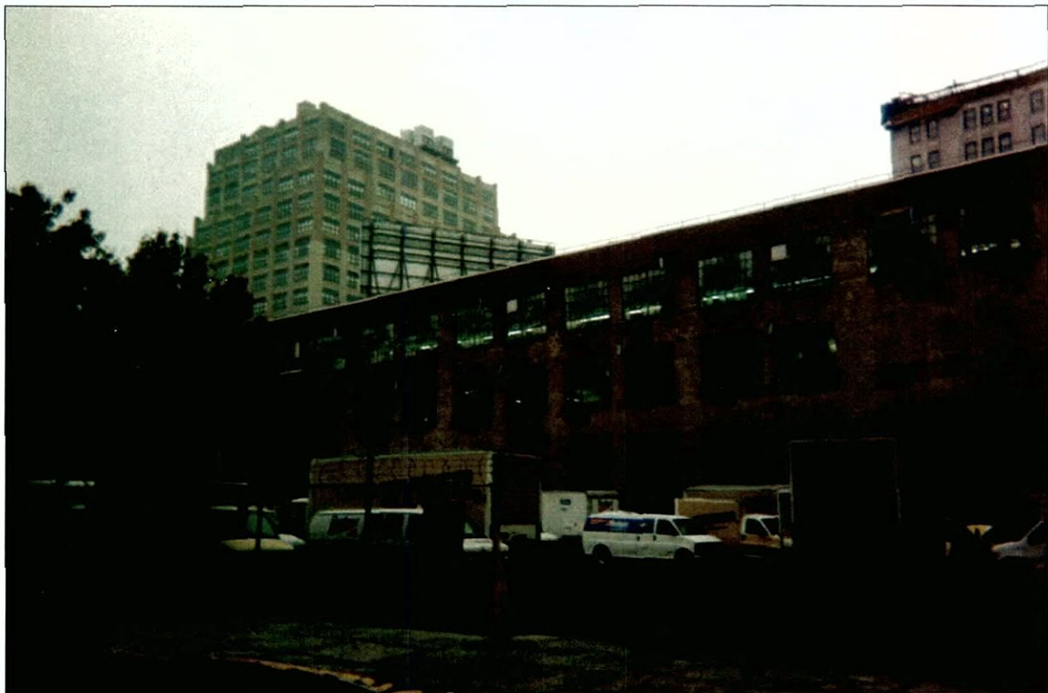
Block 706, Lot 29, facing southeast. Foto IV A 1-2
