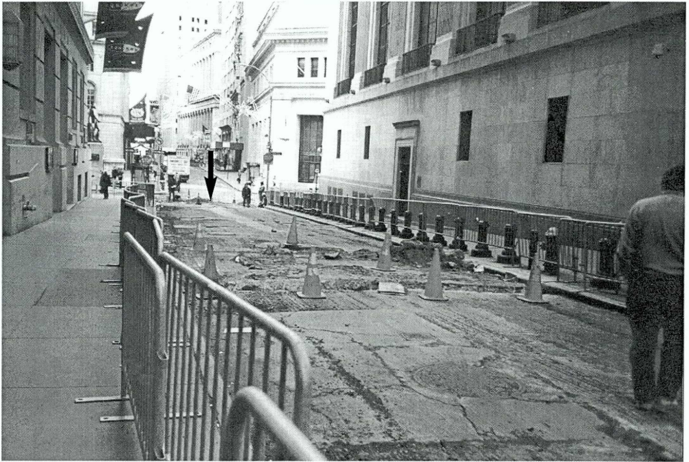
40 View east on Wall Street between New Street and Broad Street. Test Pit 7 (TP7) is in the foreground. Test Pit 8 (TP8) in the background (arrow) is near the Broad Street intersection. (Spritzer 11/15/03)
