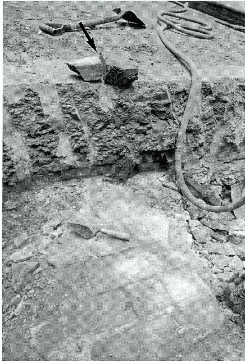
38 Remnant of 9-inch thick concrete base for asphalt block paving revealed in Test Pit 3 (TP3) on Exchange Place east of Broadway. Fragments of the asphalt block (arrow) and whole blocks, that measured 3 by 5 by 12 inches, were also noted. This road surface, which was 1.5 feet below current grade, was introduced in 1931 or 1932 (see text and Figure 39). (Geismar 9/27/03)
