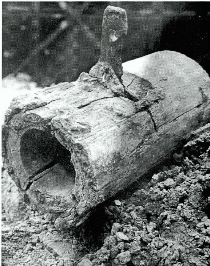
14 Section of log water main with stop cock in place. (Courtesy of Chase Archives)
