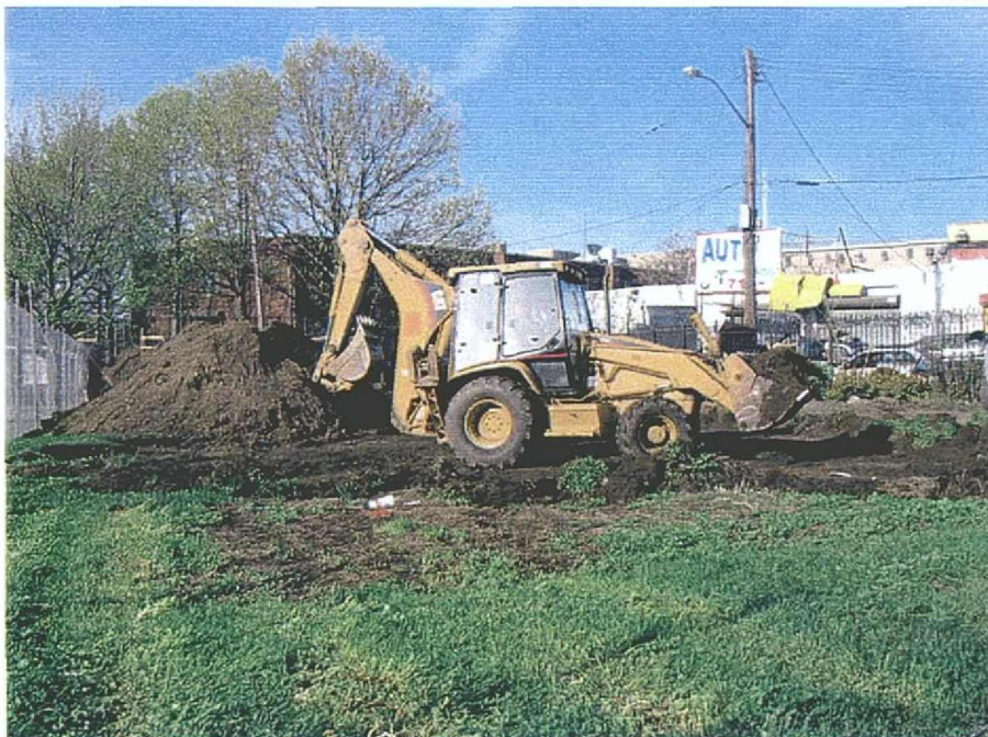
Figure 17: Excavation in northern (front yard) of house
