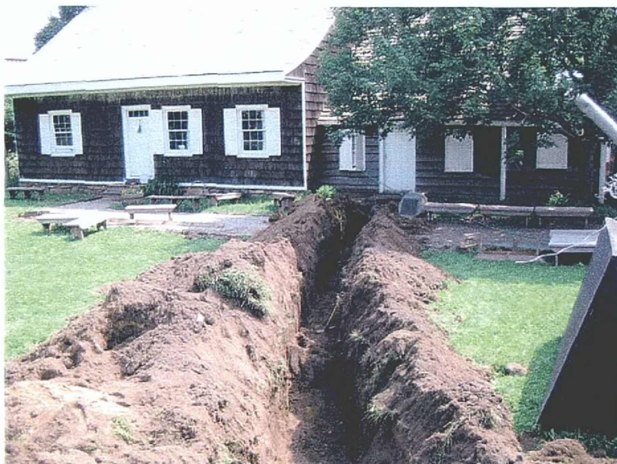
Figure 12: water-utility line connection into the house
