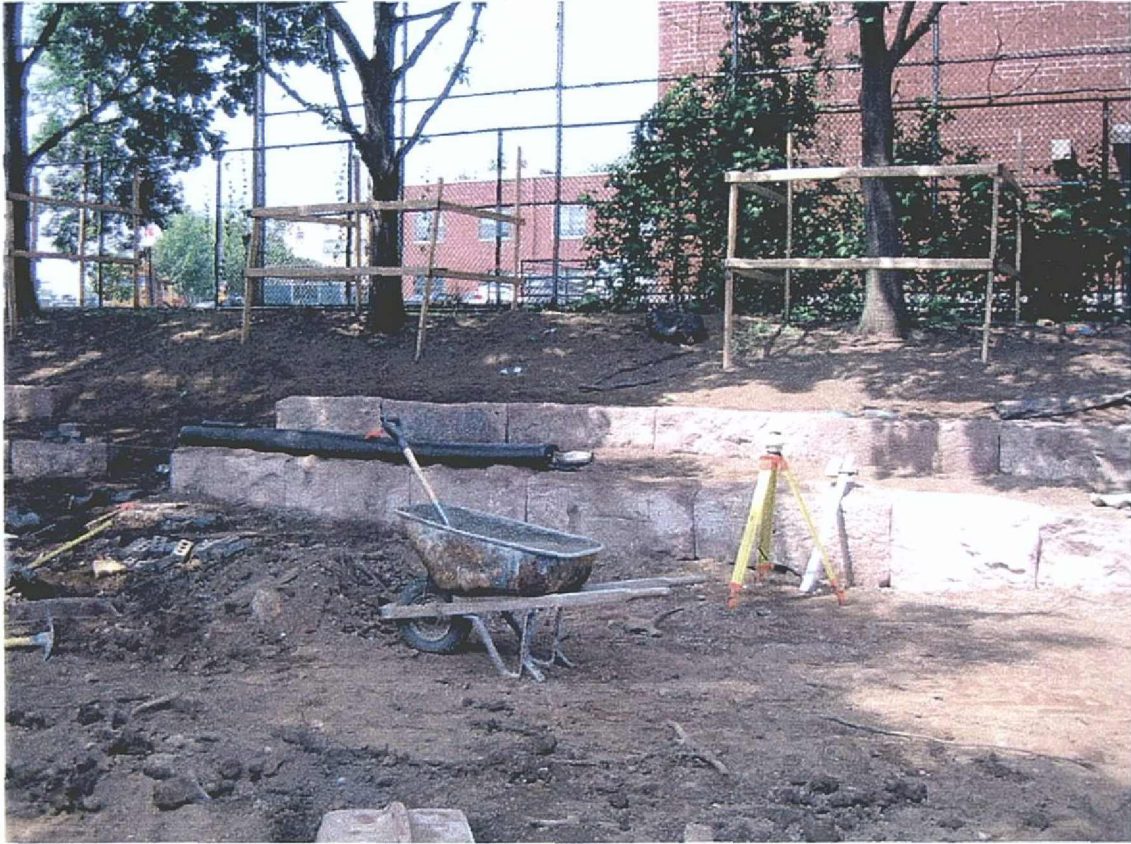
Figure 8: stone seating area-retaining wall
