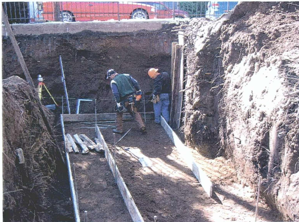
Figure 5: Stairway foundation
