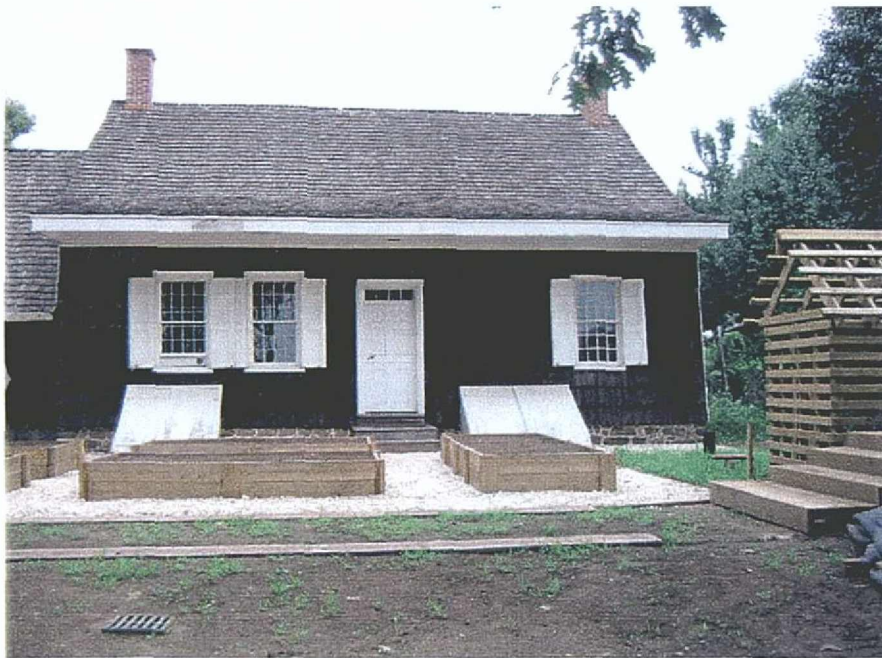
Figure 7: Completed flower bed area
