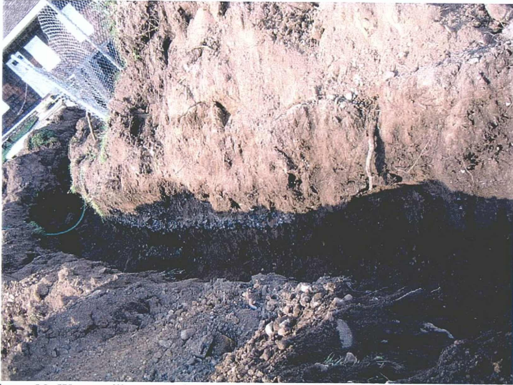
Figure 20: Water-utility trench in the northern field showing remains of Canarsie Lane
