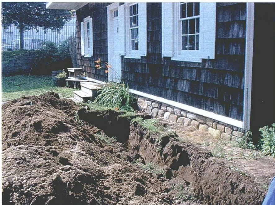
Figure 15: Extended trench for water-utility line in northern field
