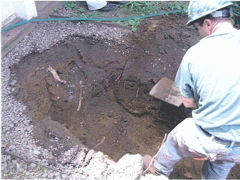
Figure 16: hand excavation of water-utility line adjacent to house
