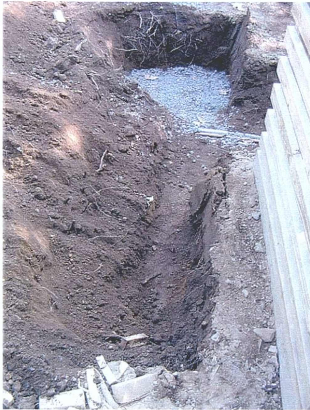
Figure 6: HVAC connection area
