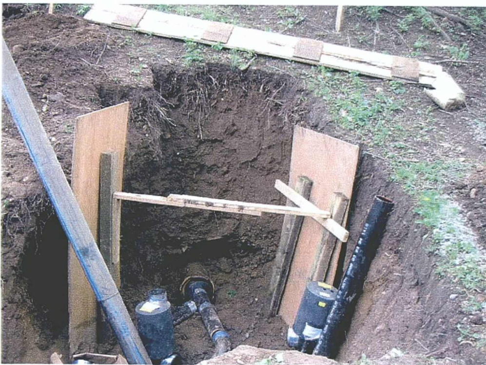
Figure 21: Sewer connection – southern field
