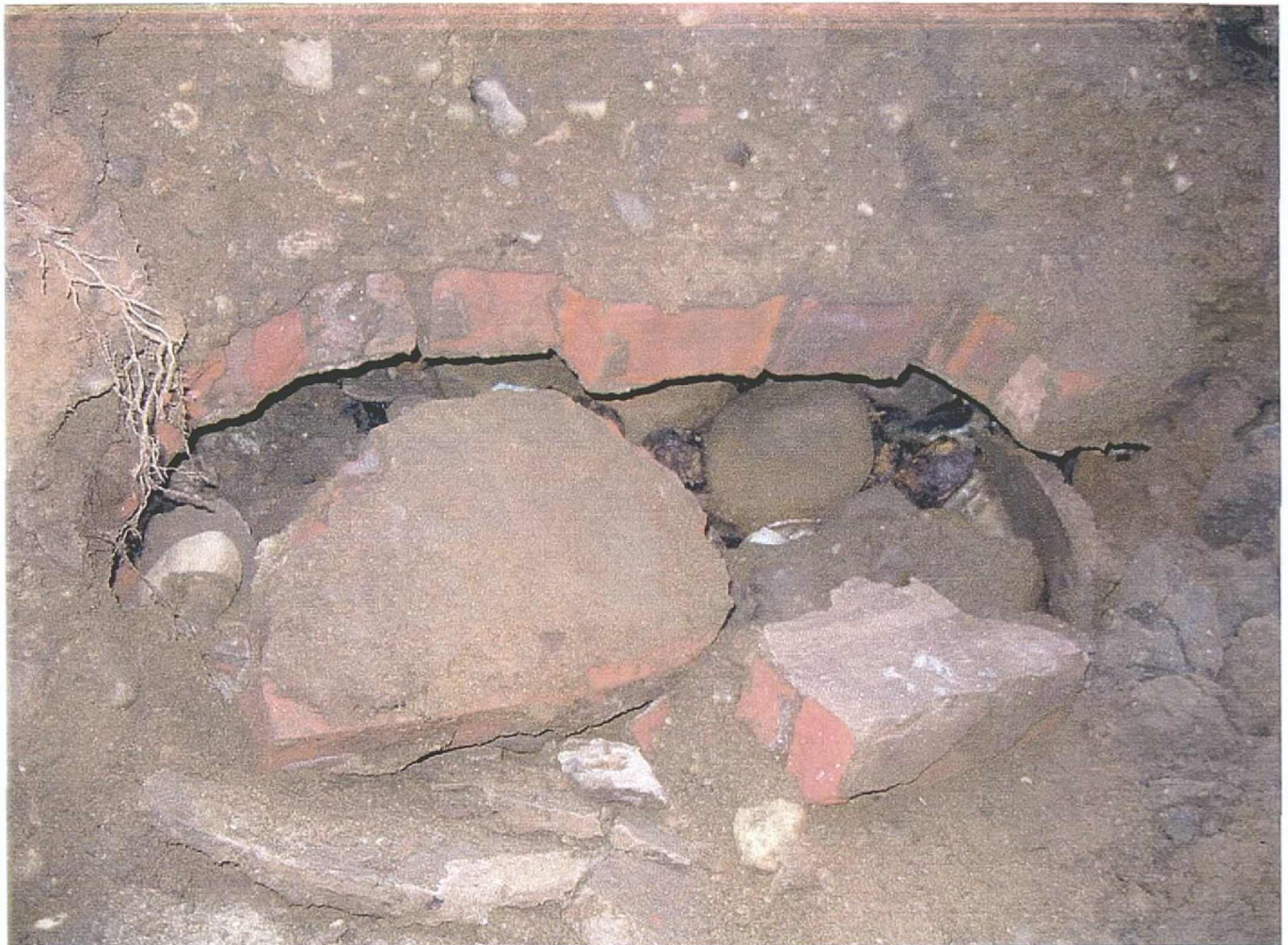
Figure 12: Top and side portion of cistern cut into with back-hoe
