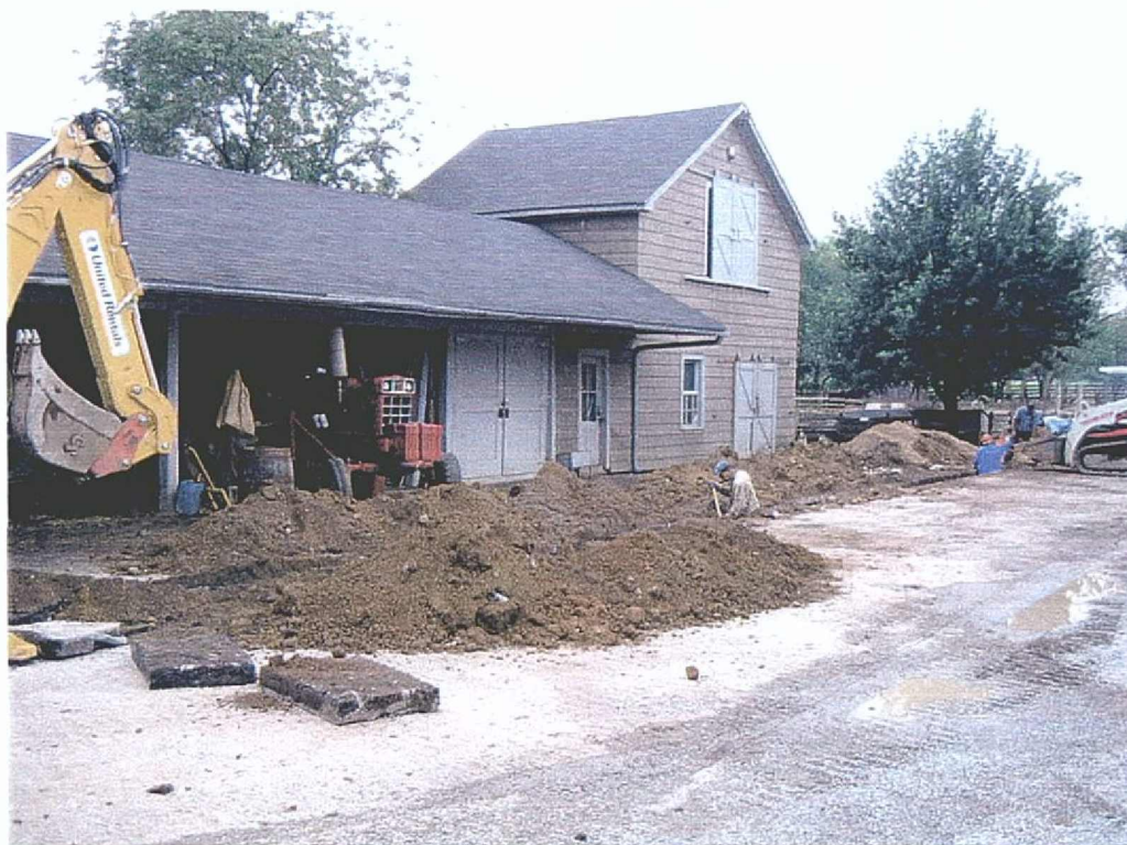
Figure 22: Excavation for new Utility Lines in roadway
