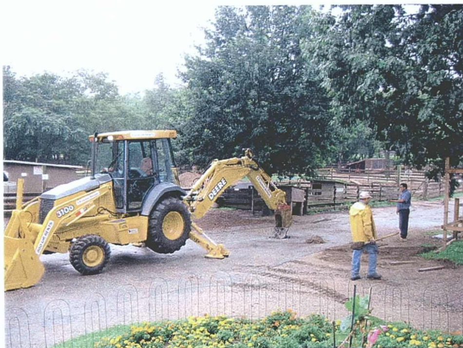
Figure 03: Excavation the Utility Line
