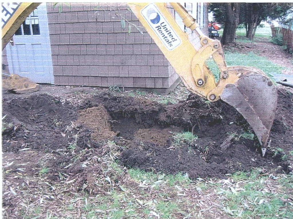
Figure 20: Excavation for Drinking Fountain, Dry Well and Wash Basin area
