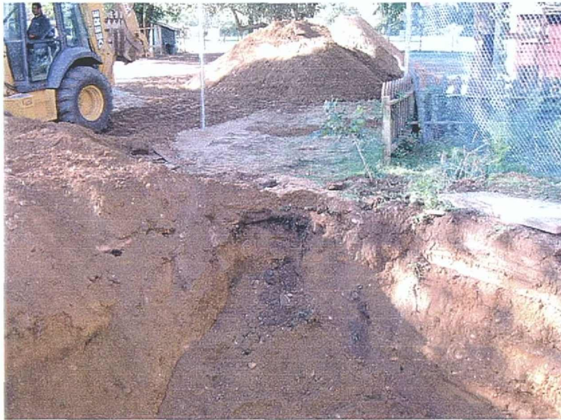
Figure 26: Trench connecting underground water storage tank with Windmill area
