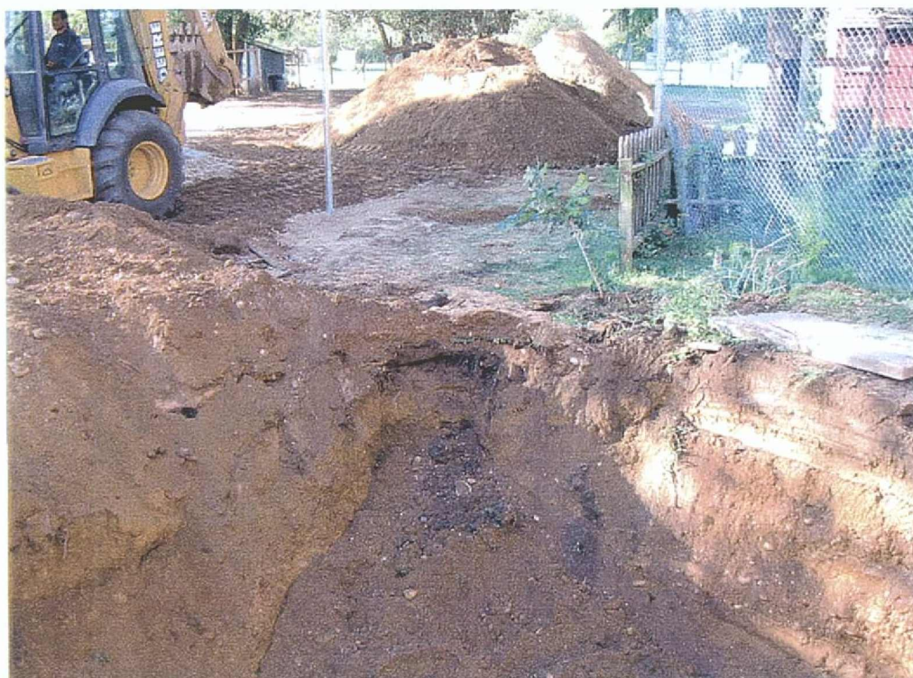
Figure 16: Clean fill in the stratigraphic layers of the large underground water storage tank area.
