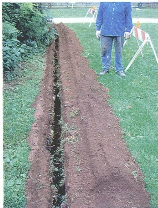
Figure 09: Utility Line trench completed
