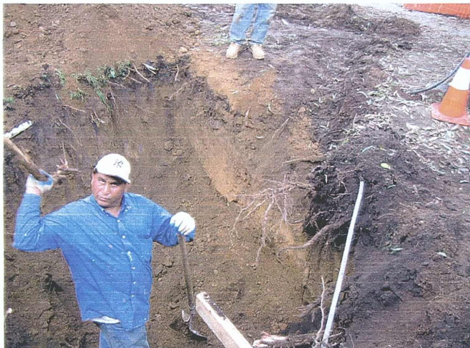
Figure 21: Clean fill in trench for Drinking Fountain, Dry Well and Wash Basin
