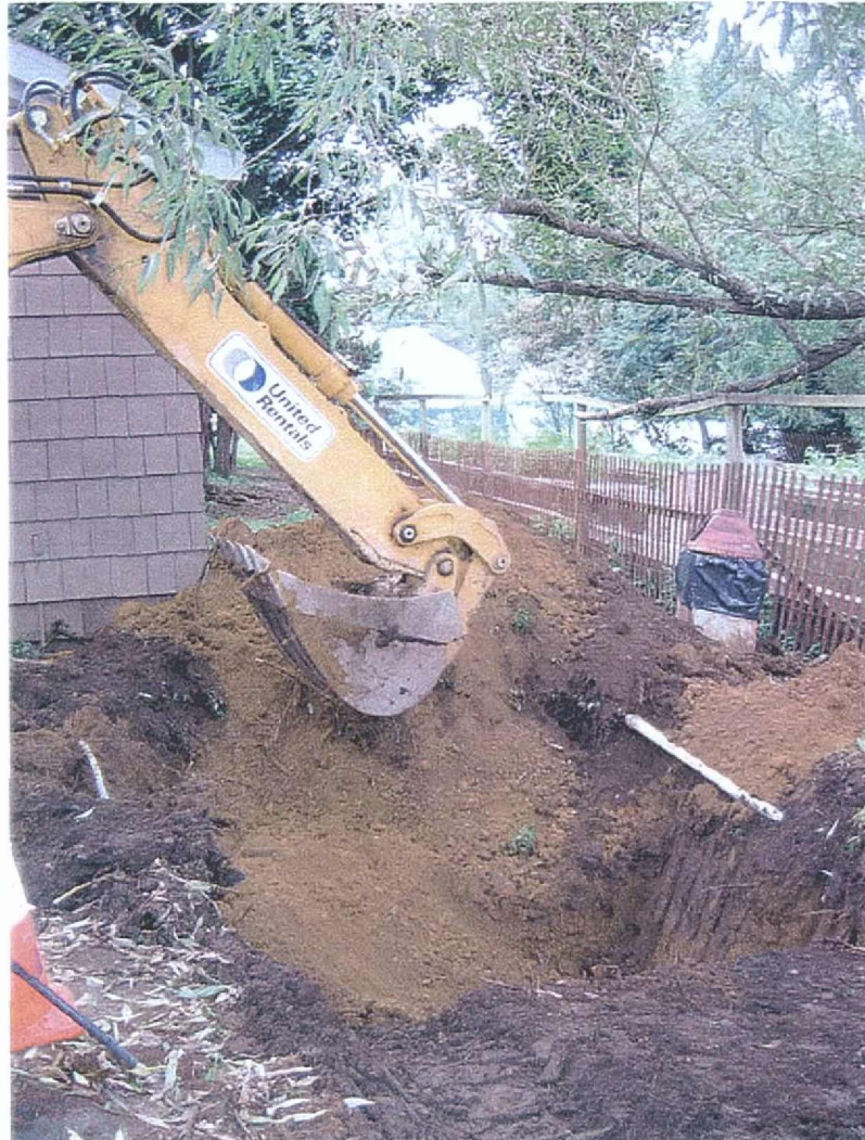
Figure 06: Clean fill in the water fountain, dry well and wash basin area
