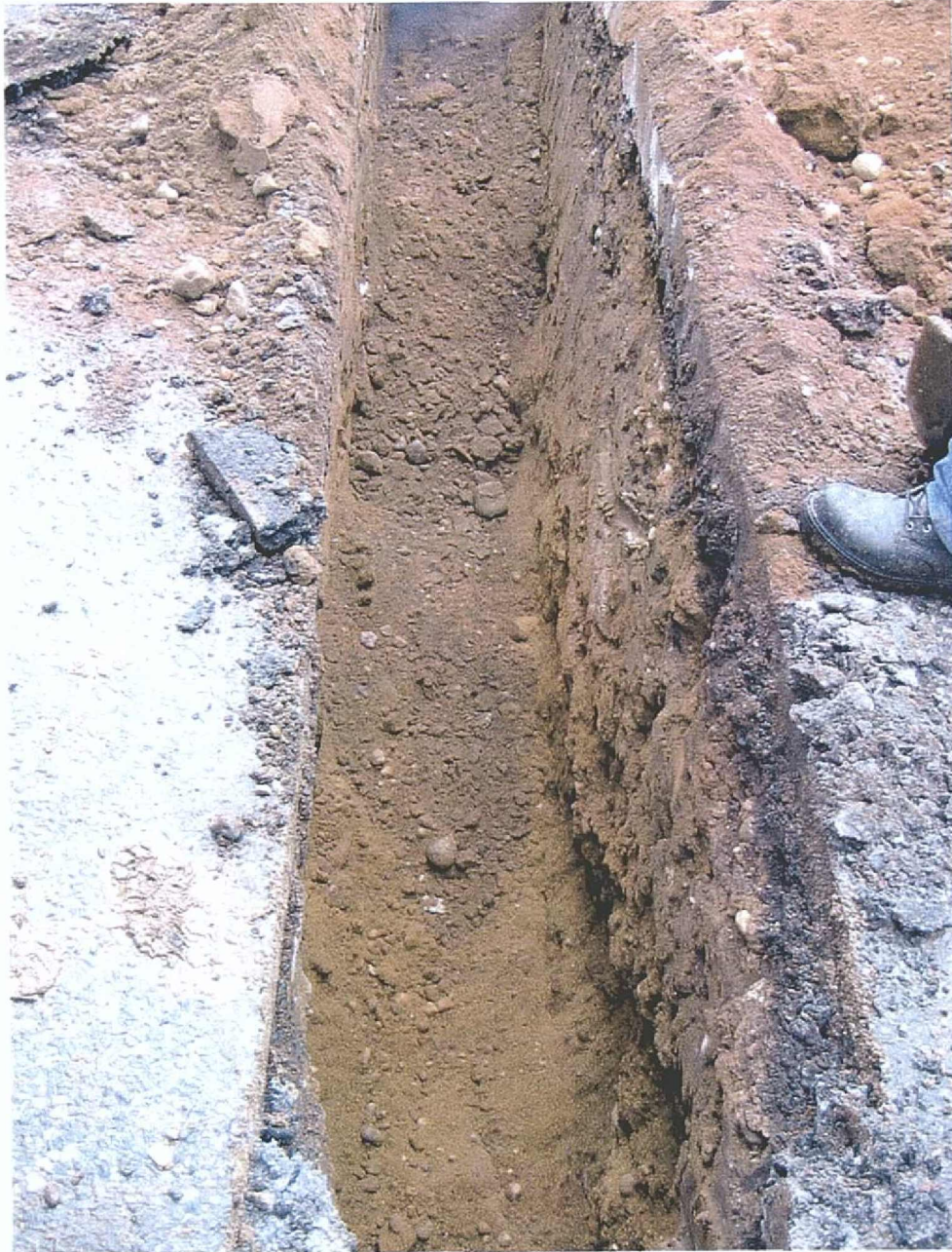
Figure 04: Clean fill in comprised the majority of the Utility Line area
