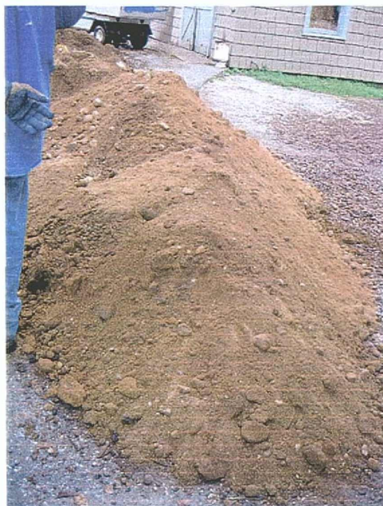
Figure 23: Clean fill from excavated Utility Line in the roadway
