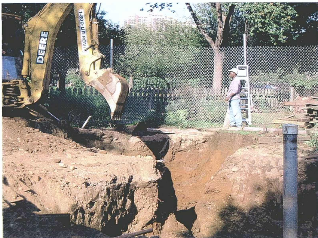
Figure 15: Excavation for large underground water storage tank
