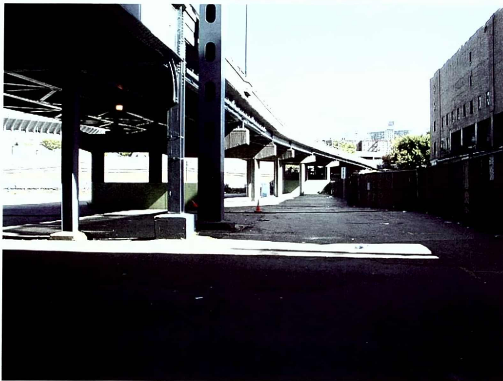
Photograph 10: Ramp for the Major Deegan Expressway north of Building A. View looking east with Yankee Stadium on the left.
