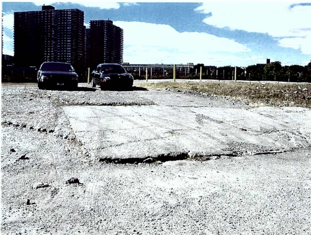
Photograph 18: Surface of Pier 3, showing uneven surface and former concrete foundation. View looking west.
