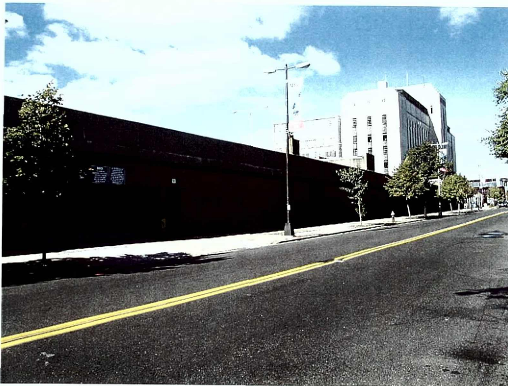
Photograph 6: Building C (on left) and the Bronx House of Detention (on right). View looking north with River Avenue in the foreground.
