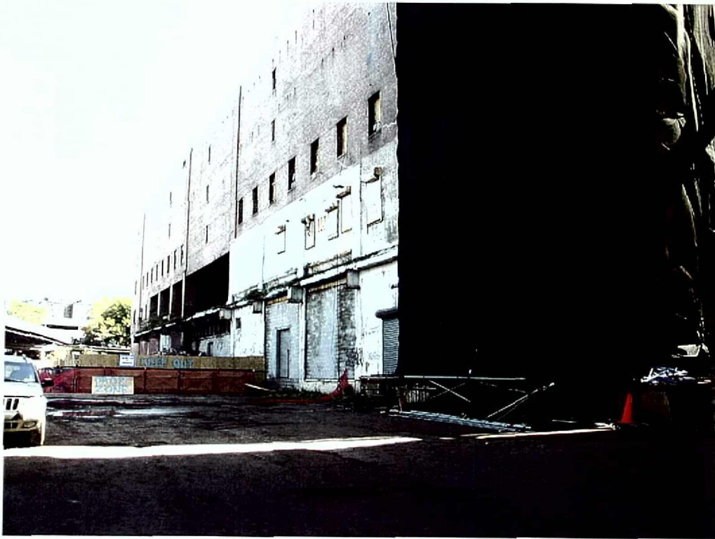
Photograph 1: Building A, in the process of being demolished. View looking southeast.
