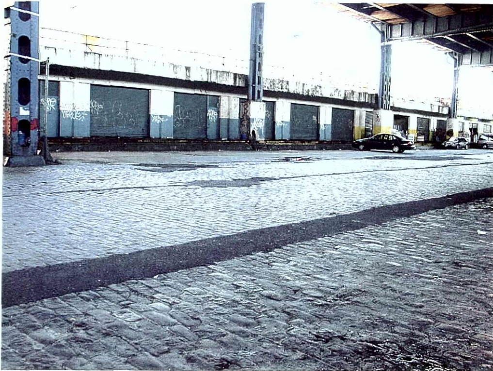
Photograph 2: Building B. View looking southeast with Exterior Street in the foreground and the Major Deegan Expressway overhead.
