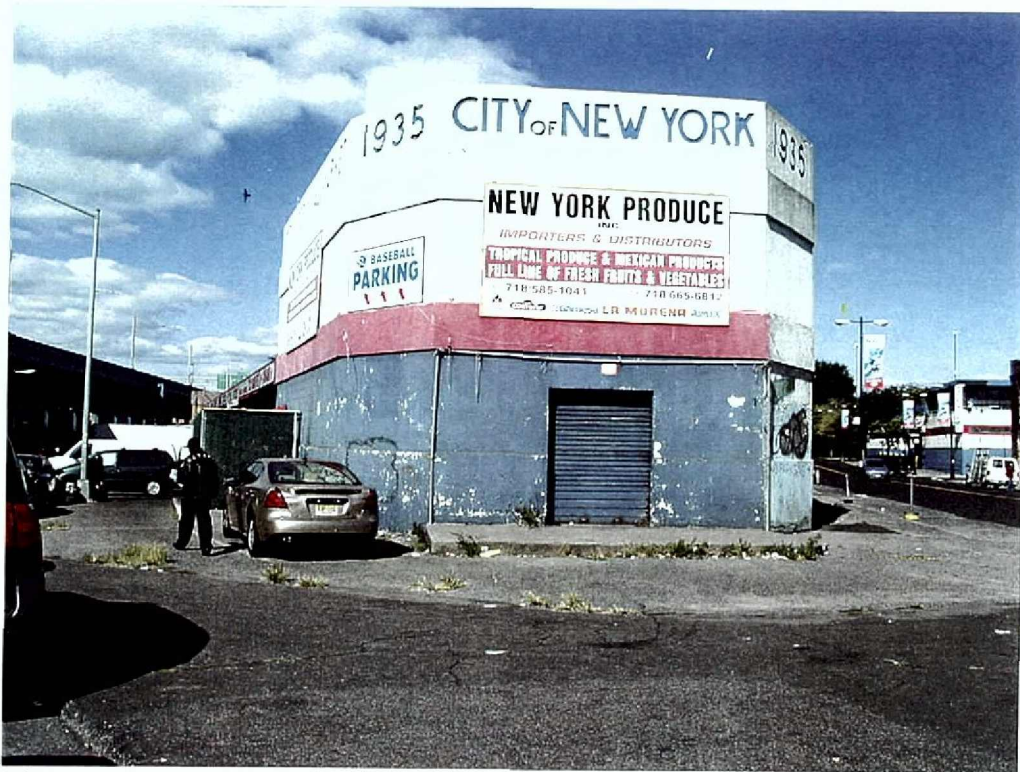
Photograph 5: Building D. View looking northeast with River Avenue on the right and Exterior Street and the Major Deegan Expressway (overhead) on the left.
