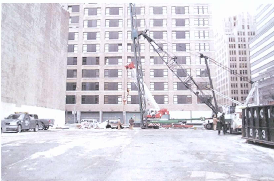
Plate 6. The proposed location of Shaft 28B; view to the south.
