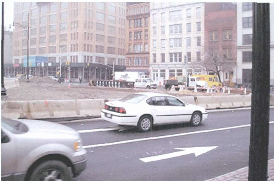
Plate 7. The proposed location of Shaft 29B (Block 213); view to the southwest.
