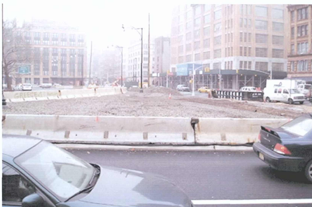
Plate 8. The proposed location of Shaft 29B (Block 213); view to the south.
