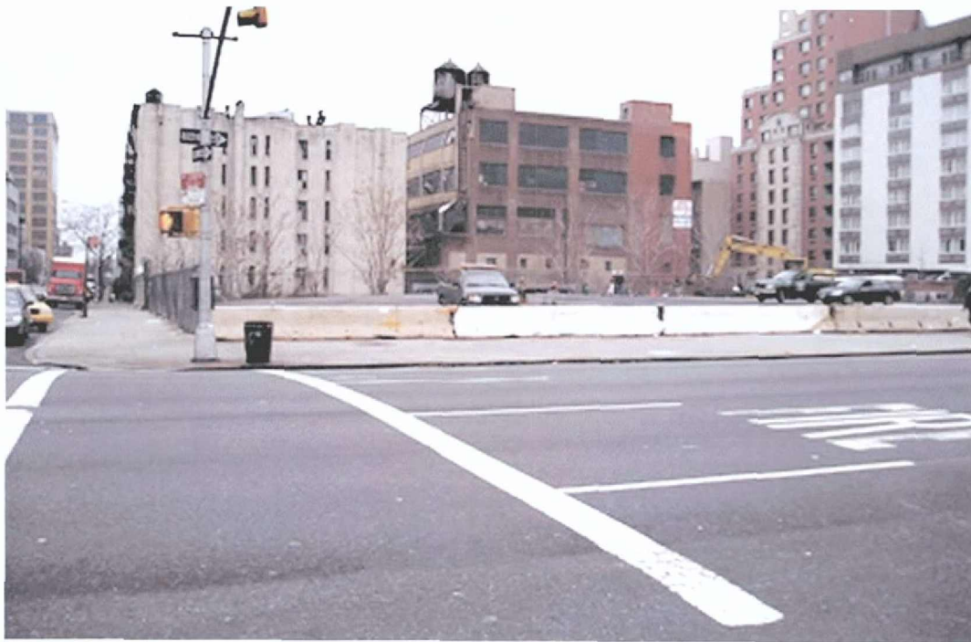
Plate 1. Block 1077, Lot 29 (proposed Shaft 25B) from the corner of Tenth Avenue and West 49 th Street; view to the west.
