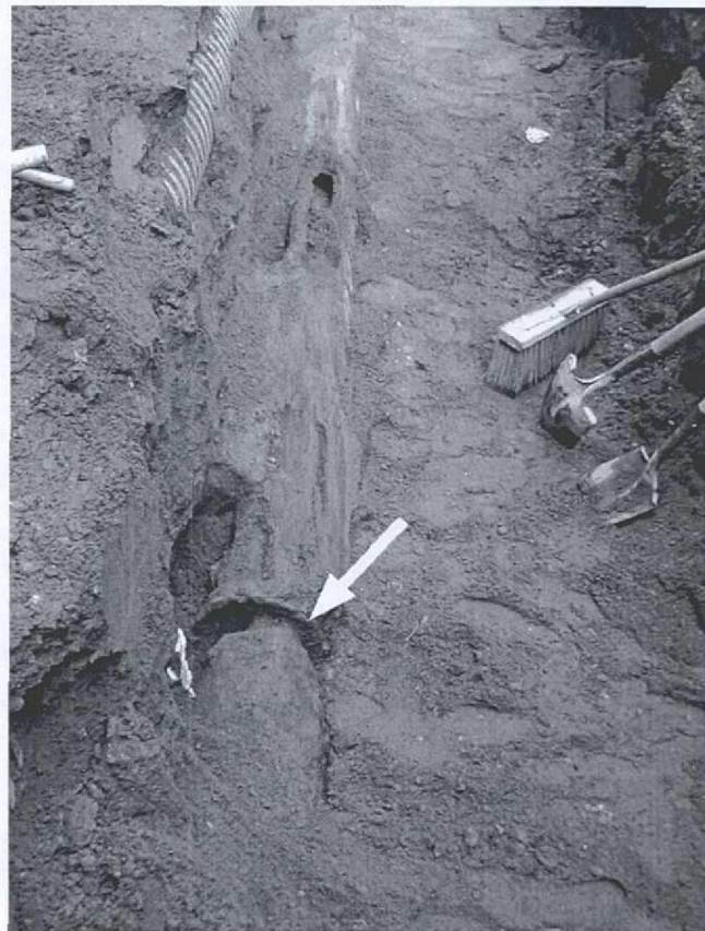
7 Intact joint (arrow) of partially exposed log water main in situ . Each segment is more than 13 feet long. (Geismar 10/22/04)
