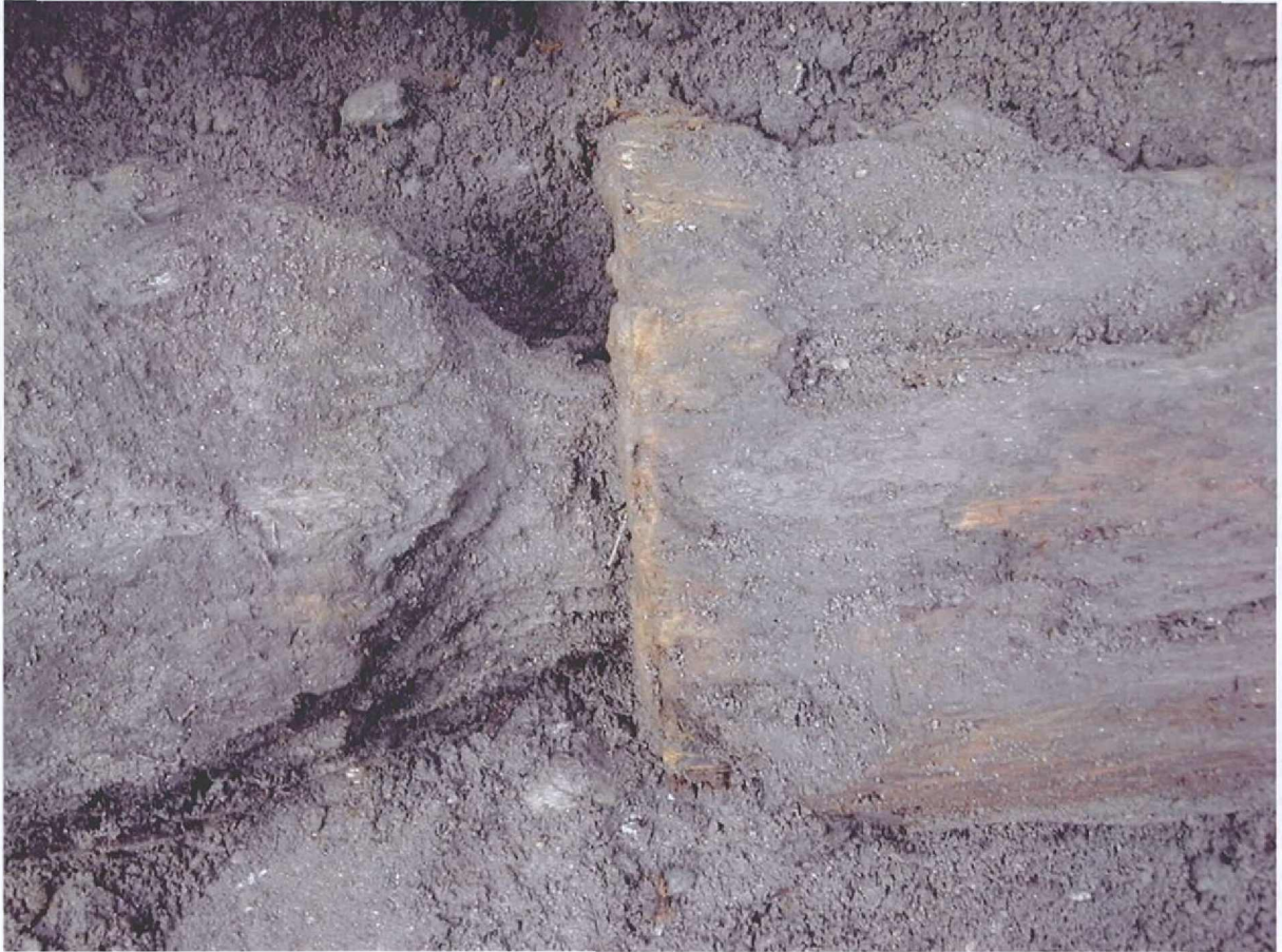
8 Detail of the exposed log water main joint, with the male (left) and female (right) components in situ and intact. (Geismar 10/22/04)
