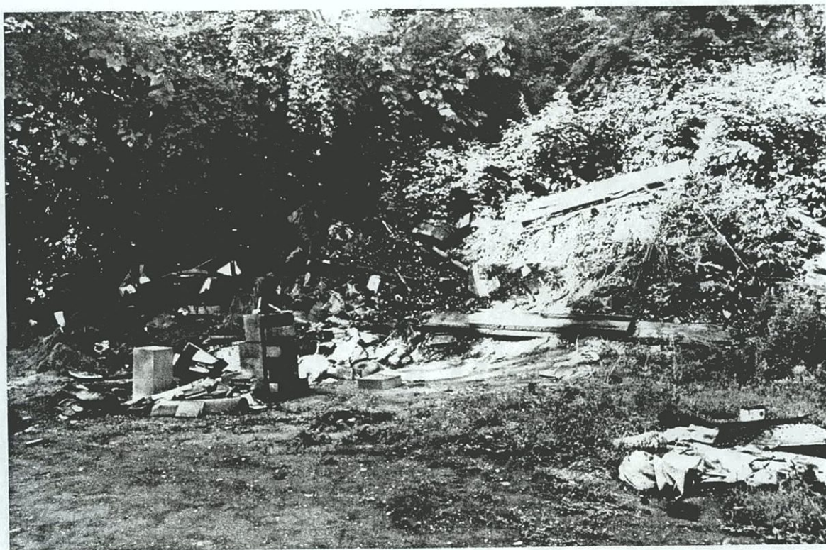
Plate C-28. Rubble and fill piles in the yard area associated with the condemned house located south of the Visitors Center (JMA Archeological Survey Area E3); view to the southwest.
