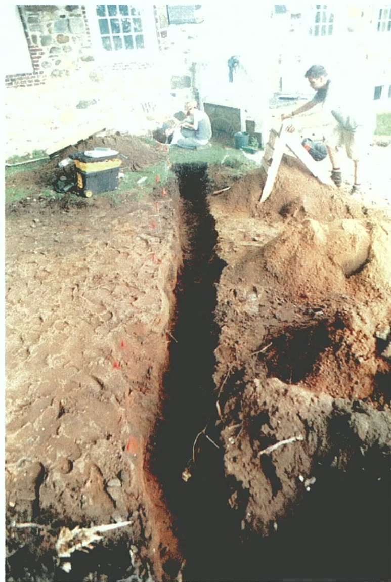
Plate C-35. JMA personnel excavating Trench F3 (archeological units F3.6–F3.16); view to the east.
