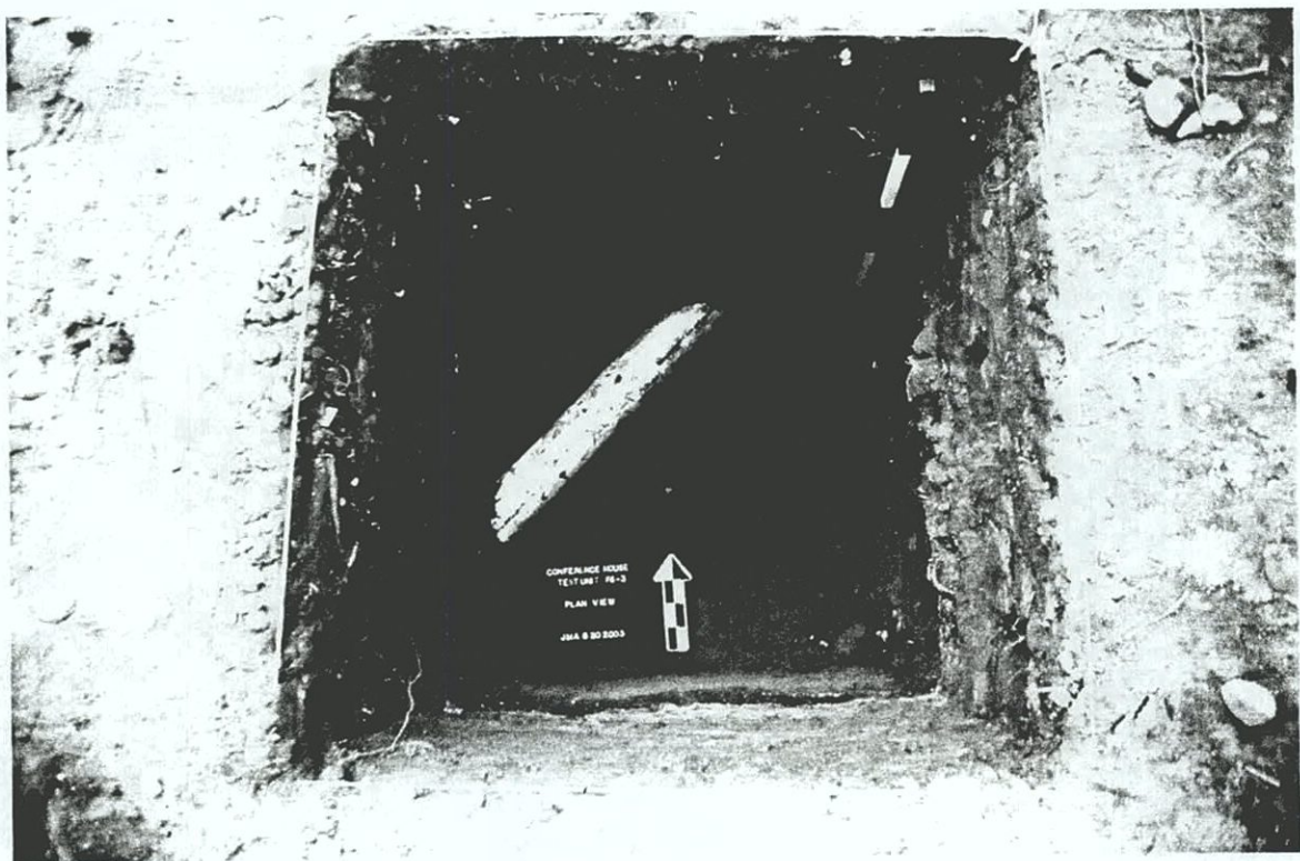
Plate C-45. Buried PVC pipe and disturbed soils documented in EU F6.3; view to the north.
