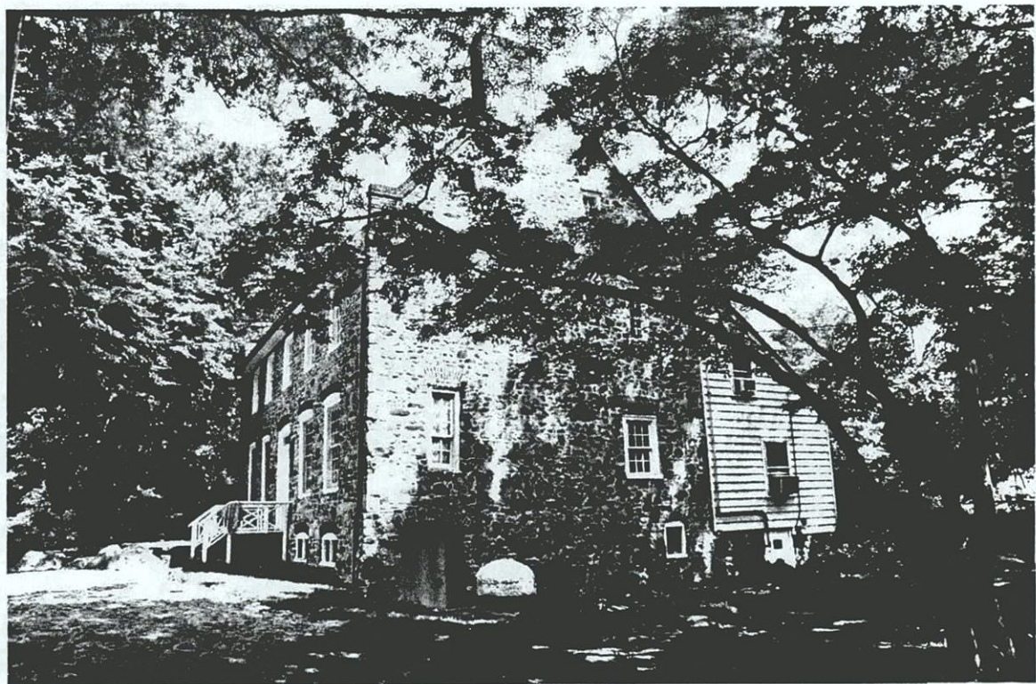
Plate C-30. South façade of the Conference House (JMA Archeological Survey Area F). Location of EU F2.7 west of door to Conference House extension at right of photograph.
