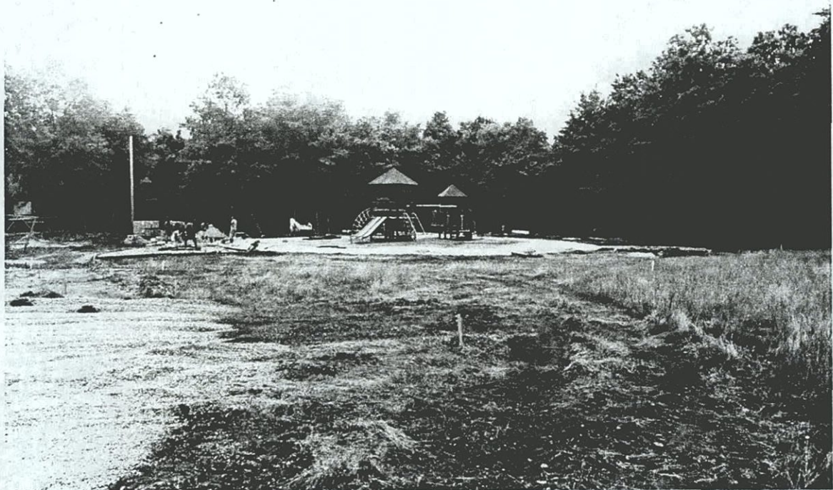
Plate C-24. Playground during construction within JMA Archeological Survey Area D1; view to the south.
