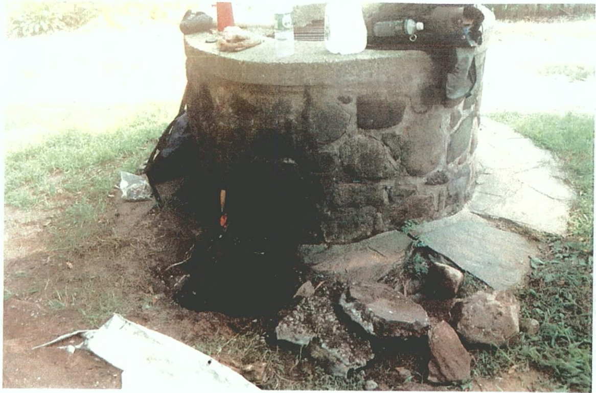
Plate C-42. Location of STU F6.0 relative to the existing well in the north yard of the Conference House; view to the south-southeast.
