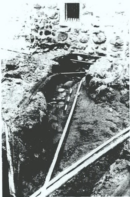
Stone feature observed in utility trench extending south from Excavation Unit F2.7.
