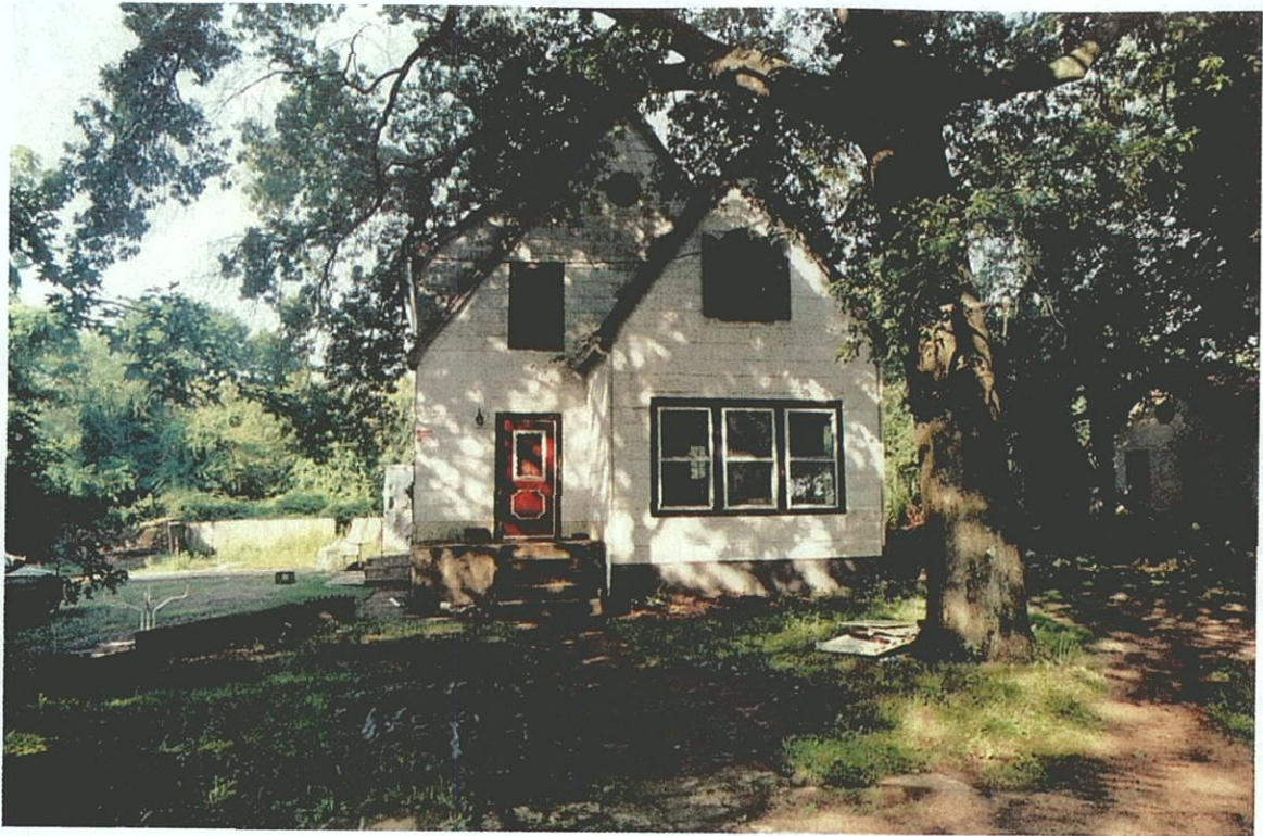
Plate C- 25. House proposed for demolition located south of the proposed Visitor's Center (JMA Archeological Survey Areas E1, E2, and E3); view to the west.
