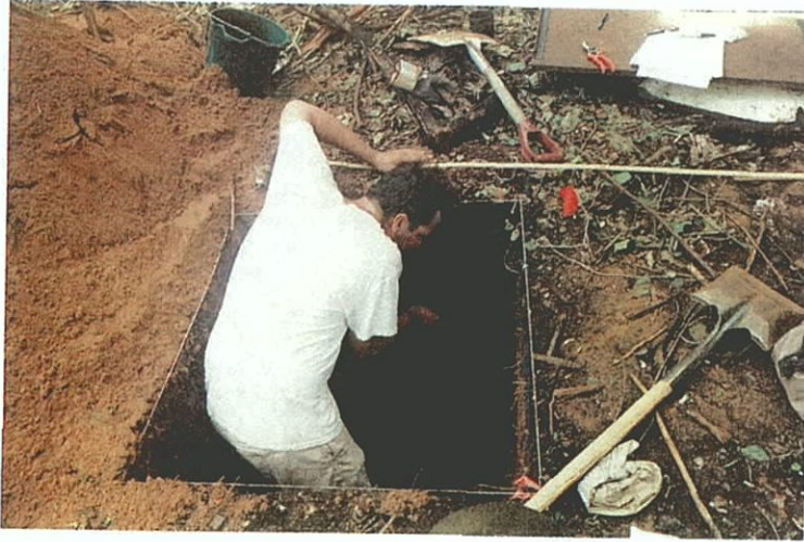
JMA personnel excavating Unit E2.2.
