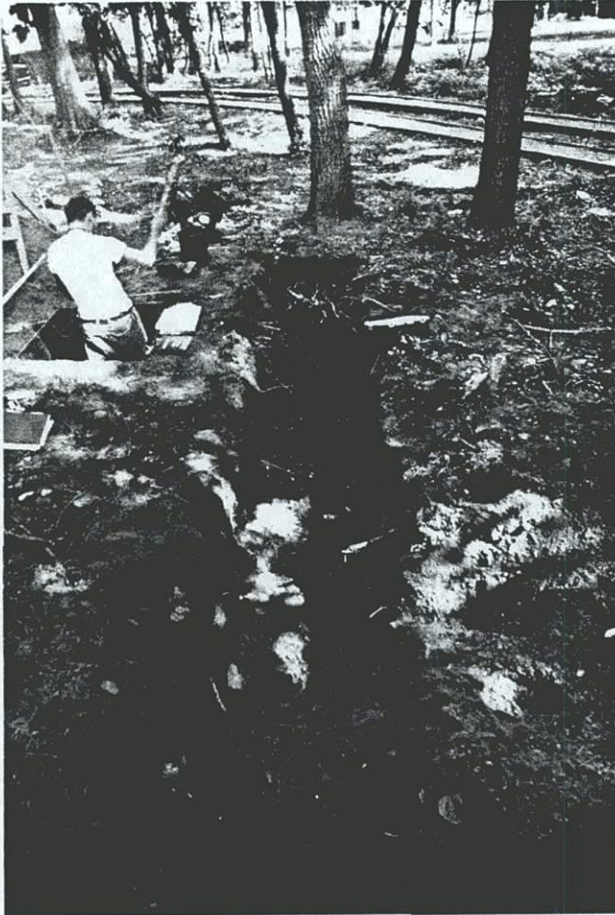
Location of EU F5.1 (left) relative to trench excavated by contractor; view to the south.
