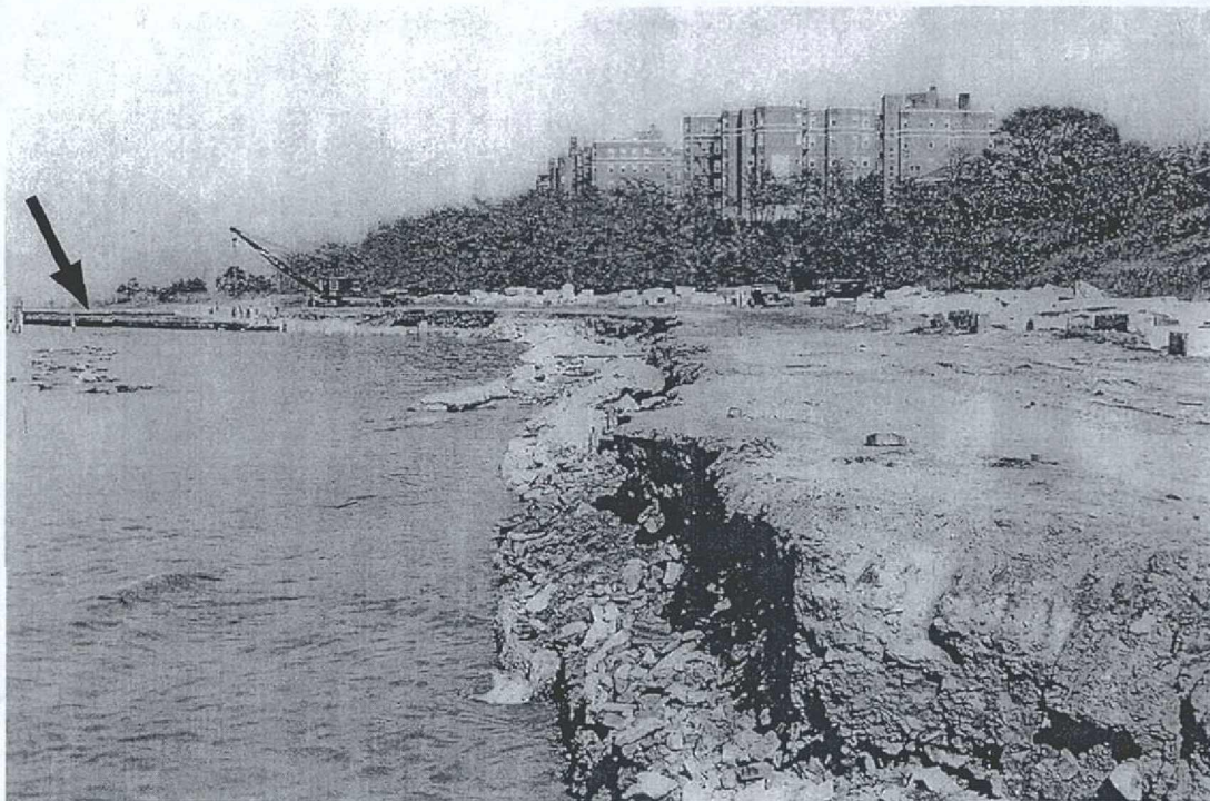
22 Shore (Belt) Parkway under construction in the vicinity, but south, of Bridge 13. Note fill and some cribbing (arrow) visible north of the project APE. (Photo Brooklyn Public Library)
