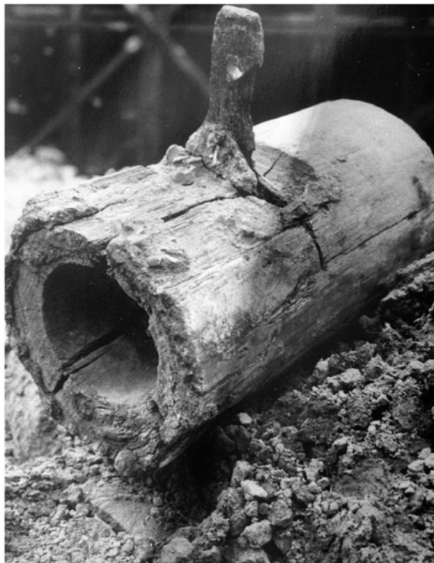
Figure 5 – Section of log water main with stop-cock in place. (Courtesy of Chase Archives)
