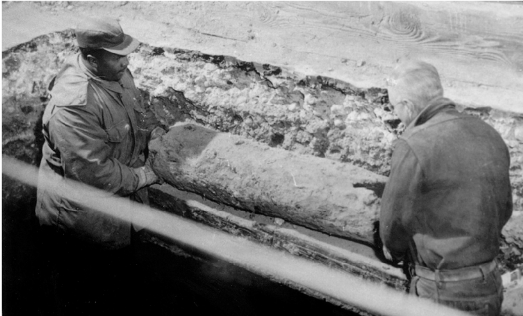
Figure 4 – Section of log water main being removed from intersection of New Street and Exchange Place in 1965. (Courtesy of Chase Archives)
