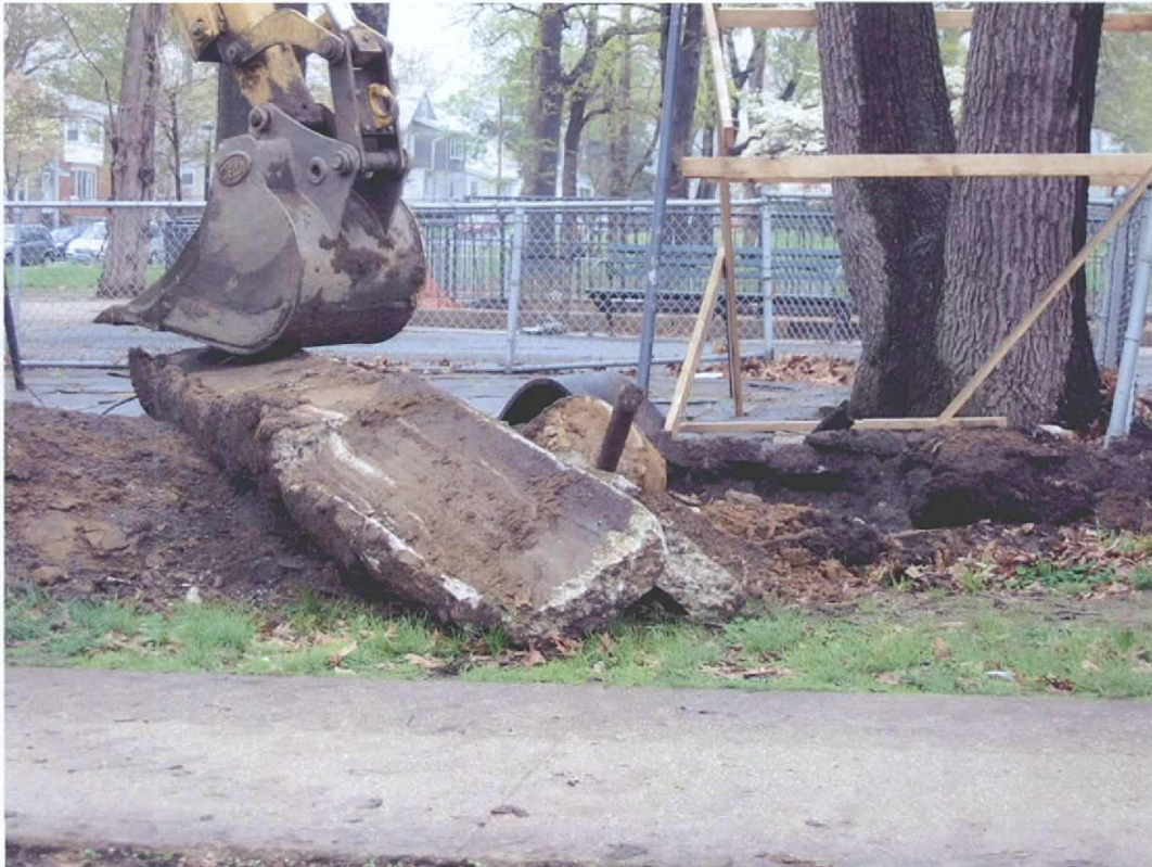
Photograph 05: Removal of existing chain link fence foot along 46 th Avenue
