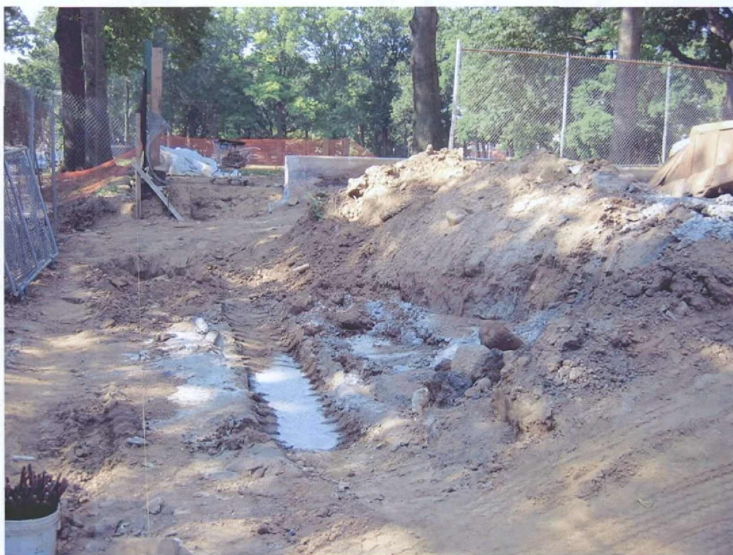
Photograph 08: Removal of concrete layer of northern playground
