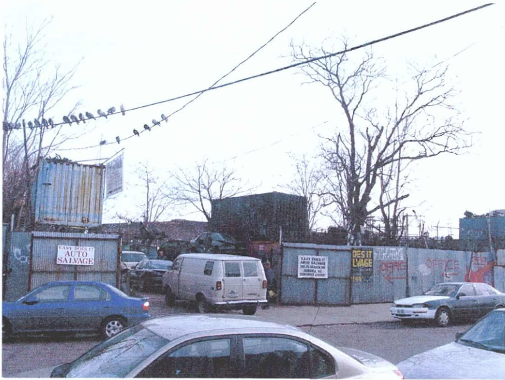
Fig. 38. View of part of site 411, block 10107, looking southeast from 150th Street.
