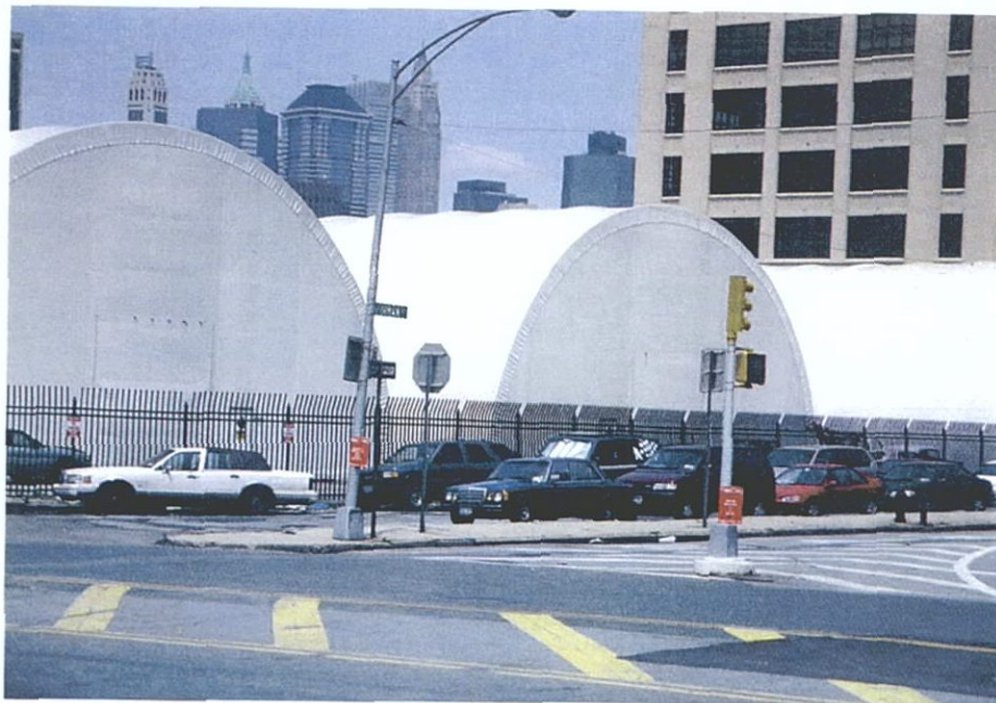
Photograph 48: Block 245, looking northwest from intersection of Furman Street and Atlantic Avenue. Domed storage sheds and Trade Facilities building in background.
