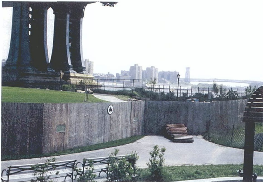
Photograph 10: Block 16, looking northeast from inside park. Manhattan Bridge pier on left. Note recessed area.
