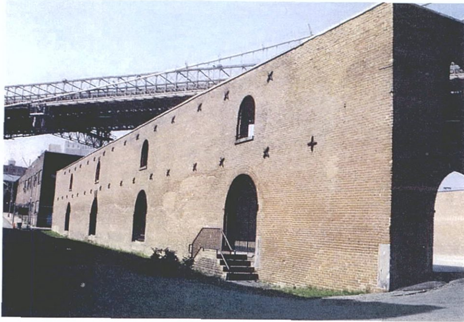
Photograph 19: Block 26, looking southwest from former Dock Street. Fulton Store remnant on right.
