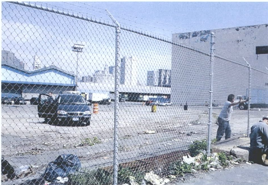
Photograph 34: Block 199, looking northwest Furman Street opposite line of Cranberry Street. Southern end of Cold Storage Warehouses on right. Pier 1 sheds on left.
