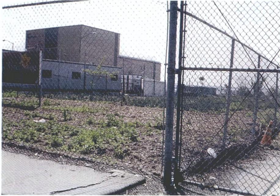
Photograph 39: Block 199, looking west from Furman Street north of line of Pierrepont Street. Transit building in left background.
