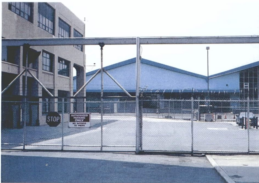
Photograph 46: Block 245, looking west from Furman Street along Joralemon Street. Trade Facilities building on left; Pier 5 sheds in background.
