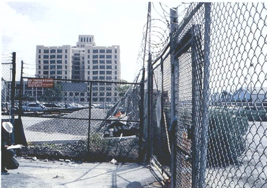
Photograph 50: Block 245, looking south from interior of block showing parking lots and storage areas. Trade Facilities building in left background; Pier 5 sheds in right background.
