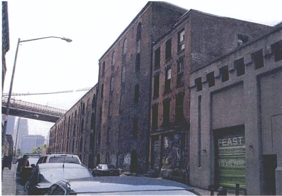
Photograph 17: Block 26, looking northwest from Water Street. Empire Stores on left, former factory building and Gair Building on right.
