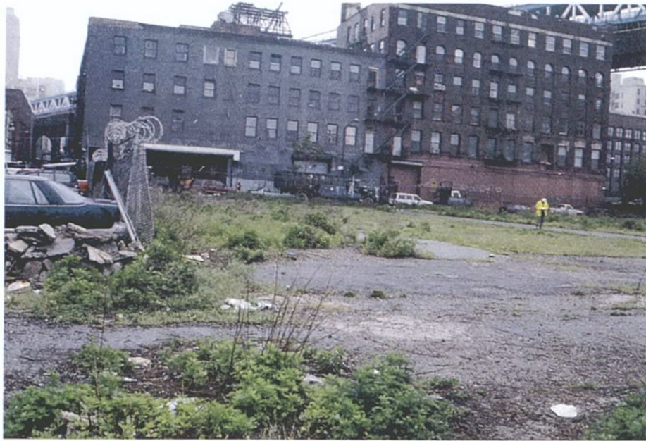
Photograph 3: Block 1, looking south from waterfront with Pearl Street on left.
