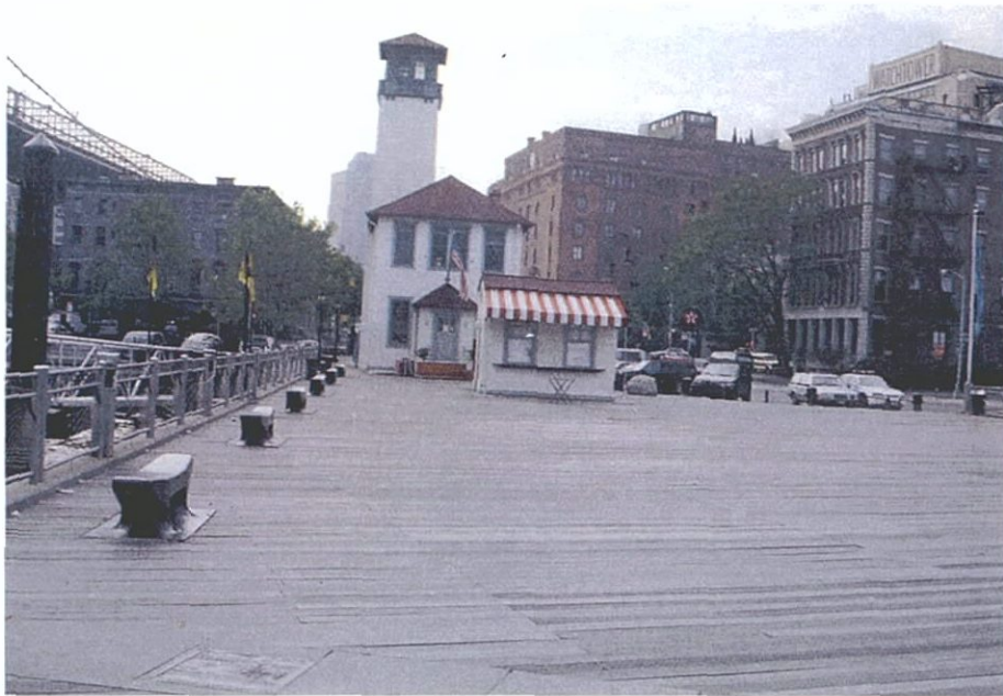
Photograph 13: Block 25, Lot 1, looking east from waterfront along Recreation Pier. Former Fire Boat house (now an “ice cream factory”) in background. Slip on left.
