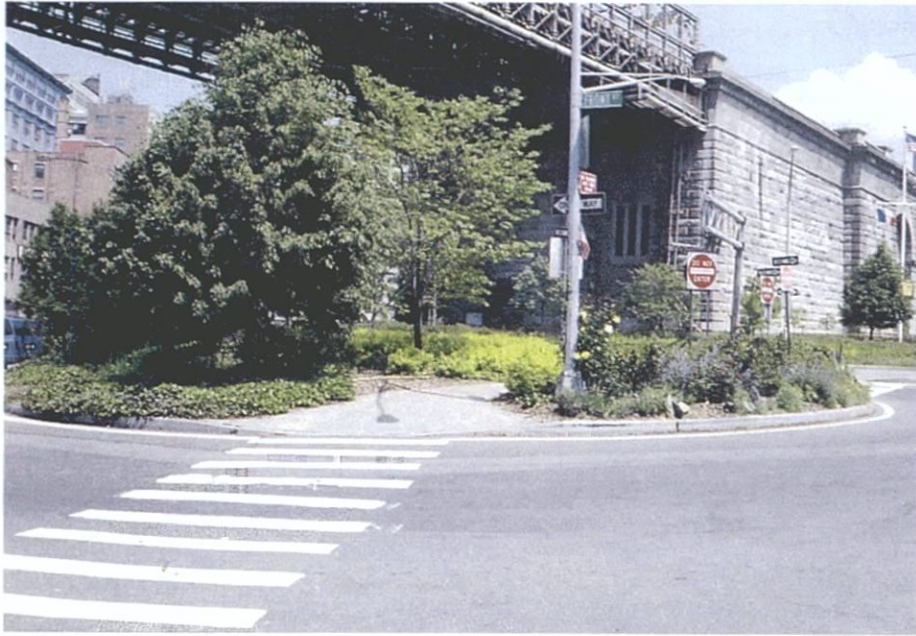
Photograph 23: Block 45, looking northeast from intersection of Front Street and Fulton Street. Traffic island formerly part of the block. Brooklyn Bridge in the background.
