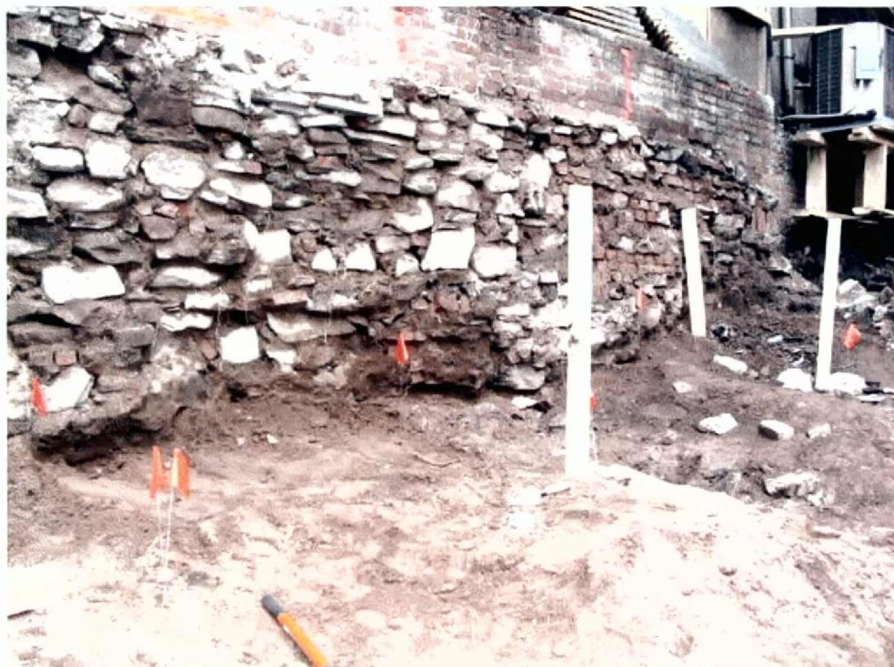
Photograph L: Facing southeast, showing the makeshift partially mortared stone and brick wall.
