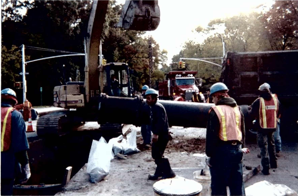
Plate 1. Installation of main at approximately Sta. 115+50; view to the east.
