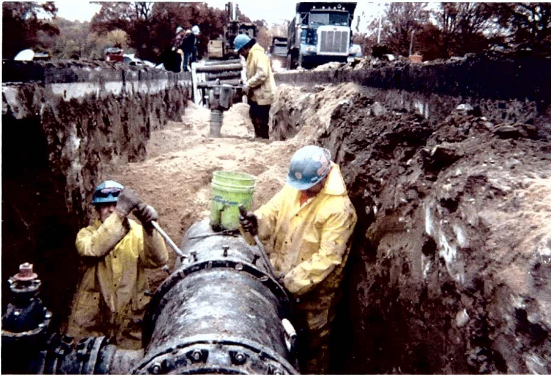
Plate 2. Installation of main at approximately Sta. 136+50; view to the west.
