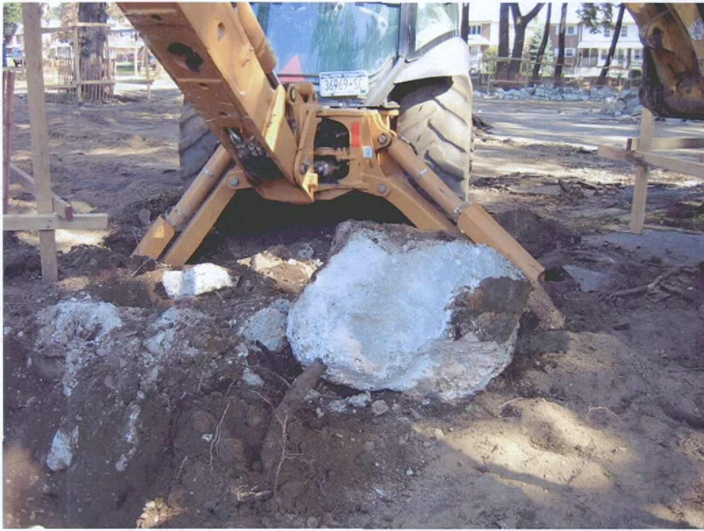
Figure 15: Removal of existing catch-basin in southern half of Park
