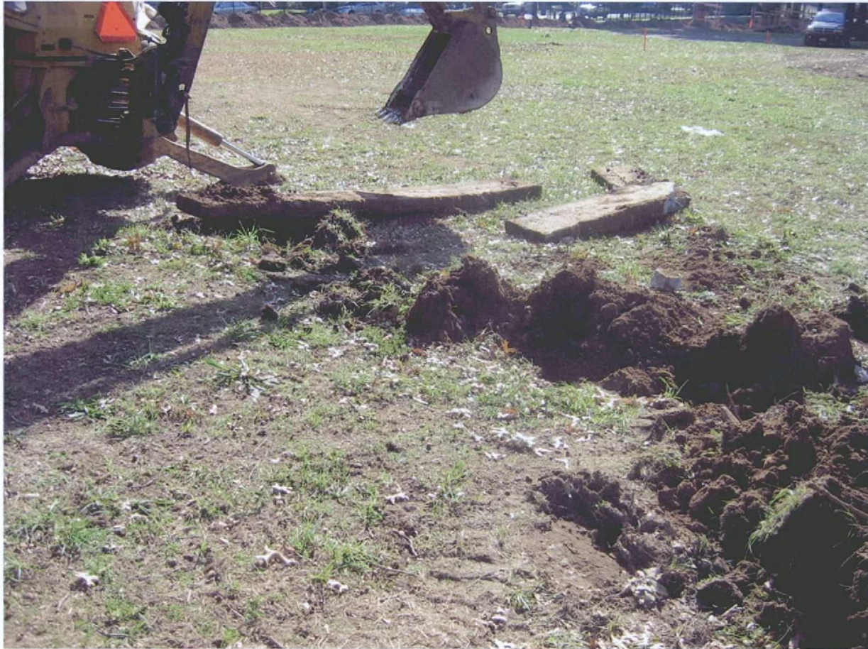
Figure 07: Excavation Area E: Park Interior - Removal of interior curbing
