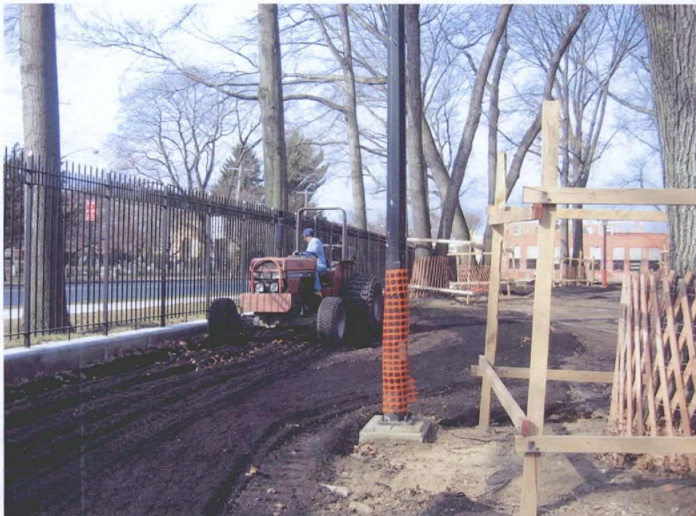
Figure 14: Installation of new fill in southern half of Park
