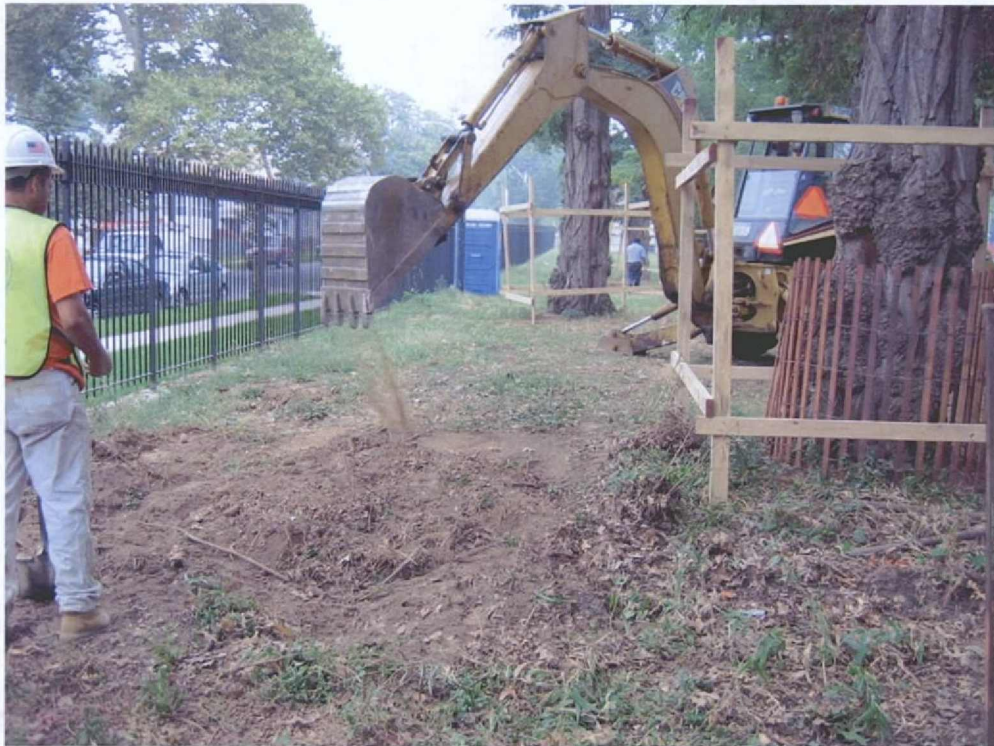
Figure 11: Excavation for new Dry Well along 164th Street
