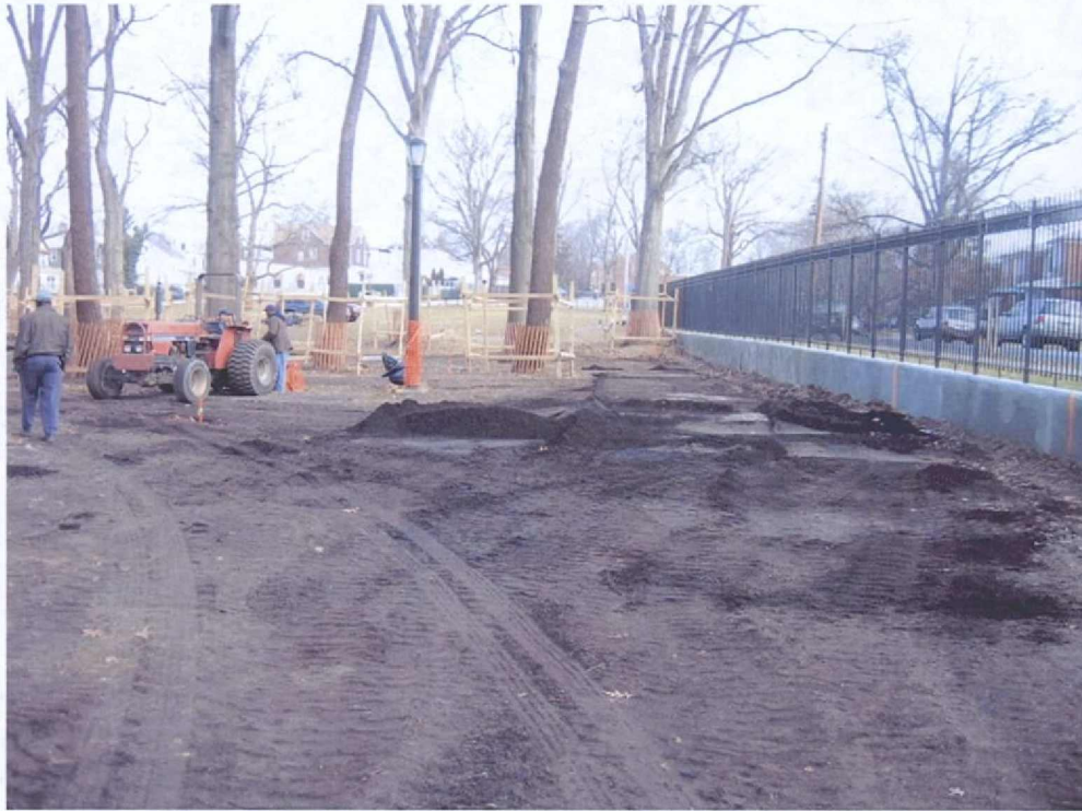
Figure 13: Installation of new fill in southern half of Park
