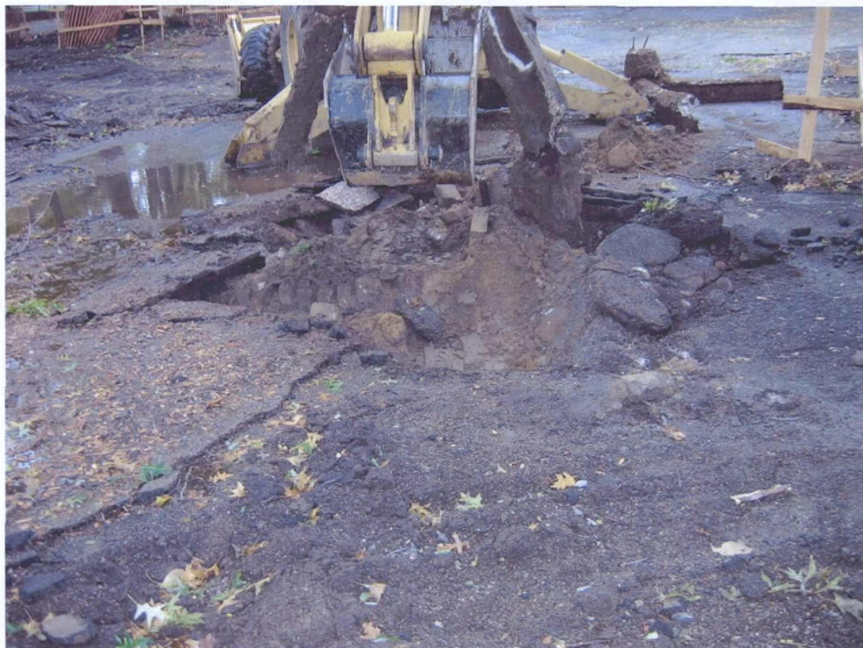
Figure 10: Excavation Area F: - Removal of Asphalt and Concrete from the previously Existing 1930s Playground.
