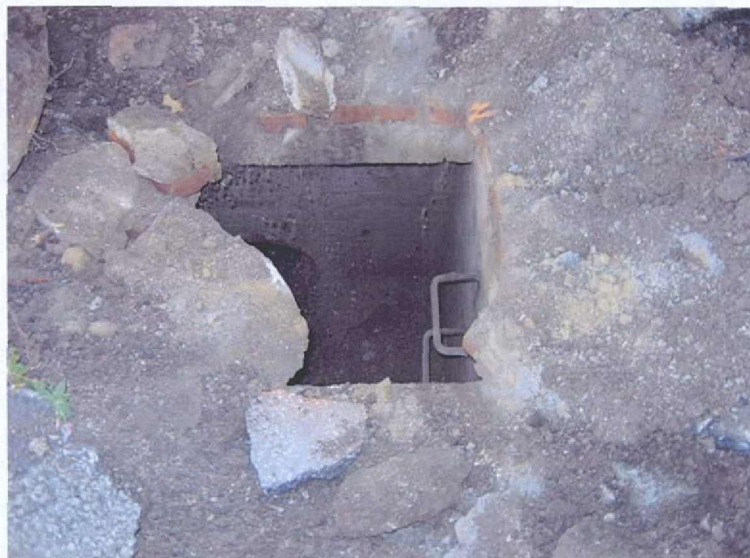
Figure 03: Excavation Area B: 46 th Avenue - old dry well slated for replacement
