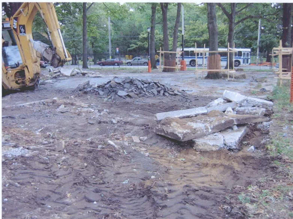
Figure 12: Removal of existing surface in southern half of Park
