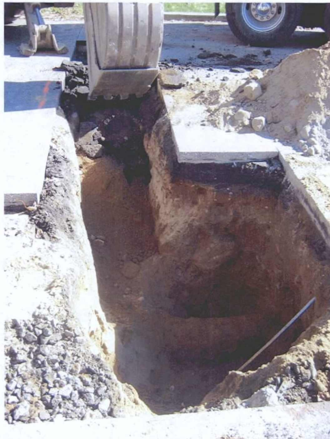
Figure 06: Excavation Area D: Water Connection 164 th Street - Water Connection
