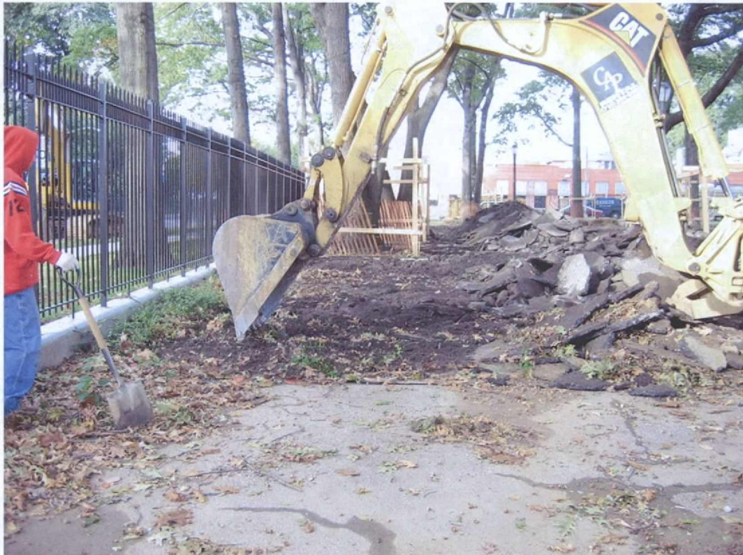
Figure 09: Excavation Area F: - Removal of Asphalt and Concrete from the previously Existing 1930s Playground.
