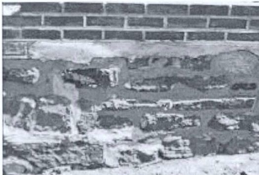
Inappropriate use of high strength mortar on a historic stone and brick wall. This technique of using the mortar has obscured the unit masonry. The type of mortar used will entrap moisture behind the masonry surface, causing damage.
