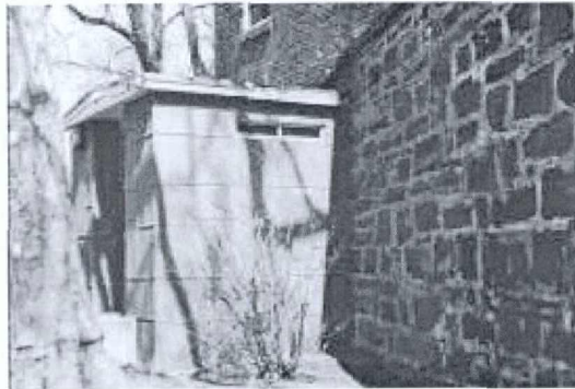
A small addition placed on a secondary facade of a brick and stone building in the historic district. The surface of the addition attempts to emulate stone, unsuccessfully. The design is inconsistent with the existing structure. This addition is an intrusion.
