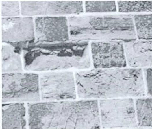
Illustration of deteriorated stone typical of the effect trapped moisture will have on masonry surfaces. This could be caused by the use of improper mortar in tuckpointing and/or abrasive cleaning of the masonry.
