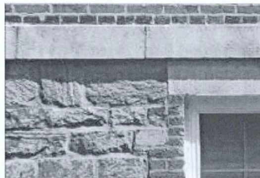
Appropriate use of mortar on a historic stone and brick wall. This technique of using the mortar has preserved the unit masonry. The type of mortar used will allow moisture behind the masonry surface to escape, preventing damage.
