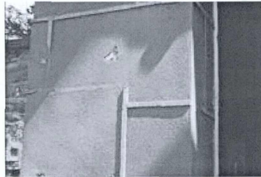
A close-up of the fake stone surface shown to the left. The base material is stucco, with applied mortar designed to suggest stone blocks. The design is inappropriate and unsuccessful. The deterioration of the materials suggests that they are not durable.
