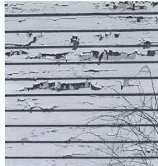
Painted wood shiplap siding typical of frame buildings in the Historic District. Deteriorated paint is easily replaced. Deterioration is typically caused by excessive moisture generated inside the building.
