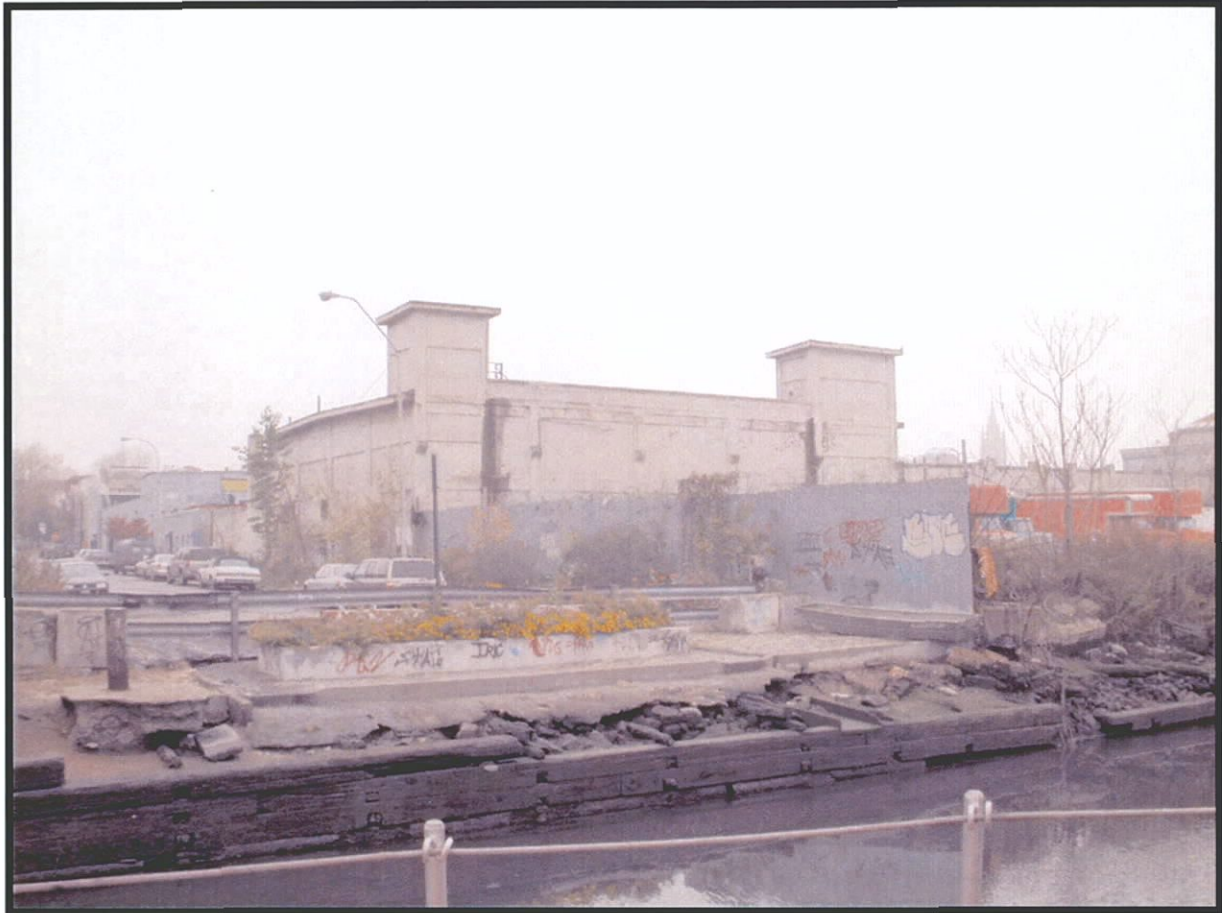
Plate 3.23. Gowanus Canal Assessment of Eligibility: View North of Forman Blades Lumber building (Photographer: James Lee, November 2003) [HRI Neg.# 03070 D1-34].
