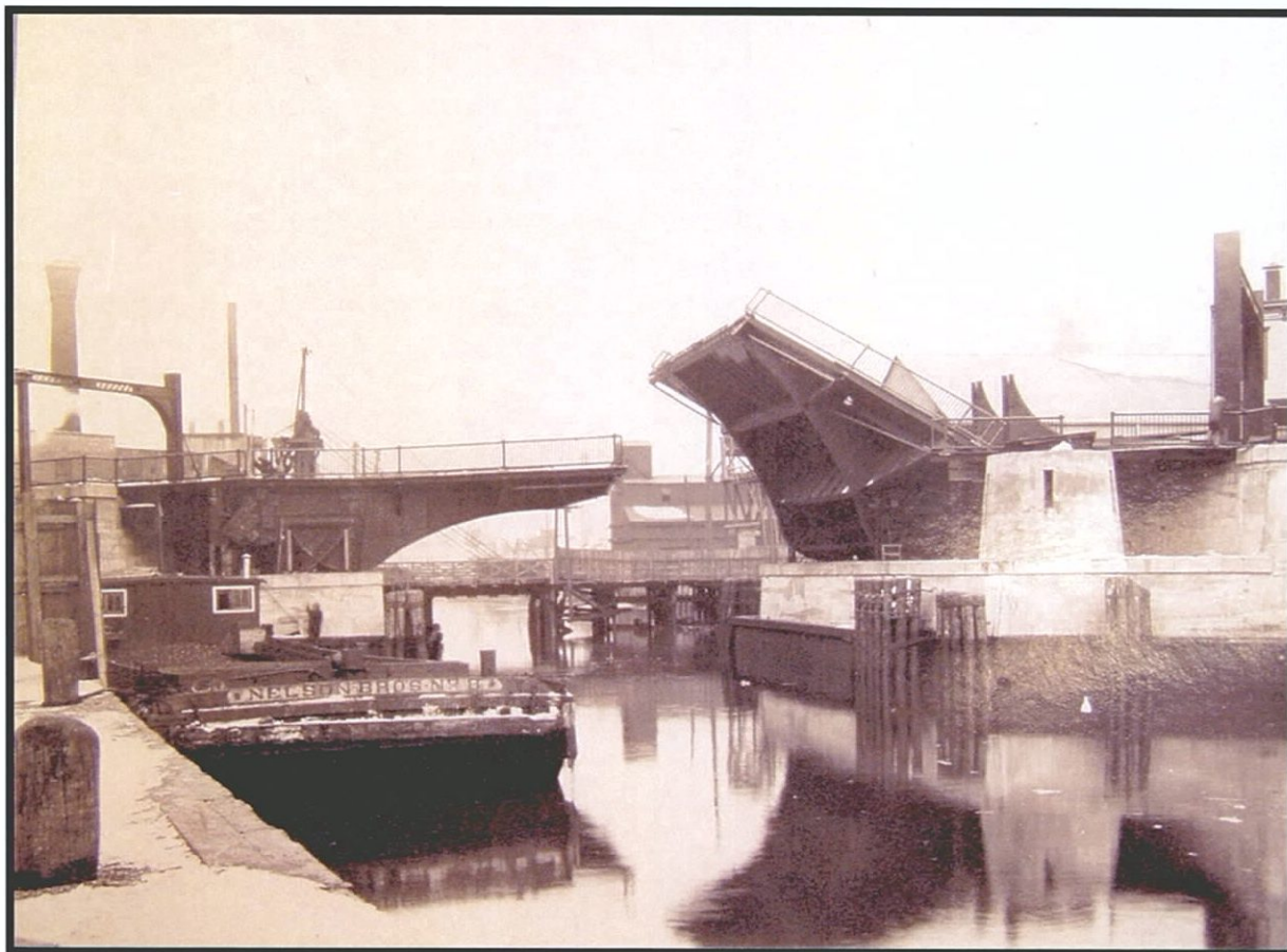
Plate 2.5. Gowanus Canal Assessment of Eligibility: View southwest of the Union Street Bridge nearing completion. Circa 1905. The Carroll Street Bridge is visible beyond. Source: Brooklyn Public Library.
