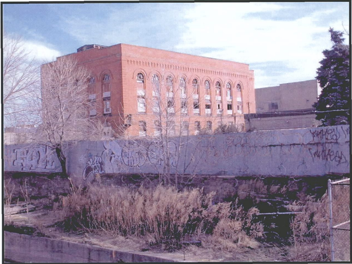
Plate 3.22. Gowanus Canal Assessment of Eligibility: View East of Former Brooklyn Rapid Transit Power House (Photographer: Charles Ashton, January 2004) [HRI Neg.# 03070 D3-07].
