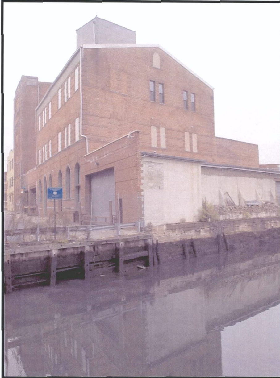
Plate 3.6. Gowanus Canal Assessment of Eligibility: View northeast at Bond Street, showing several types of concrete bulkheads of concrete additions to timber cribwork bulkheads. The circa 1900 building at the center of the view was formerly used by an ice company and a brewery, but probably not serviced by the canal (Photographer: Thomas Flagg November 2003) [Source: Raber Associates].
