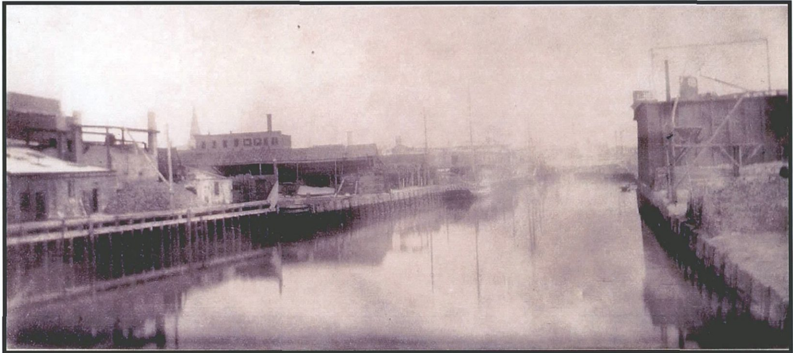
Plate 2.3. Gowanus Canal Assessment of Eligibility: View of an unidentified section of the Gowanus Canal. Circa 1877. Taken within about a decade of completion of the main canal, this view suggests the rapid industrial growth along the waterway. Most of the canal walls shown appear to be cribwork with timber fenders, but those at left may be timber sheet piling. Source: Brooklyn Public Library.
