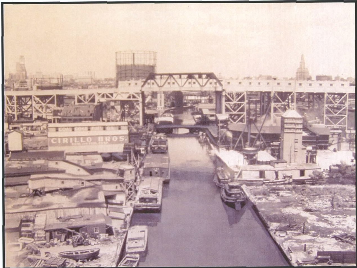
Plate 3.13. Gowanus Canal Assessment of Eligibility: View northeast of the Gowanus Canal, 9th Street bridge and the trestle for the F and G Trains. 1952. Taken from the new Gowanus Expressway overpass, this view also includes the Cirillo Bros. Coal & Fuel Co. at left, Cranford Co. concrete & asphalt plant at left just beyond covered lighter in 11th Street Basin and a number of tugboats, covered lighters, and hold barges. Source: Brooklyn Public Library.
