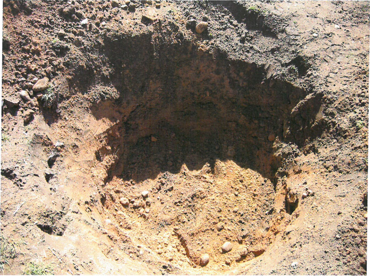
Figure 07: T01B - Excavation completed
