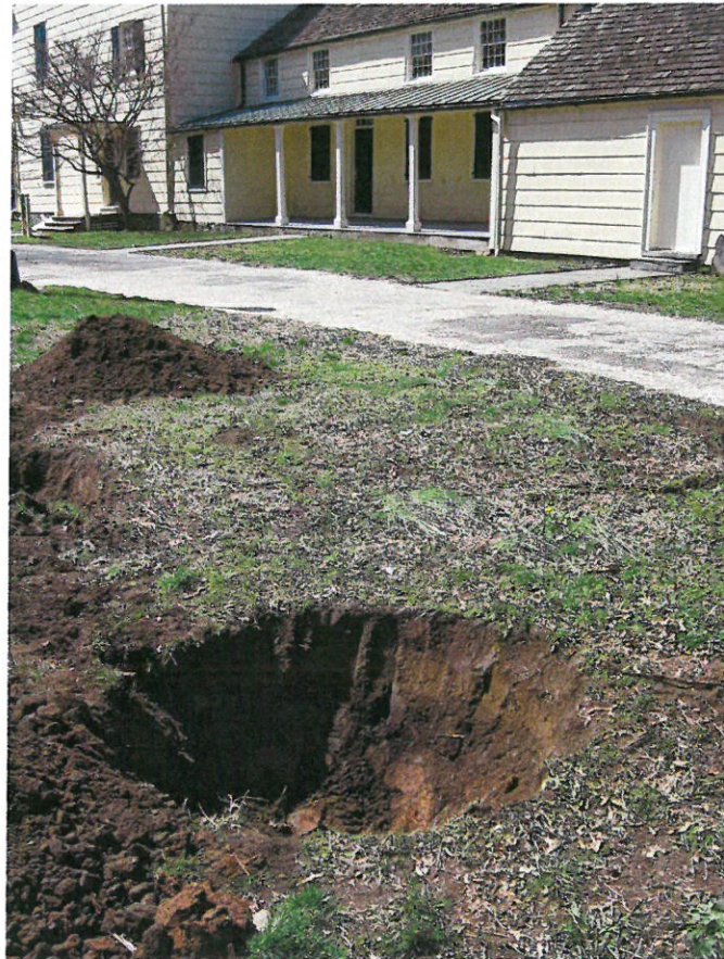
Figure 14: T03C: Completed Excavation
