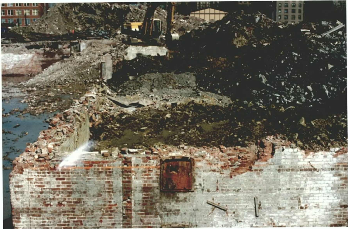
Plate 3 Debris Being Removed from Basement of Eastern Extensions of School Building View North
