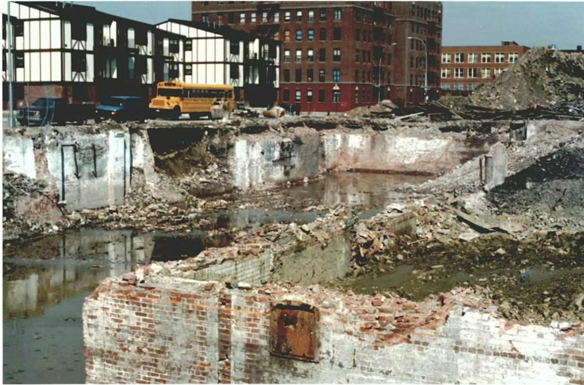
Plate 1 Basement of ca. 1915 School Building After Removal of Demolition Debris - Note Debris Pile on Northern Portion of Site View Northwest
