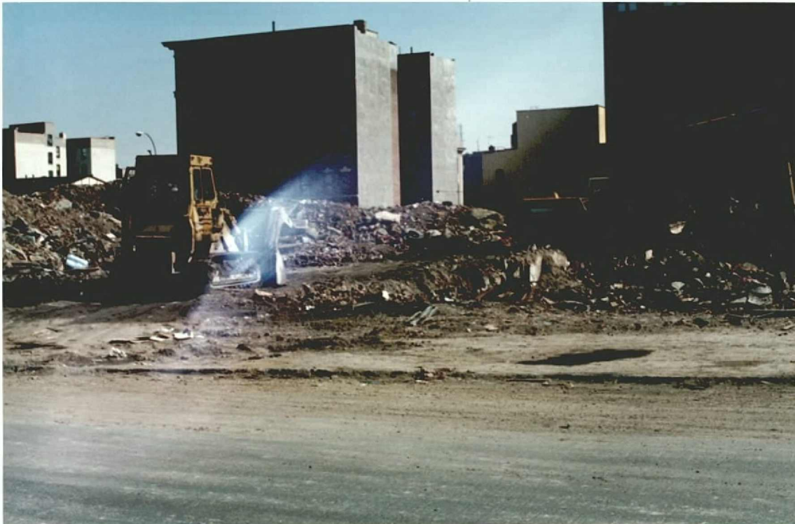
Plate 2 Debris Being Removed from Northern Portion of Site View East from West Side Trinity Avenue
