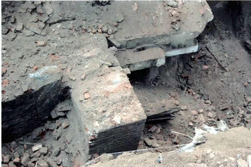
Fig. 14. View of the brick pillar at the north corner of 24 Beekman Street, looking west (the back wall of 22 Beekman Street adjoining has collapsed).
