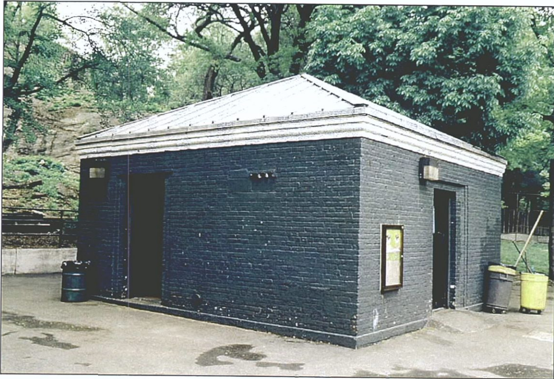
Photo 17 - Park Comfort Station, View Northwest.
