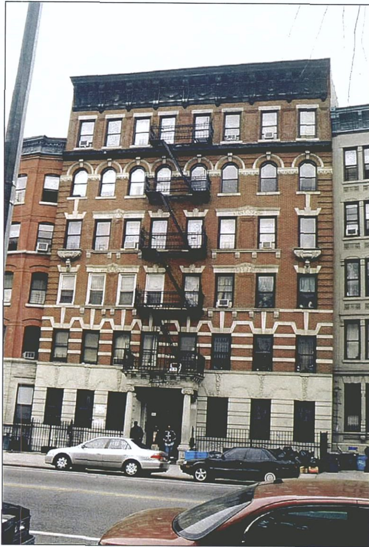
Photo 15 - 448-450 St. Nicholas Avenue, View East.
