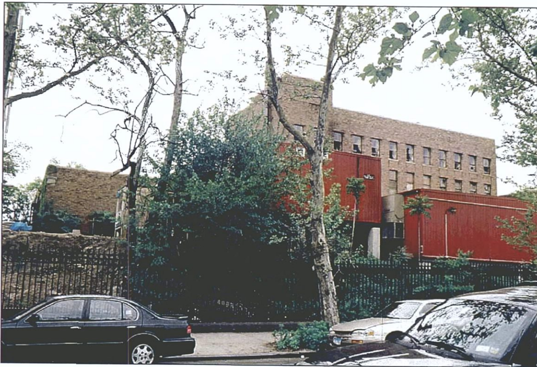
Photo 18 - Eisner Hall, View Northwest.
