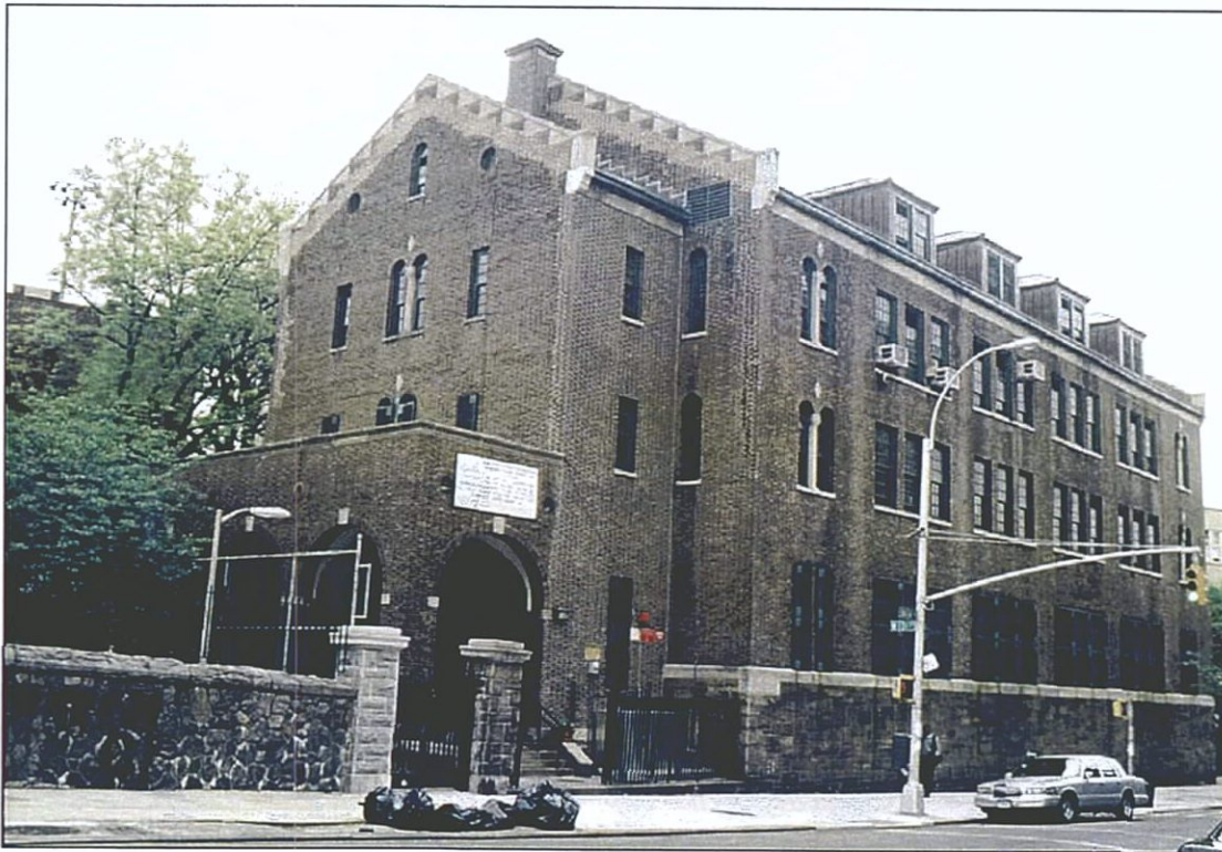
Photo 20 - Mott Hall, View Southeast.
