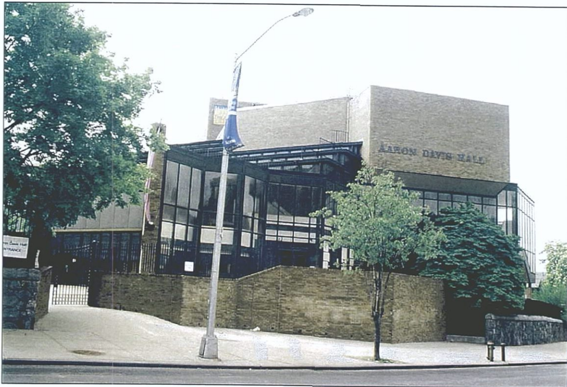
Photo 24 - Aaron Davis Hall, View Southeast
