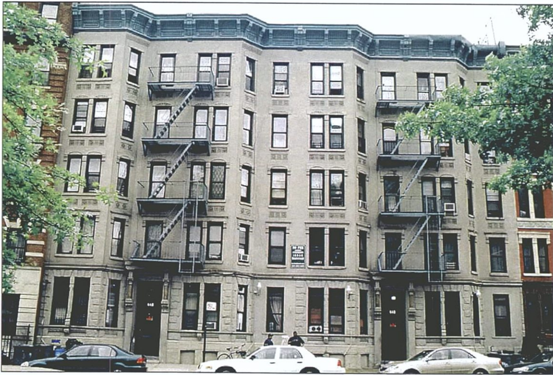
Photo 14 - 440-446 St. Nicholas Avenue, View East.
