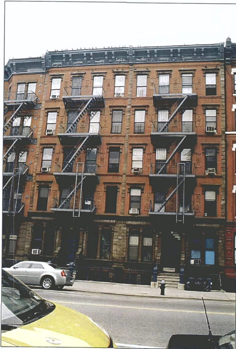
Photo 12 - 428-430 St. Nicholas Avenue, View East.
