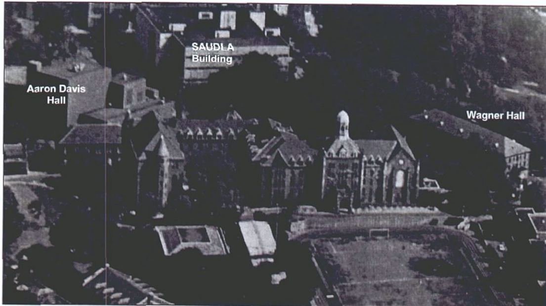
Photo 8 - 1983 Aerial View of the Finley Student Center. Compare this View to the Modern Aerial Shown in Photo 1. View North. (Source: CCNY Archives).
