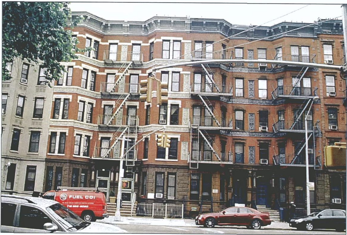
Photo 13 - 432-438 St. Nicholas Avenue, View East
