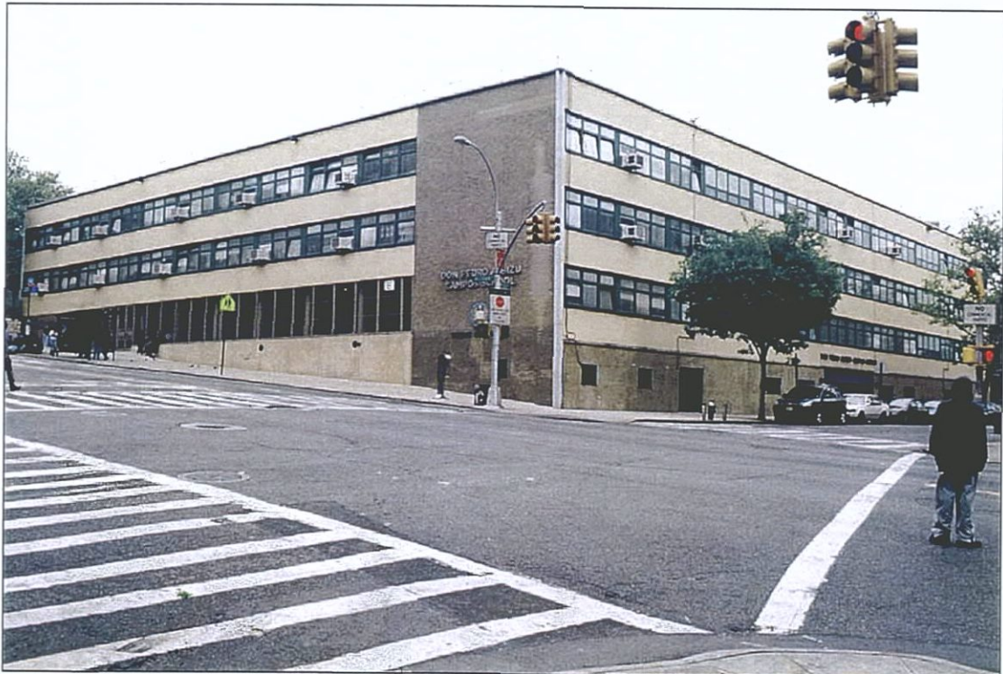
Photo 26 - P.S. 161, View Northeast.
