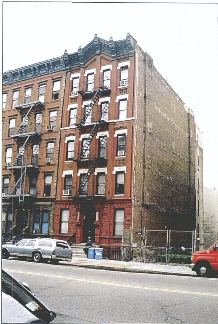
Photo 11 - 426 St. Nicholas Avenue, View East.
