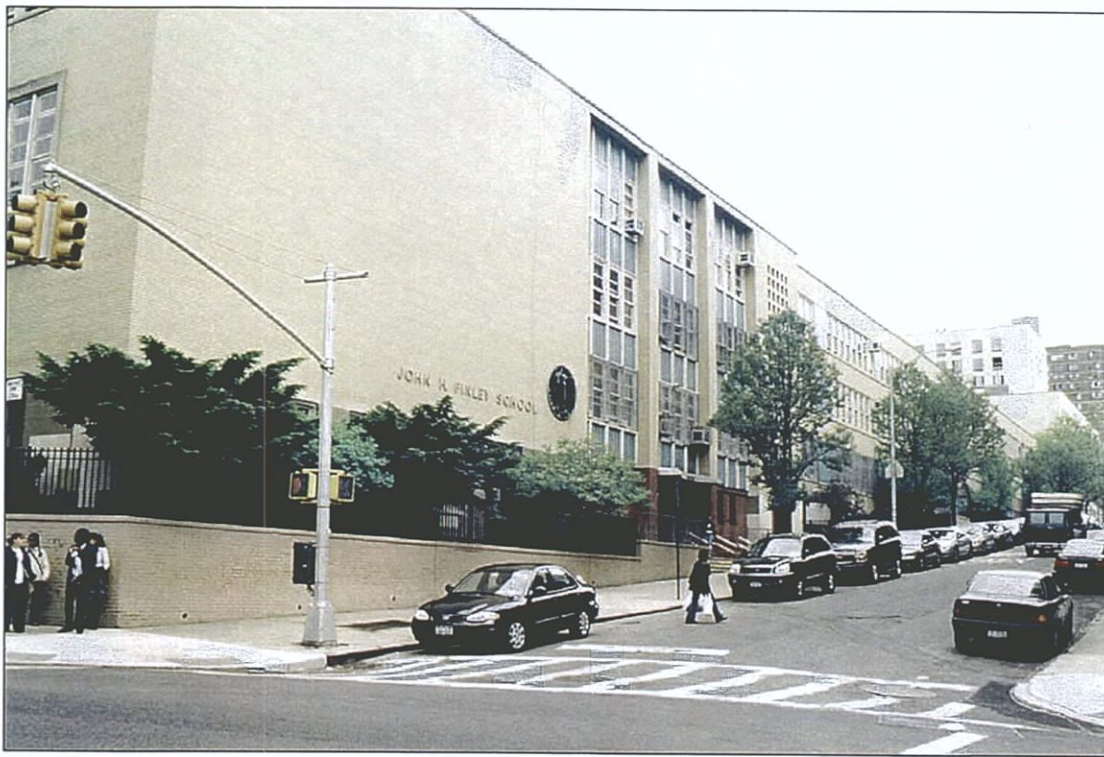
Photo 19 - P.S. 129, View Northeast.
