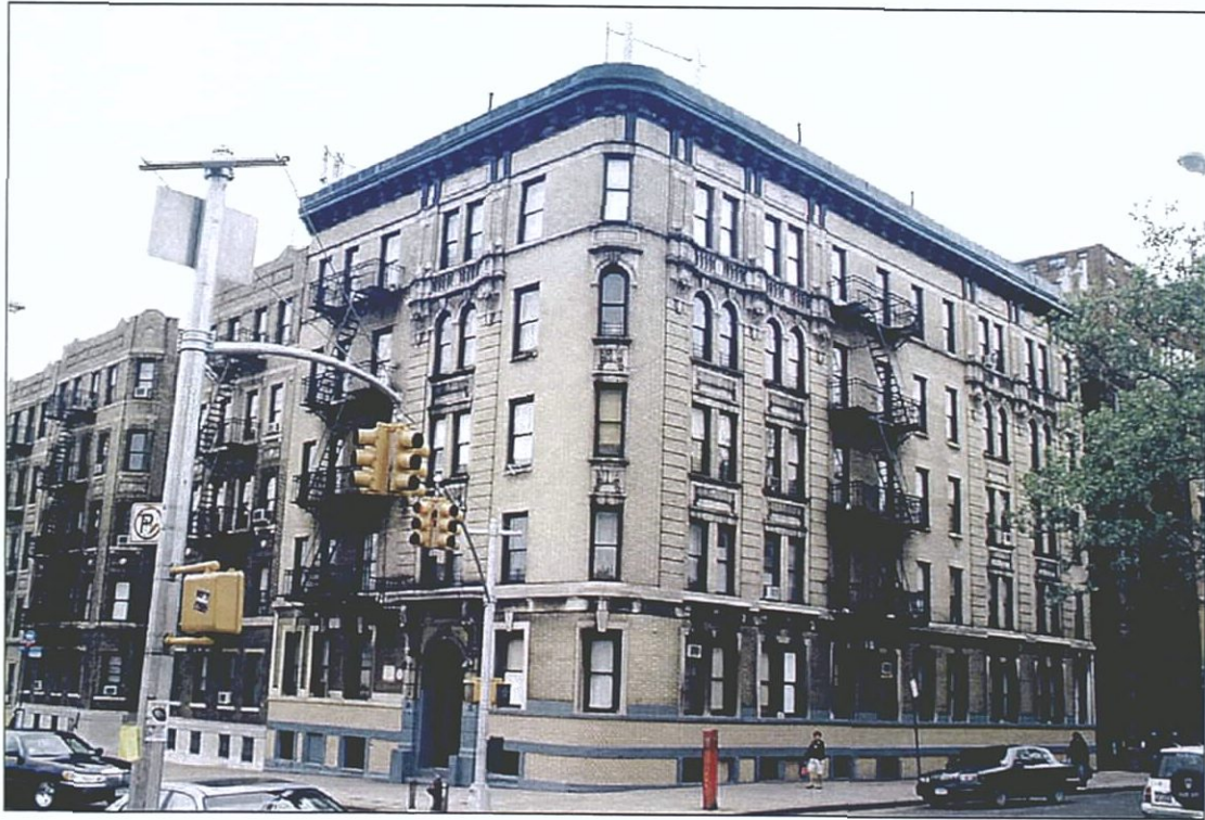
Photo 27 - 110 Convent Avenue, View Southwest.
