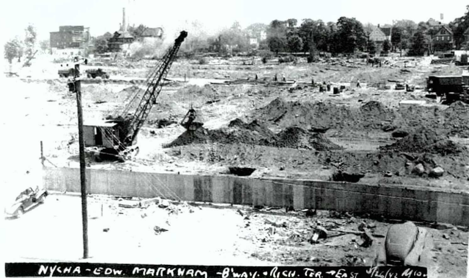
Project site showing grading and excavation of property prior to construction of Markham Gardens buildings. Note large soil stockpiles, large pits, and undulating surface. View looking east from Broadway near Richmond Terrace.
