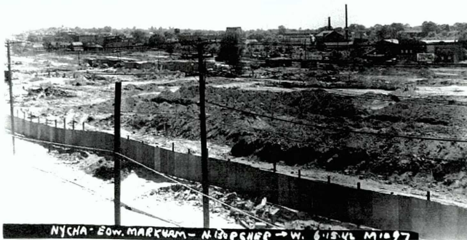
Project site showing grading and excavation of property prior to construction of Markham Gardens buildings. Note large soil stockpiles, large pits, and undulating surface. View looking southwest from North Burgher Avenue.
