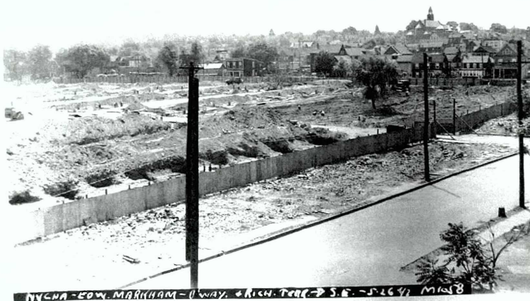
Project site showing grading and excavation of property prior to construction of Markham Gardens buildings. Note large soil stockpiles, large pits, and undulating surface. View looking southeast from Broadway near Richmond Terrace.
