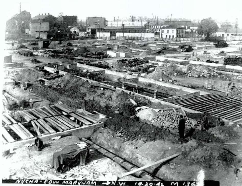
Project site showing foundations for apartment buildings and disturbed ground surface surrounding them. Note utility pipe entering foundation in foreground. View looking northwest from interior of site.
