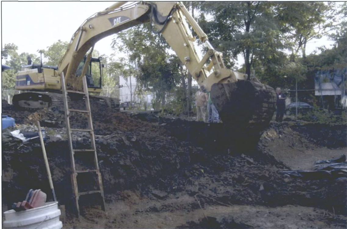
Photo 28: Mechanical Excavation of Trench 2. View Northeast.
