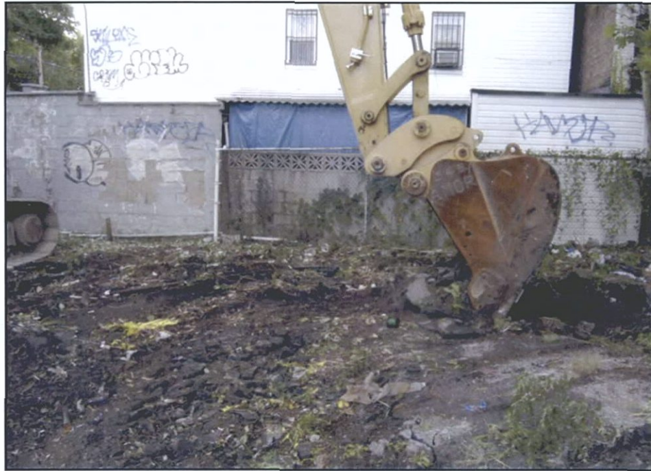
Photo 1: Mechanical Excavation of Trench 1. View South.
