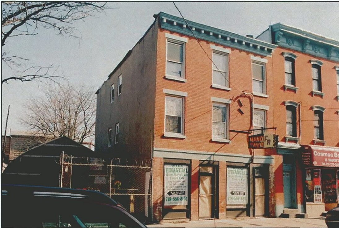
Photo 24 - 593 Bay Street (Survey No. 25) Looking Southeast
