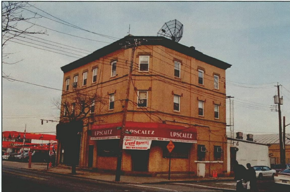
Photo 10 - 521 Bay Street (Survey No. 11) Looking Northeast
