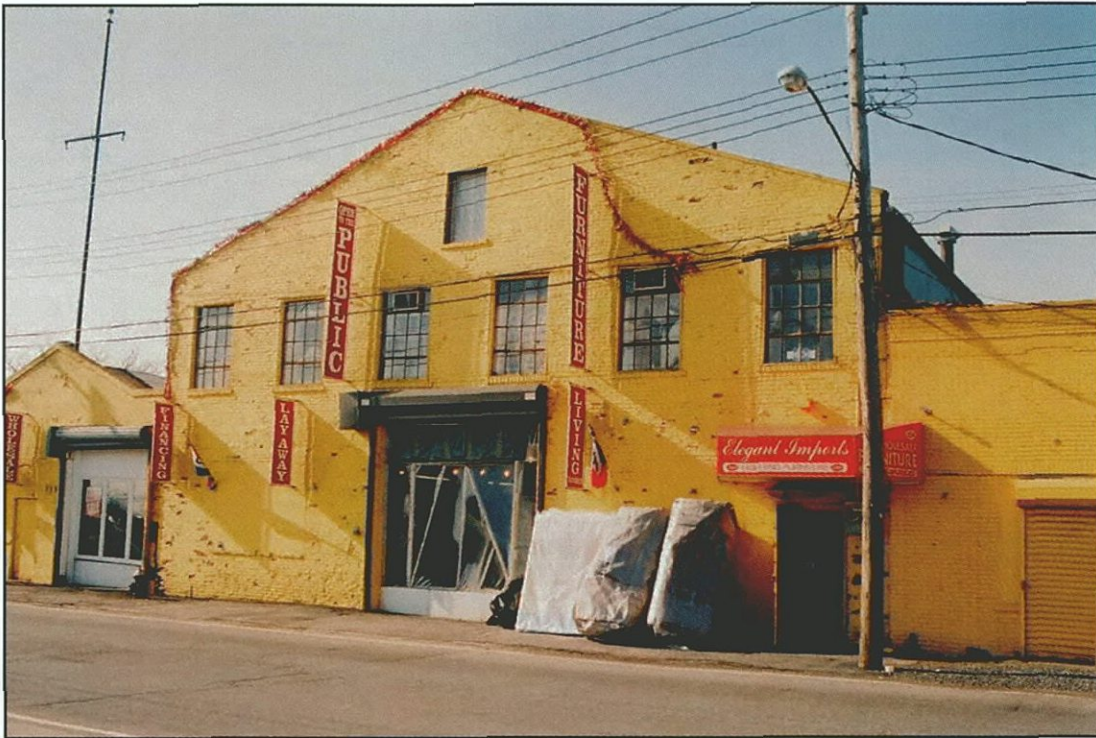
Photo 19 - 354 Front Street (Survey No. 20) Looking West
