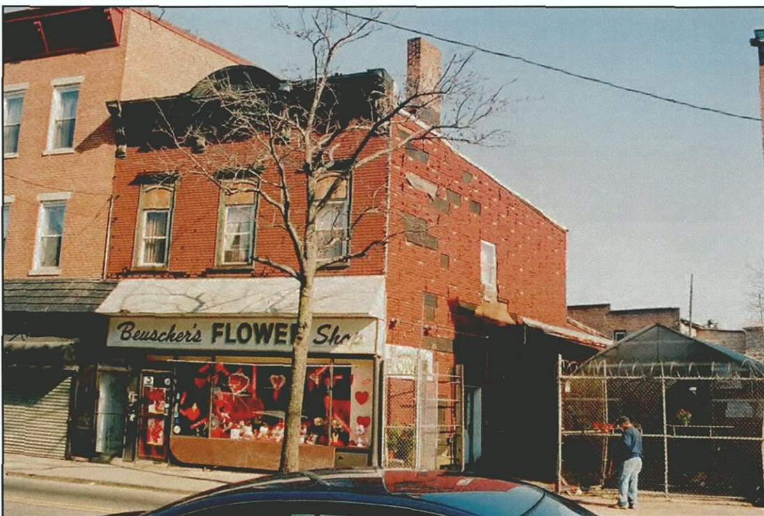
Photo 25 - 587 Bay Street (Survey No. 26) Looking Northeast
