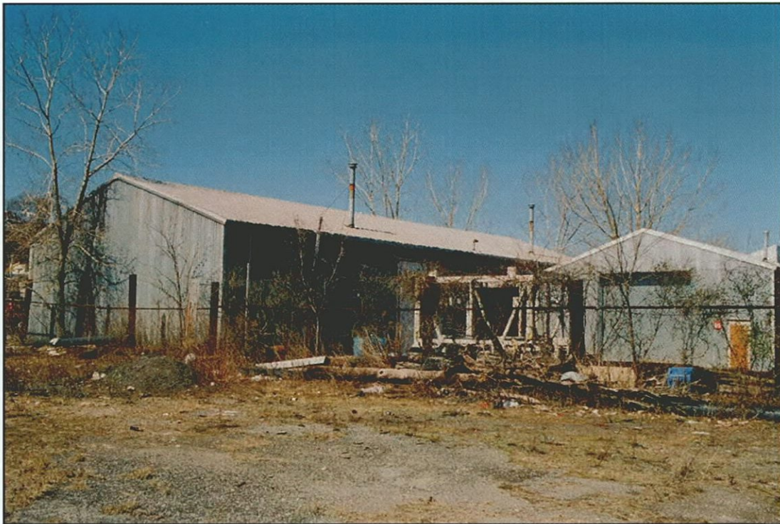
Photo 54 - Staten Island Ferry Buildings (Survey No. 63) Looking Northwest
