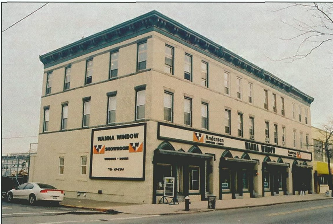
Photo 15 - 533-539 Bay Street (Survey No. 16) Looking Southeast
