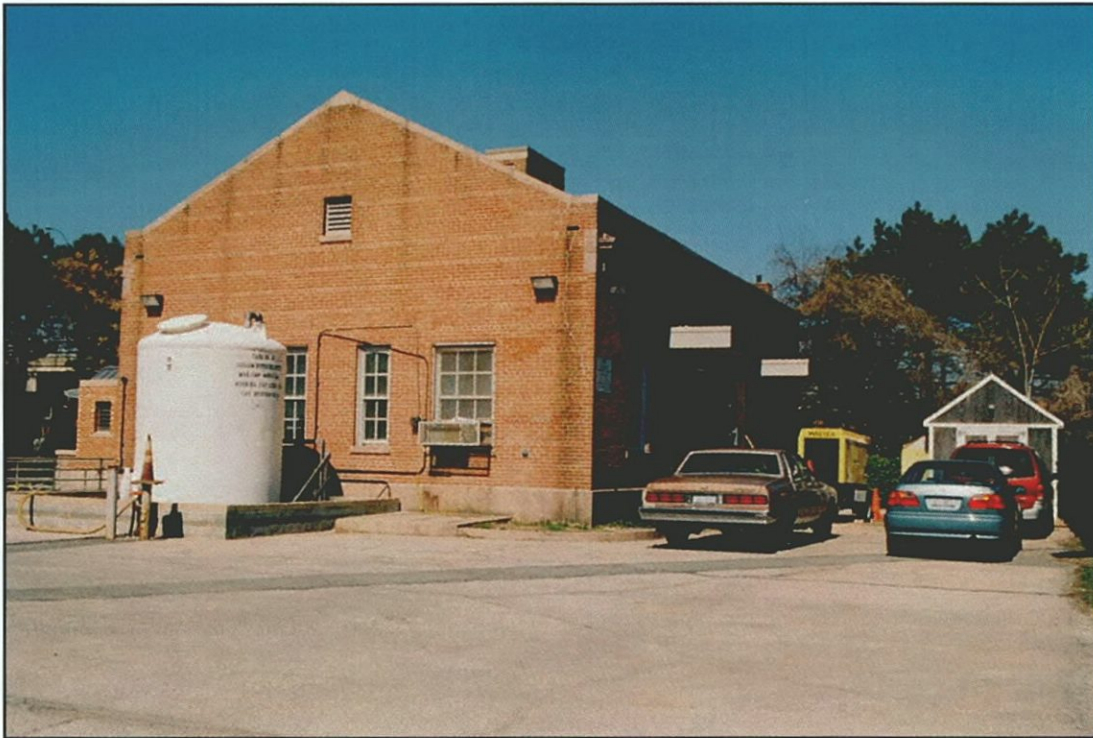
Photo 52 - Chlorination Building (Survey No. 61) Looking Northwest
