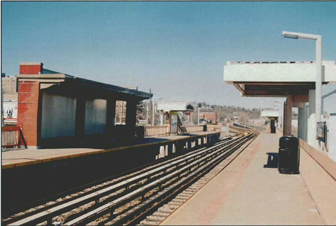
Photo 4 - Clifton Station, Staten Island Railway (Survey No. 5) Looking North
