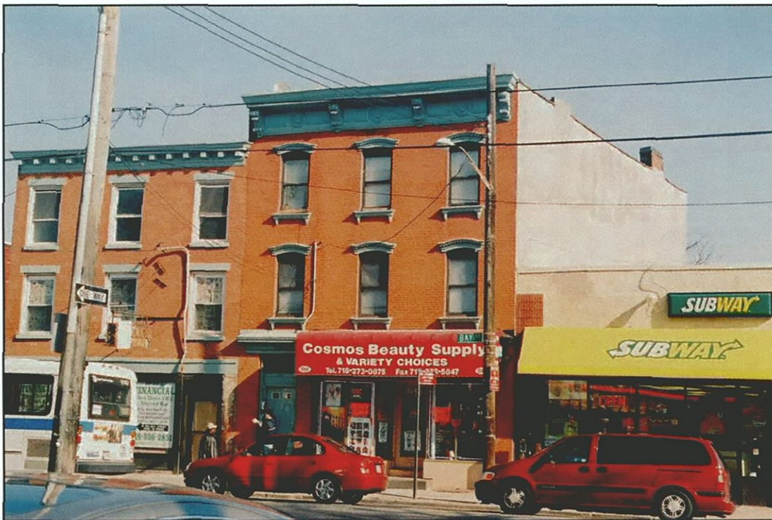
Photo 23 - 595 Bay Street (Survey No. 24) Looking Northeast
