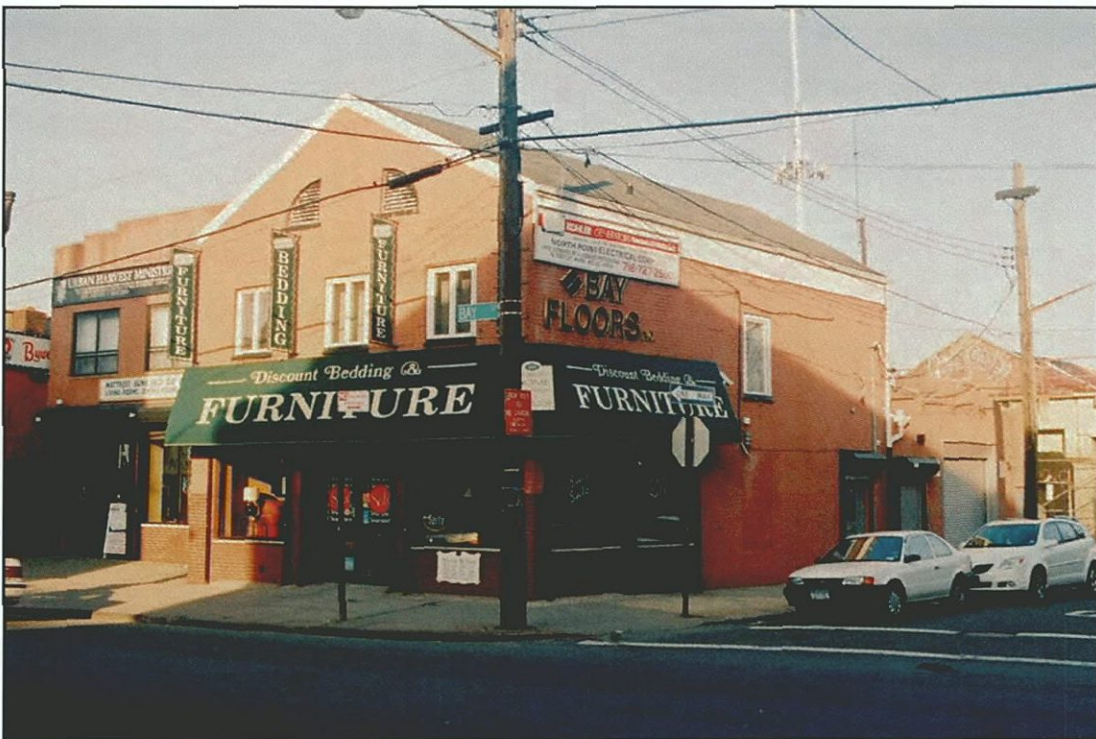
Photo 39 - 651 Bay Street (Survey No. 45) Looking Northeast
