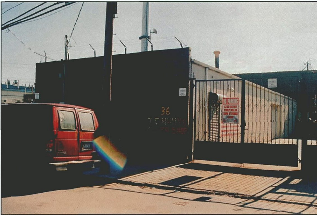
Photo 41 - 36 Canal Street (Survey No. 47) Looking Southeast
