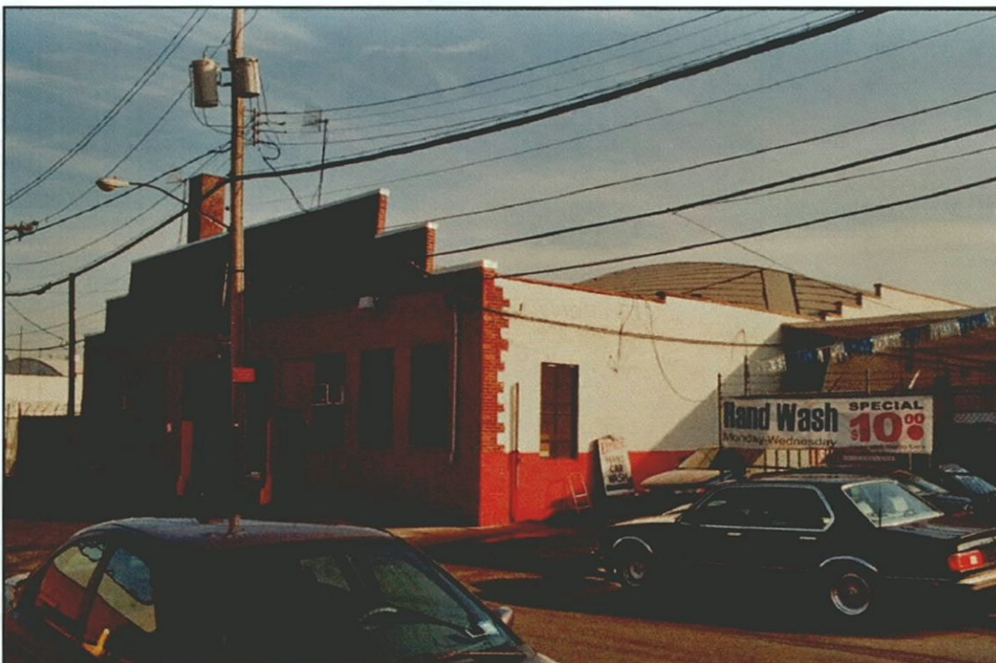
Photo 9 - 34 Wave Street (Survey No. 10) Looking Southeast
