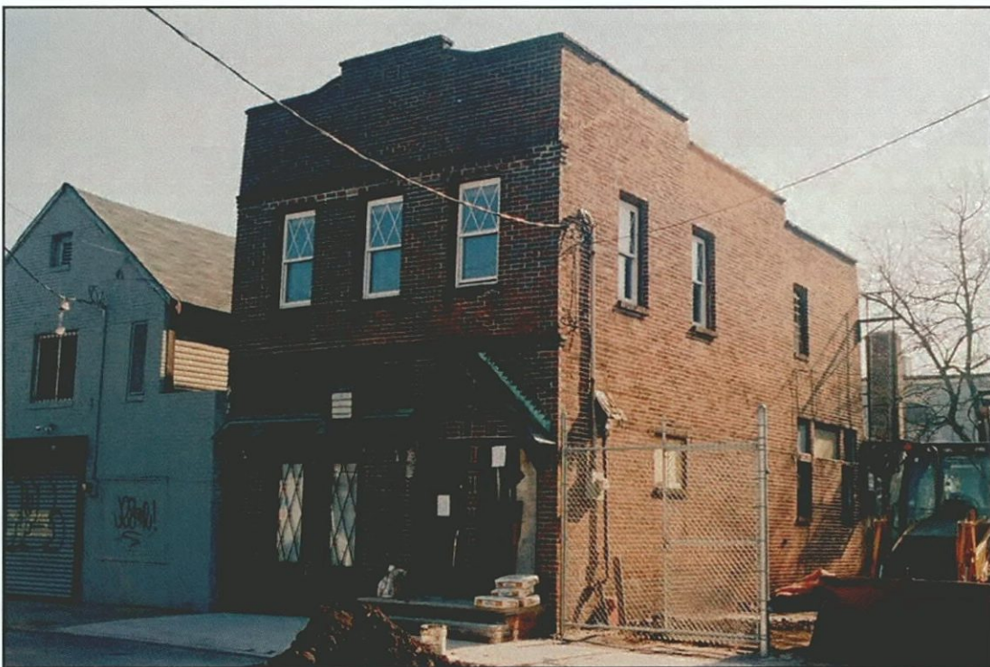
Photo 27 - 12 Cross Street (Survey No. 28) Looking Southeast
