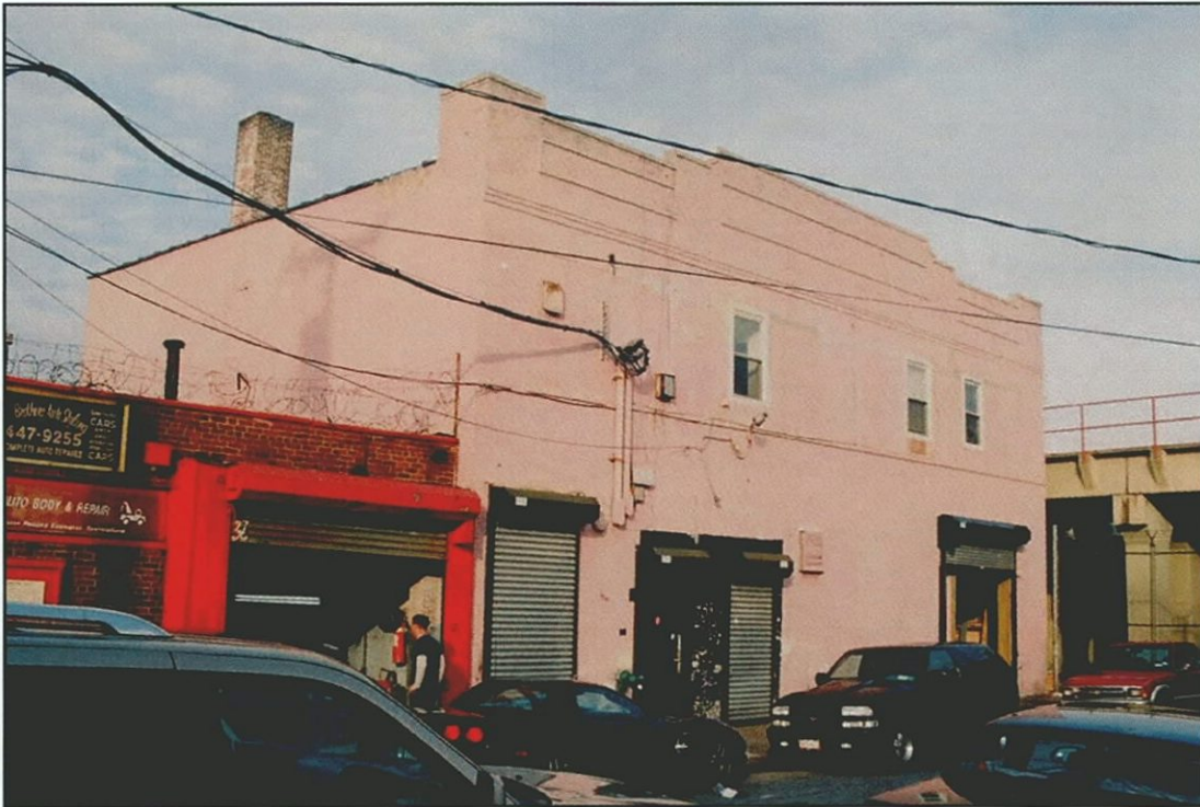
Photo 12 - 23 Sands Street (Survey No. 13) Looking Northeast
