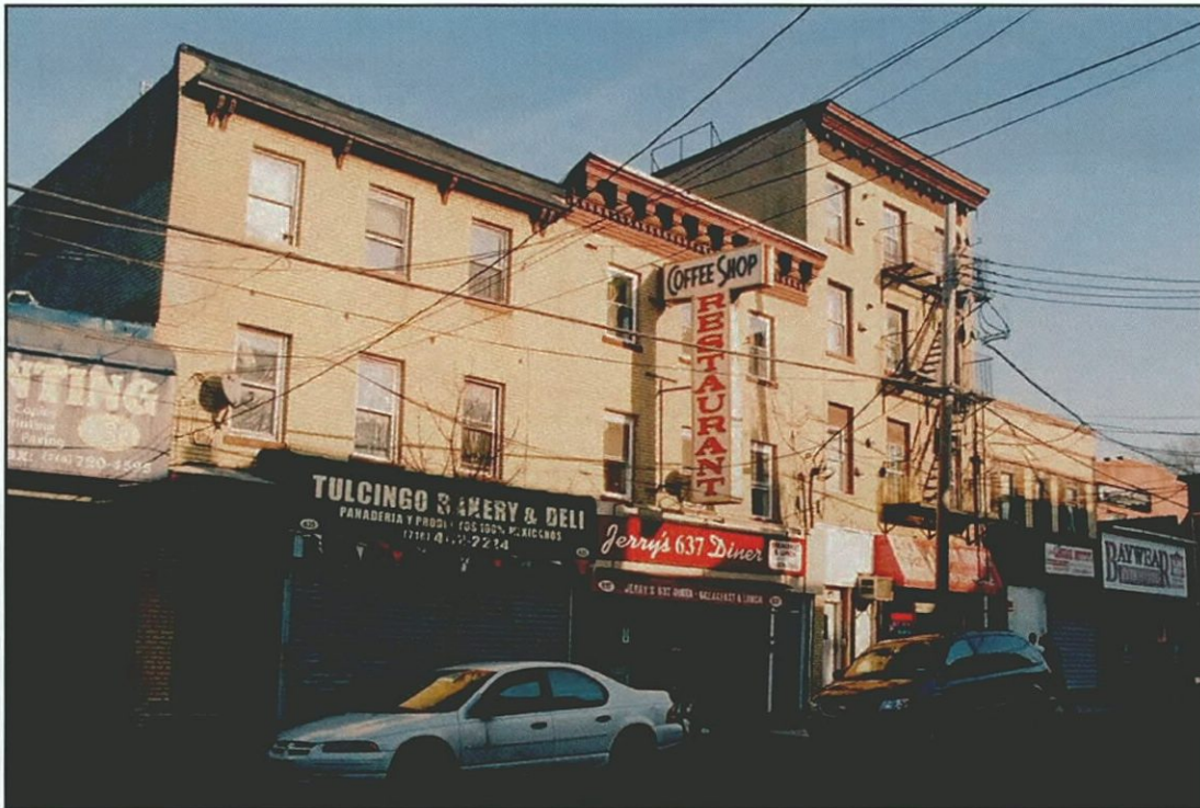
Photo 37 - 635 (Survey No. 39), 637(Survey No. 40), 639 (Survey No. 41), & 641 Bay Street (Survey No. 42) Looking Southeast
