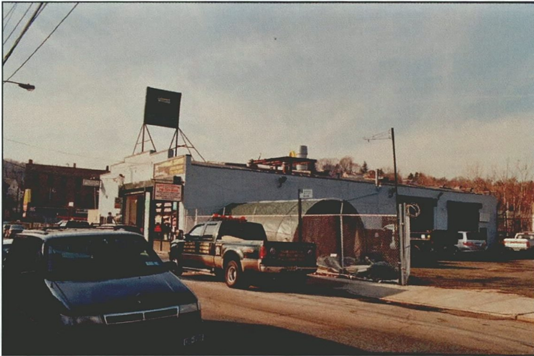
Photo 8 - 31 Wave Street (Survey No. 9) Looking Northwest
