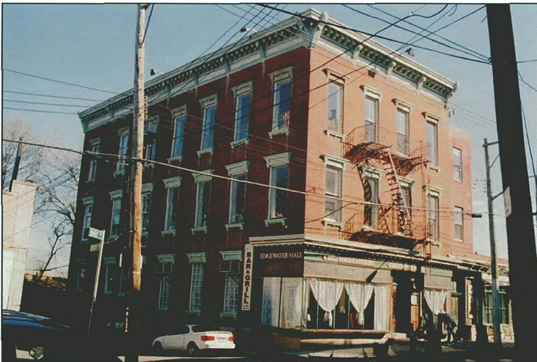
Photo 48 - 691 Bay Street (Survey No. 57) Looking Southeast
