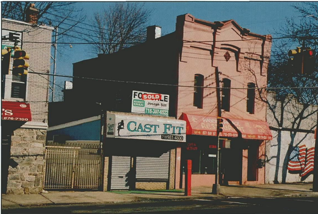
Photo 46 - 675 (Survey No. 54, left) & 677 Bay Street (Survey No. 55, right) Looking Southeast
