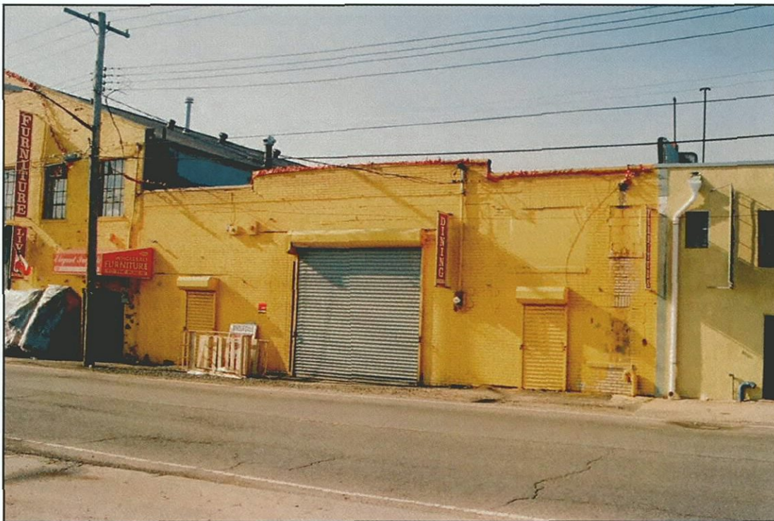
Photo 18 - 350 Front Street (Survey No. 19) Looking West
