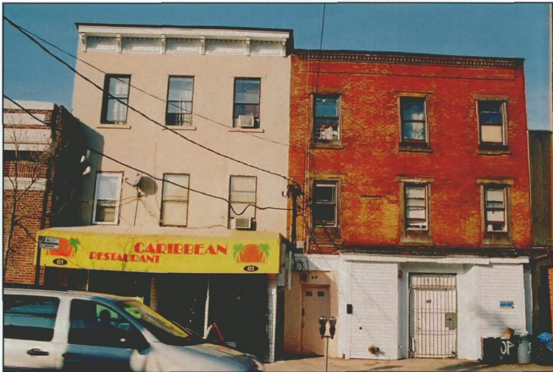
Photo 33 – 61 (Survey No. 34, left) and 59 (Survey No. 35, right) Canal Street Looking North
