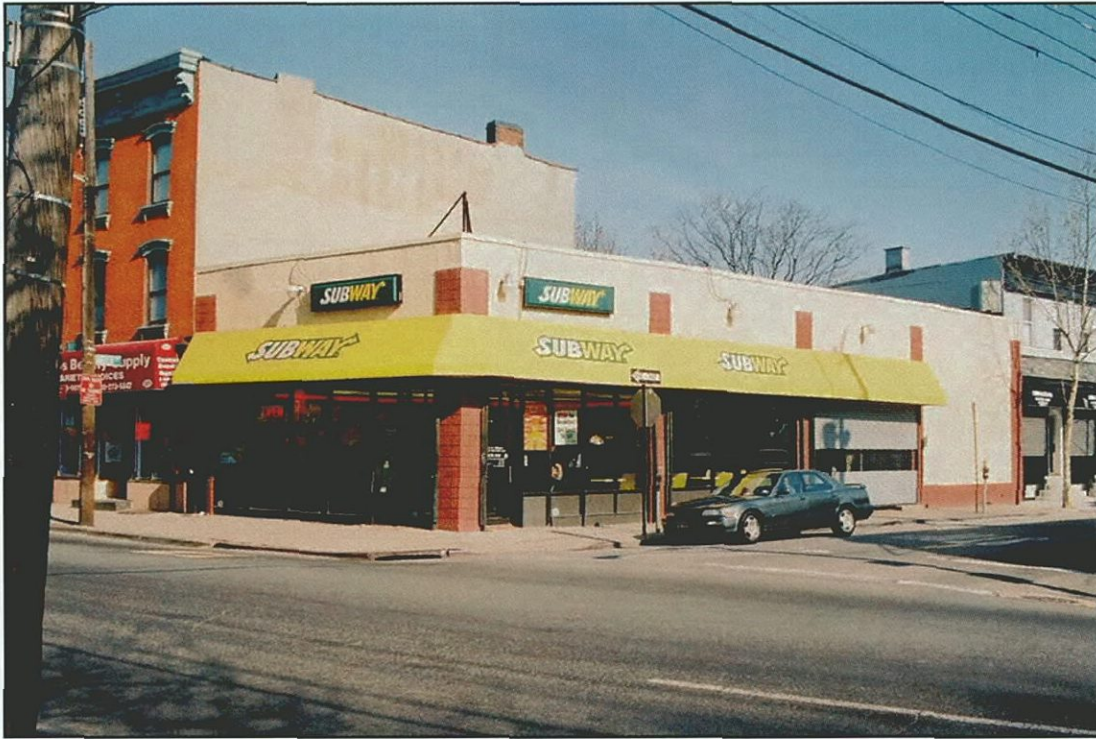
Photo 22 - 597 Bay Street (Survey No. 23) Looking Northeast
