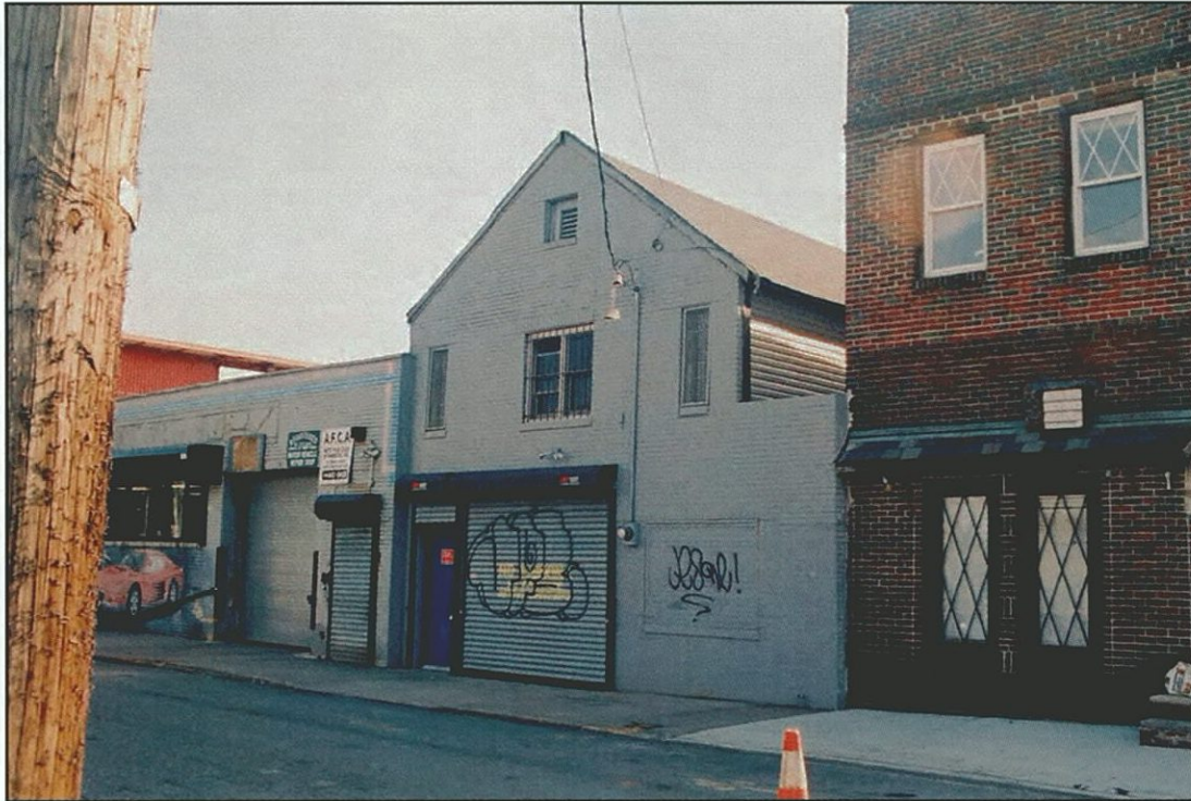
Photo 28 - 10 Cross Street (Survey No. 29) Looking Southeast
