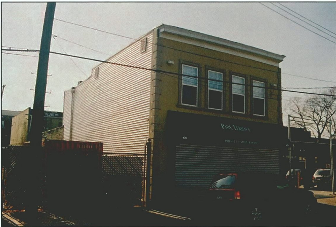
Photo 13 - 26 Water Street (Survey No. 14) Looking Southwest
