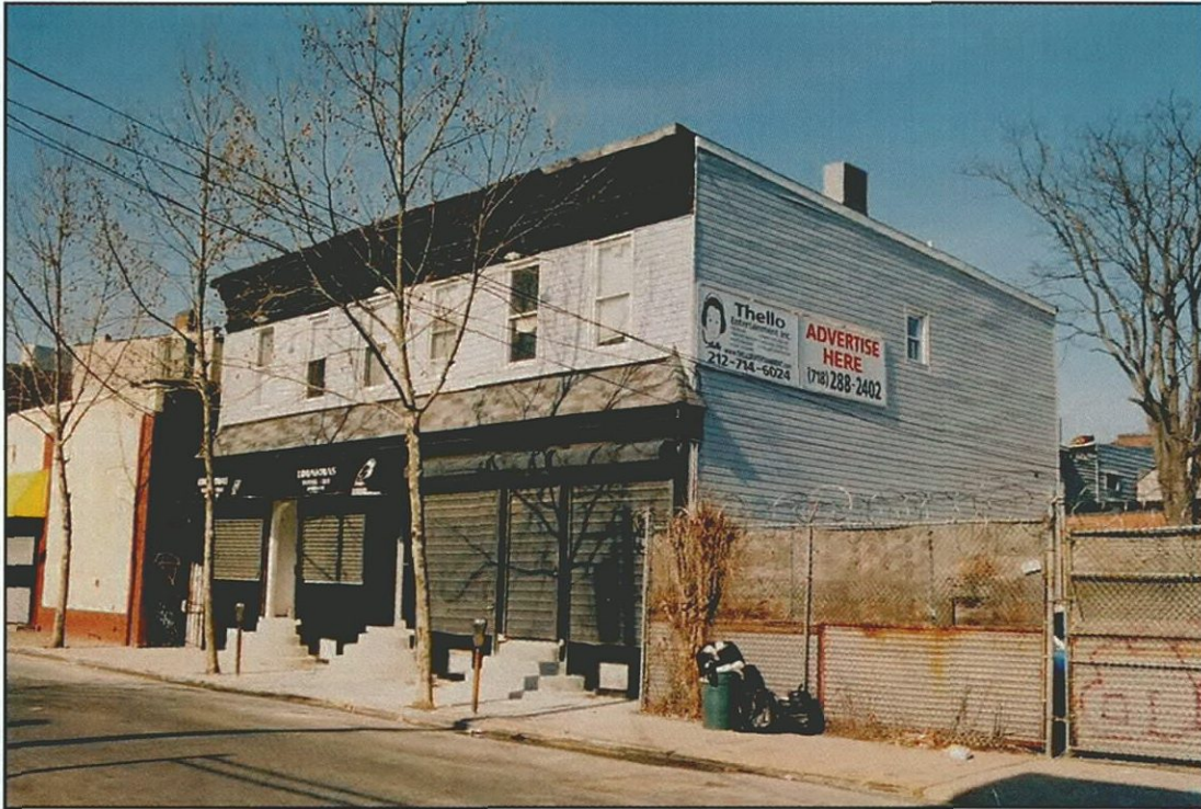
Photo 14 - 31 Water Street (Survey No. 15) Looking NW
