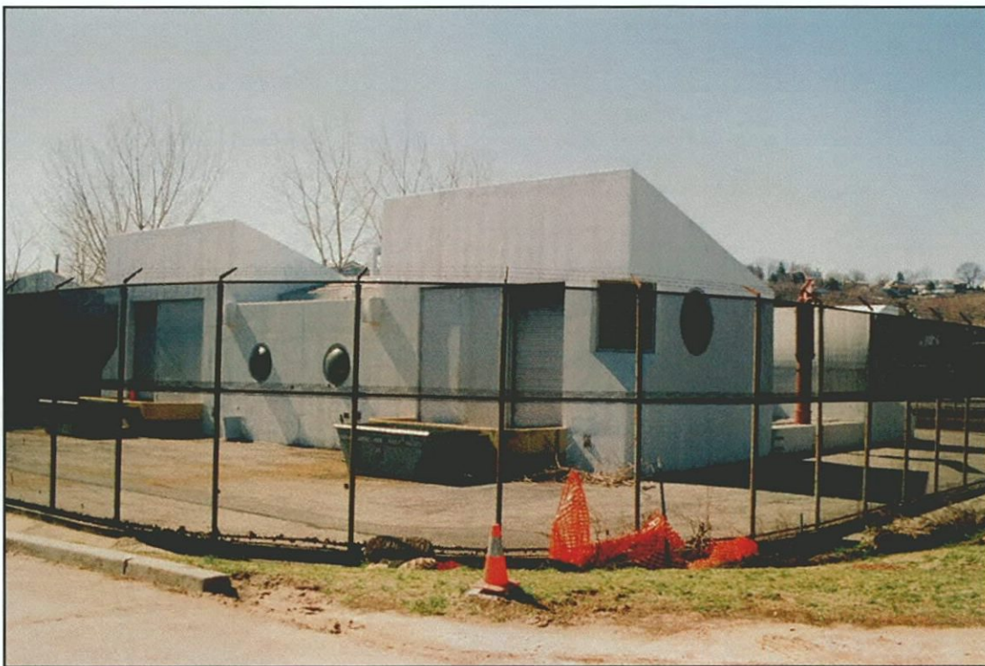
Photo 53 - Sewage Building (Survey No. 62) Looking Southwest
