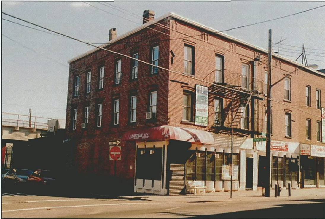
Photo 43 - 661 Bay Street (Survey No. 50) Looking Southeast
