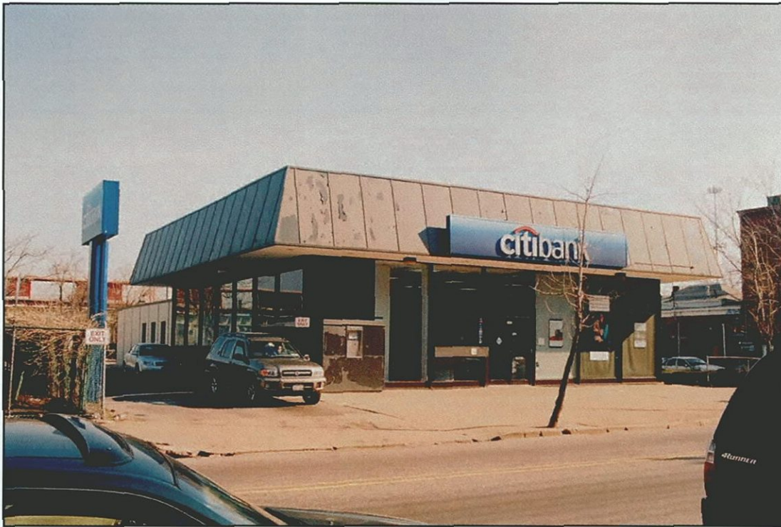
Photo 30 - 571 Bay Street (Survey No. 31) Looking Southeast
