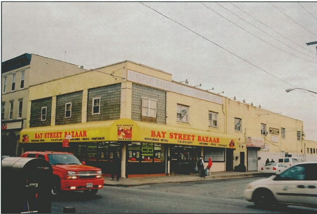
Photo 16 - 541 Bay Street (Survey No. 17) Looking Northeast
