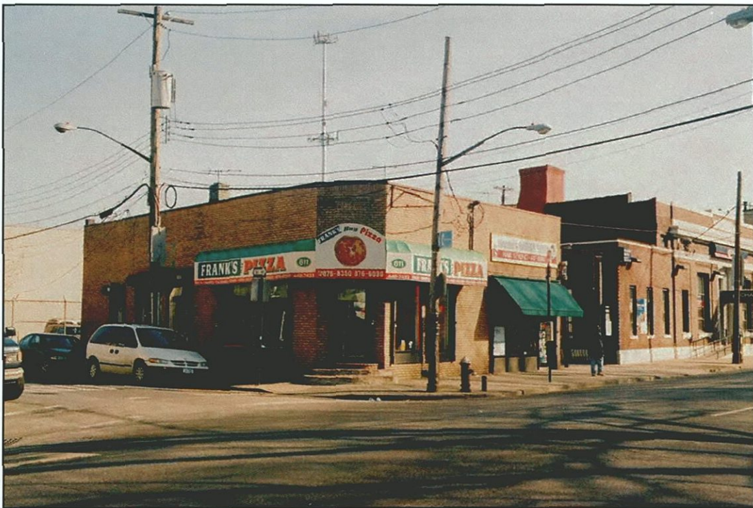
Photo 31 - 611 Bay Street (Survey No. 32) Looking Southeast
