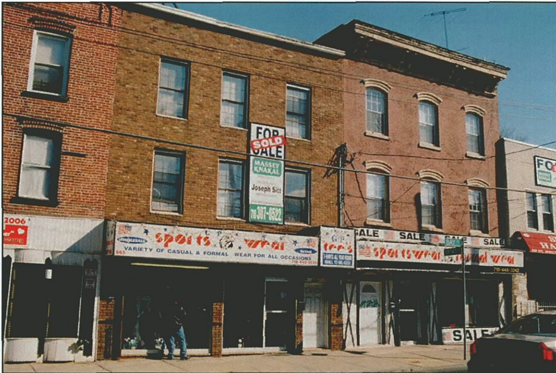
Photo 44 - 665 (Survey No. 51, left) & 669 Bay Street (Survey No. 52, right) Looking Southeast
