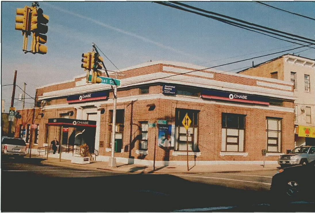
Photo 32 - 619 Bay Street (Survey No. 33) Looking Northeast
