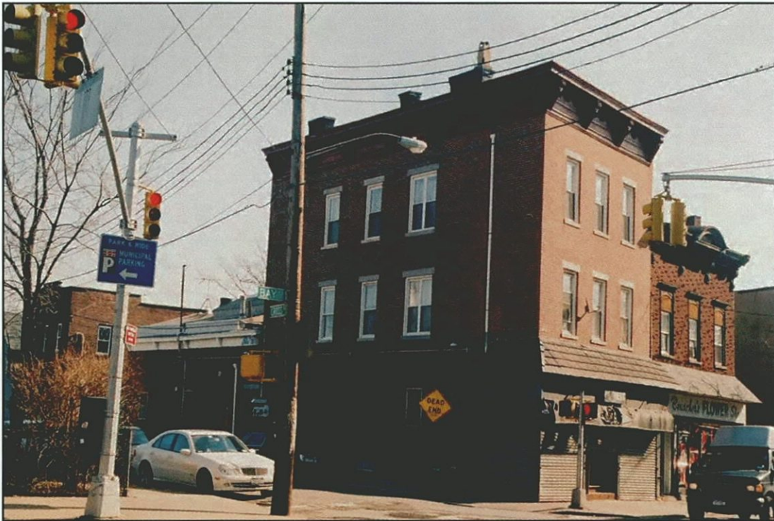
Photo 26 - 585 Bay Street (Survey No. 27) Looking Southeast
