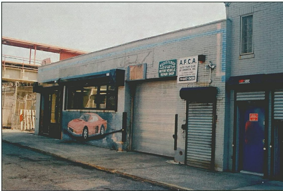
Photo 29 - 2 Cross Street (Survey No. 30) Looking Southeast
