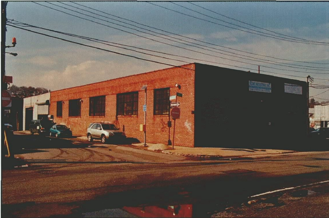
Photo 1: 326 Front Street, Survey No. 1 (foreground) and 15 Prospect Street, Survey No. 4 (background) Looking Northwest
