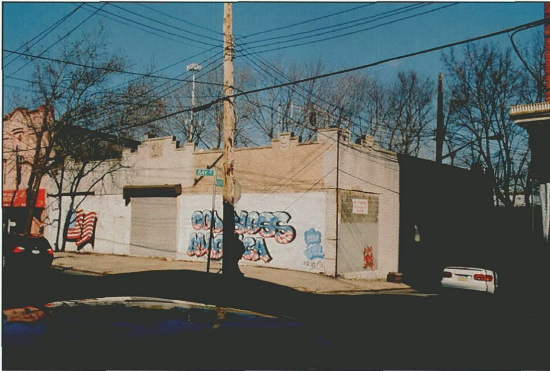
Photo 47 - 681 Bay Street (Survey No. 56) Looking Northeast
