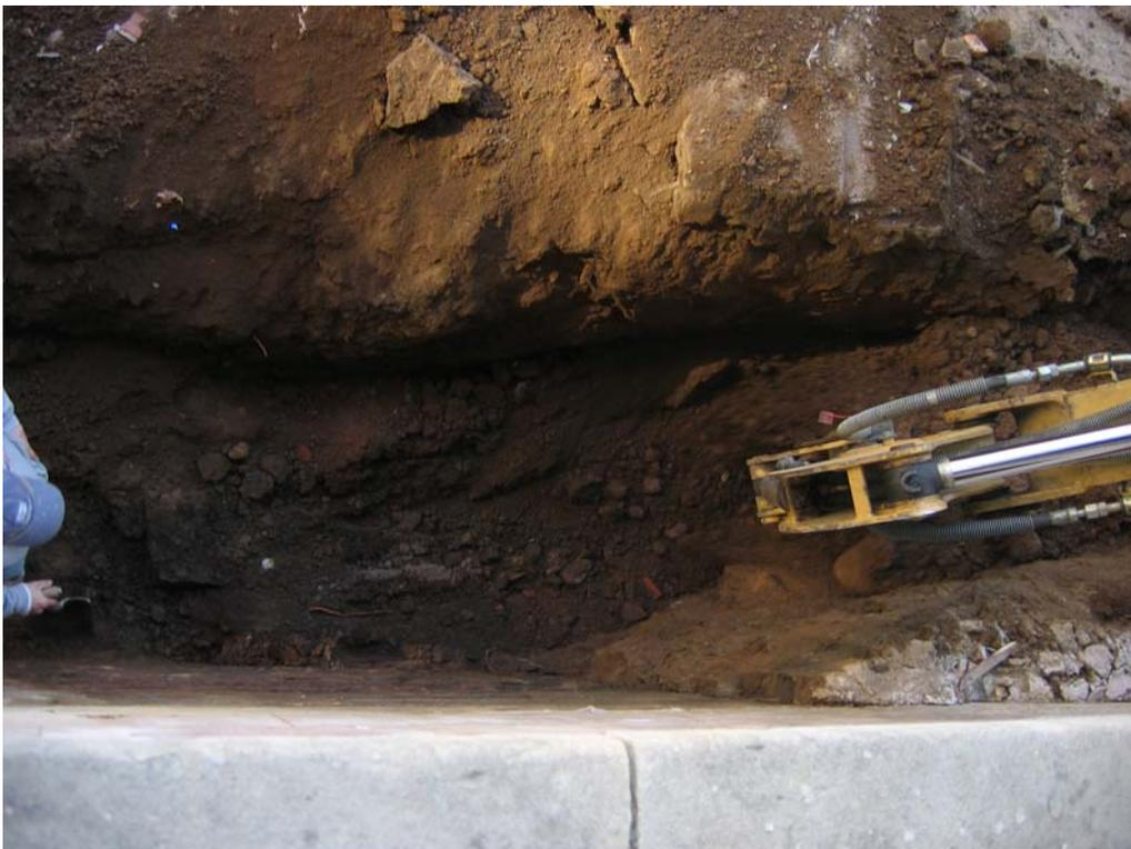
**Image 21: Excavation along the southwestern Pavilion foundation wall**
