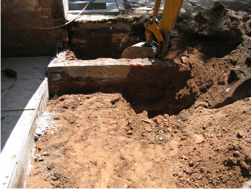
**Image 34: Staircase excavation showing original curbing and 19th century brick wall remains**
