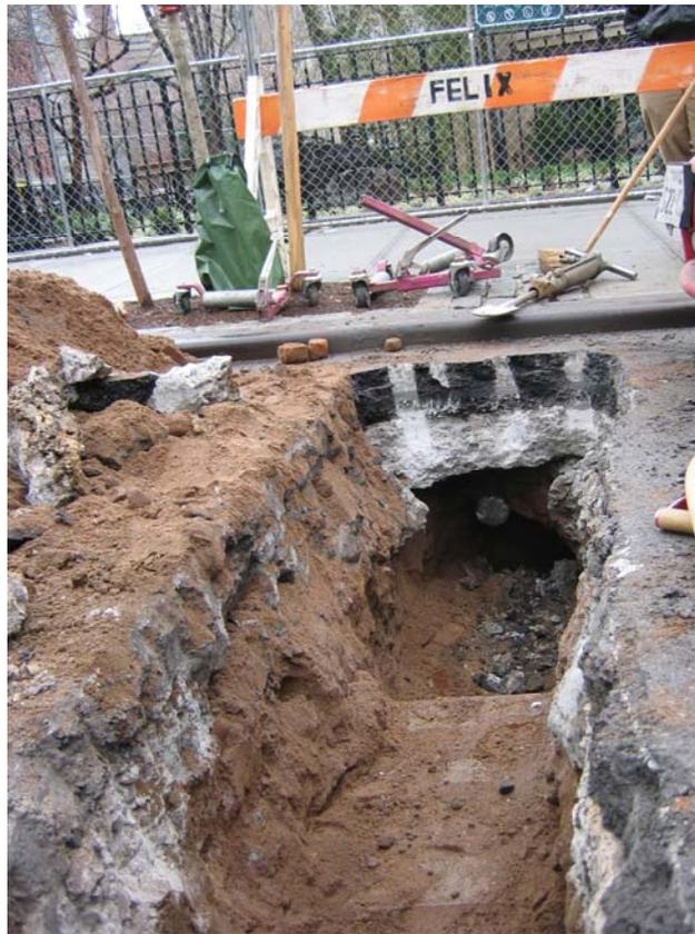
**Image 06: Completed gas line excavation trench**
