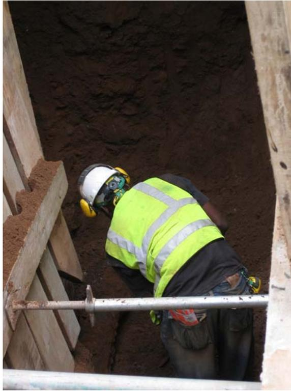
**Image 28: Excavation for water line - note the consistency of the modern deposited soil that was used to raise the level of the street to the current level.**
