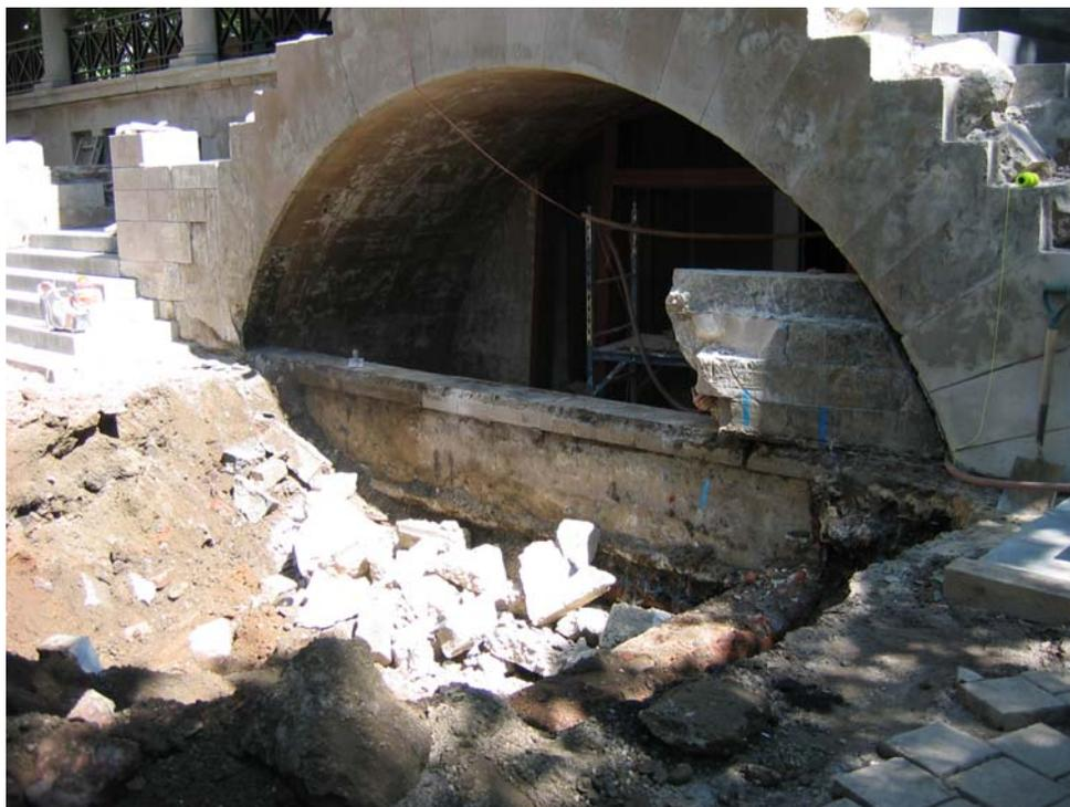
**Image 33: Staircase excavation showing original curbing and 19th century brick wall remains**
