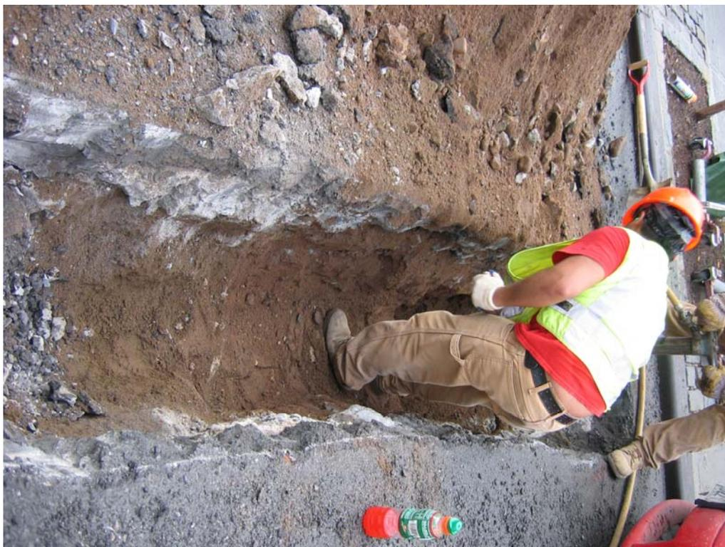
**Image 29: Excavating for the new gas line**
