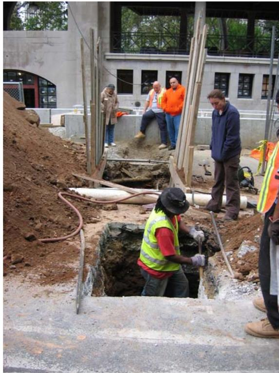
**Image 03: Excavation within the street for the water line**
