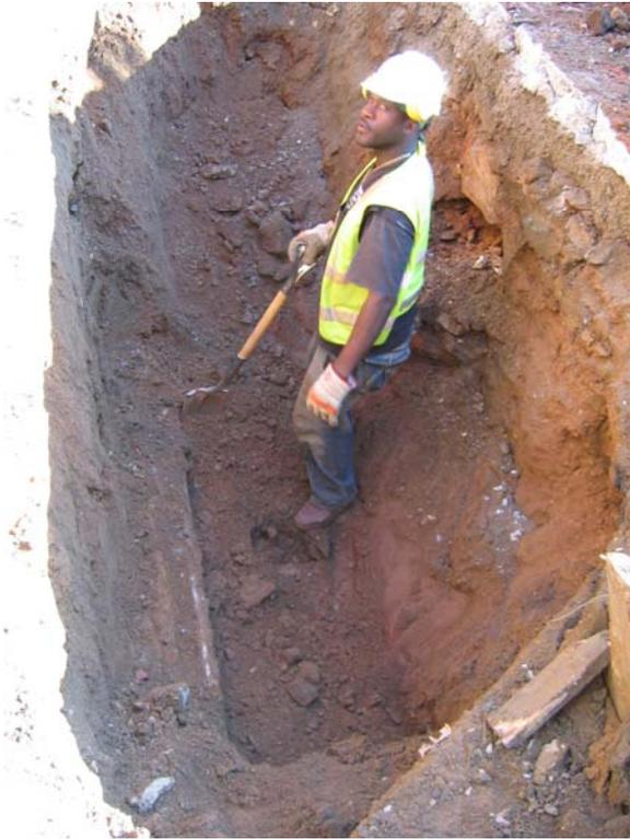
**Image 27: Excavation for water line**
