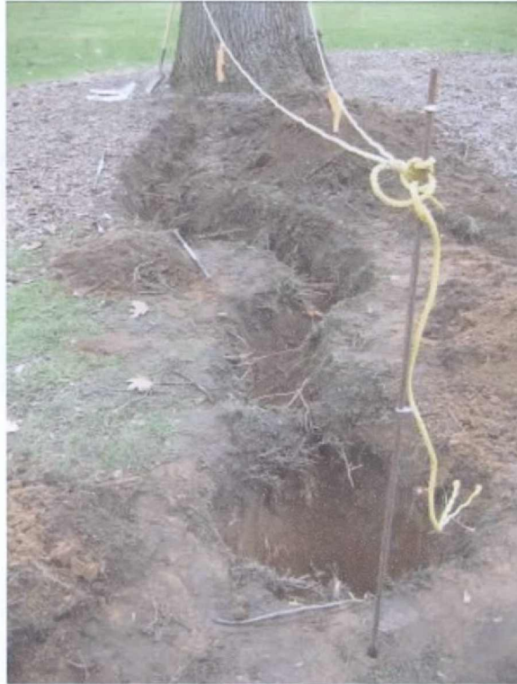
Photo 1 Completed trench at Tree 322 facing south.
