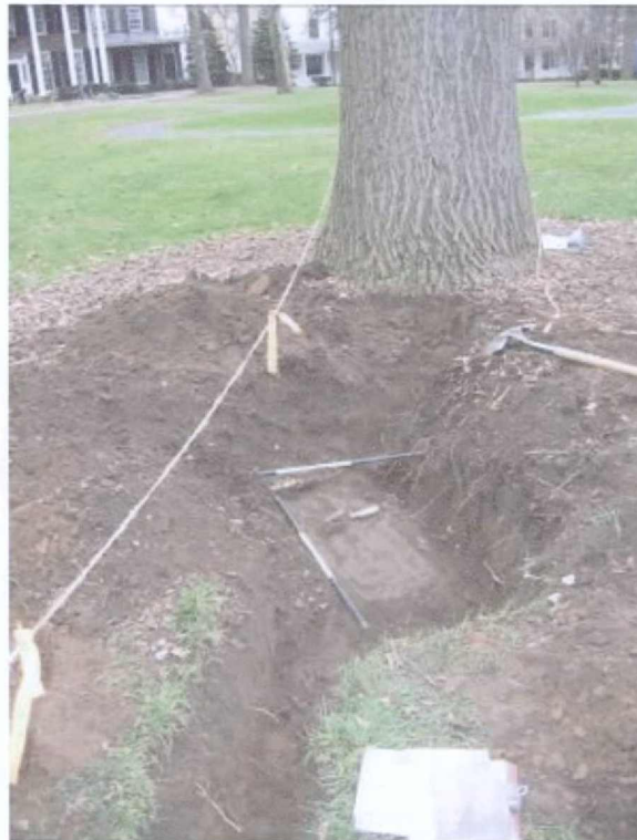
Photo 2 Completed trench at Tree 346 facing southeast showing the stone feature.
