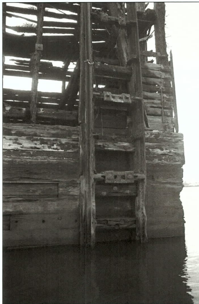
Figure 5-166. Starboard forward spud. Note trucks. View to the northwest (port).
