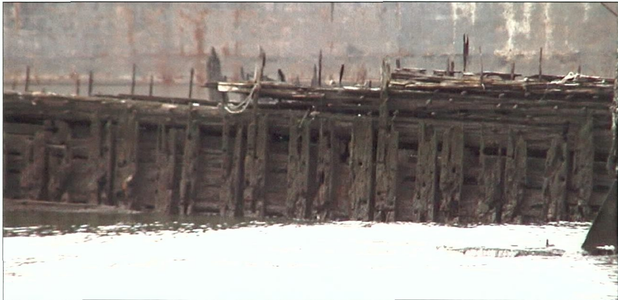
Figure 6-105. Port side, amidships, showing arrangement of futtocks and frames. View to the southwest.
