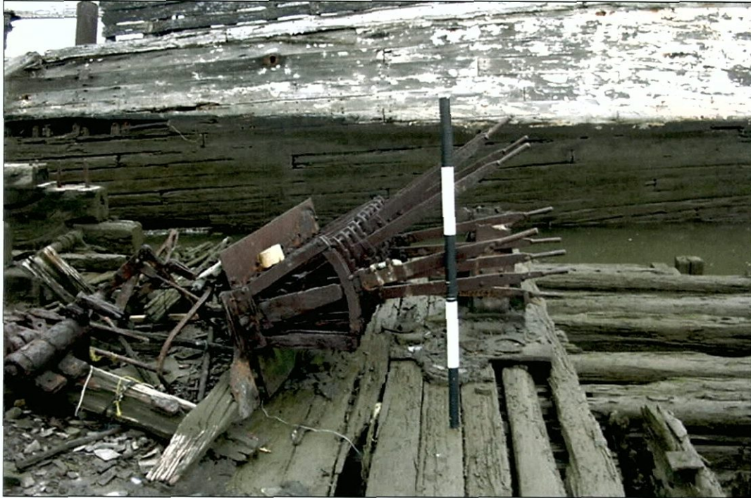
Figure 4-60. Hoisting drum control box. View to the east (port).
