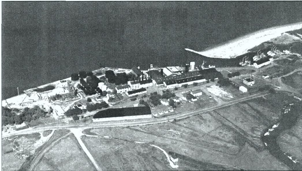
Figure 7-14. Port Monmouth, New Jersey plant, shown in the mid-1950s. This plant would be the homeport of the Smith Company for nearly the entire 60+ years of its existence (photo courtesy of Bob Cabbage).
