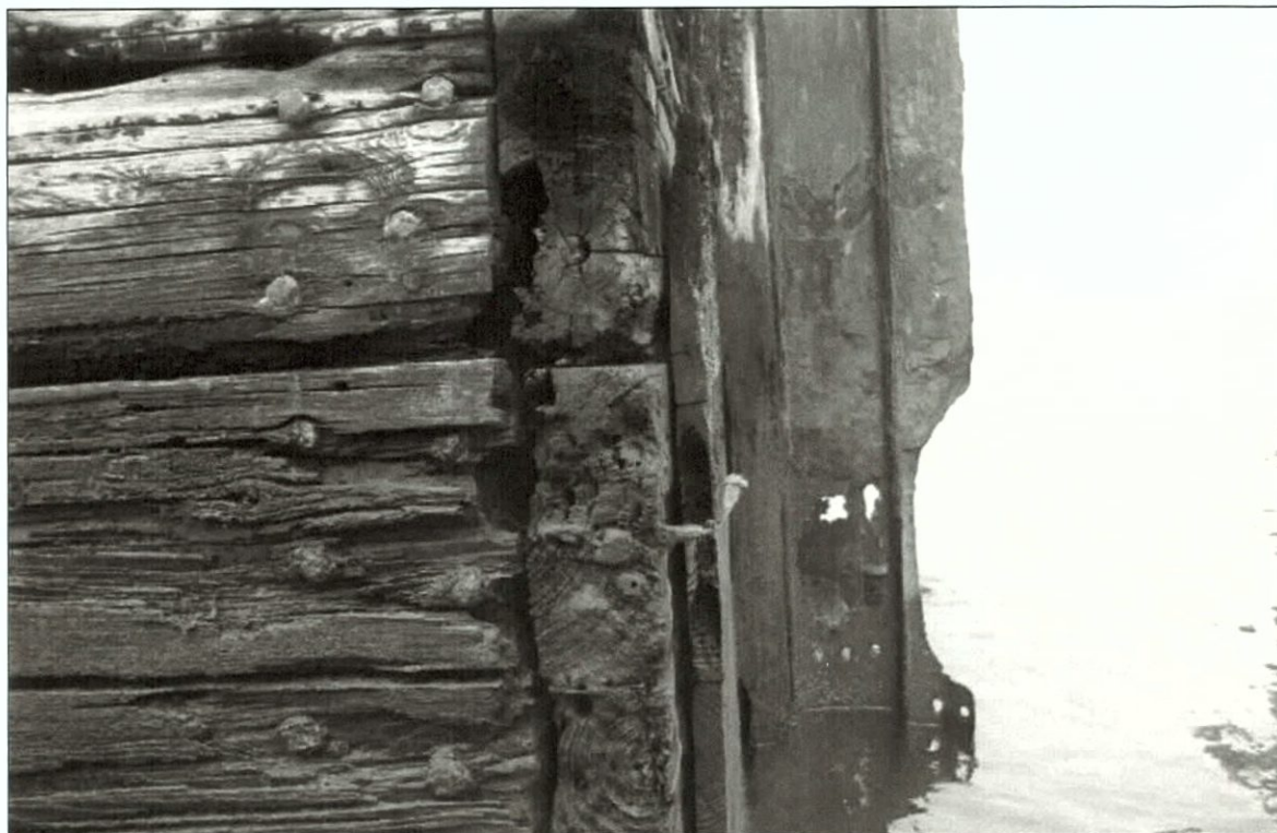
Figure 5-28. Outer planking of pontoon.
