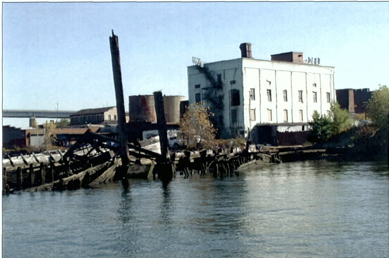
Figure 4-24. V36 starboard side, looking forward. View to the south.
