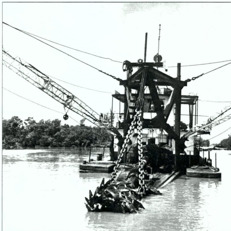
Figure 4-07. Dredge boom, showing cutterhead. Note also the cable system (photo courtesy of the Florida Photographic Collection).
