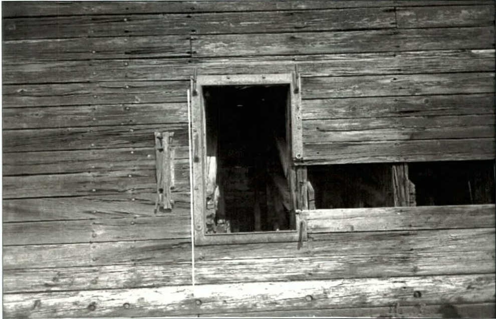
Figure 5-136. Port wing central hatch. View to the west (port).
