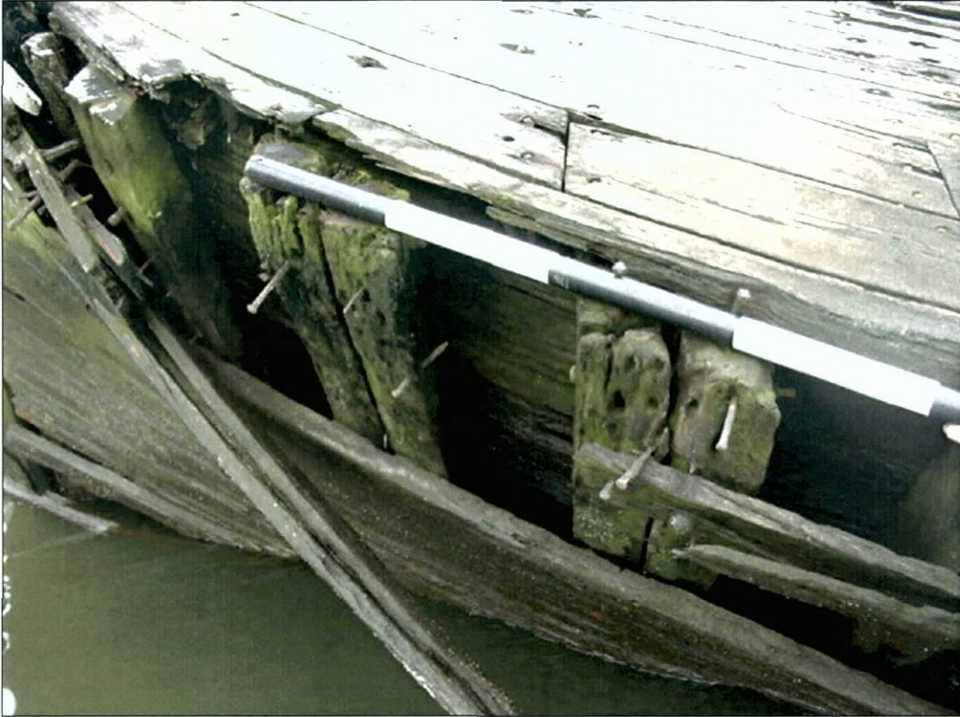
Figure 7-53. Close-up of canted frames. Port bow, looking west.
