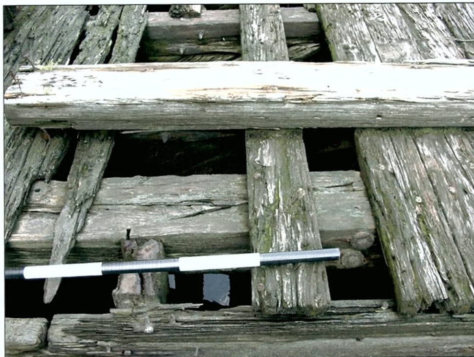
Figure 5-82. Bilge block stringer detail, aft port. Note placement of stringers over deck beams. View to the north (forward).
