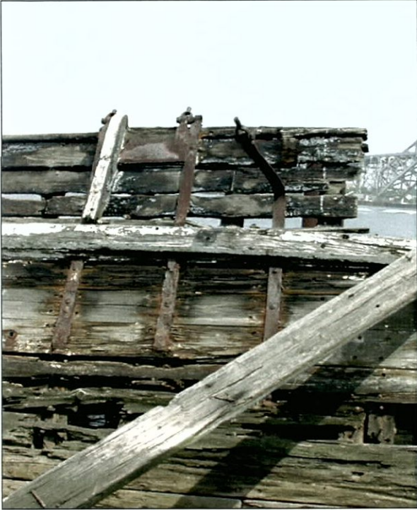
Figure 7-88. Detail of starboard chain plates.
