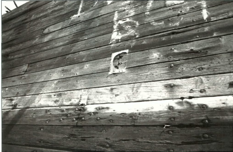
Figure 5-177. Port wing outer surface, showing carriage bolts at bulkhead (right) and the inter-frame plank joint (reinforced by a chock on the interior of the vessel). View to the northeast (starboard forward).
