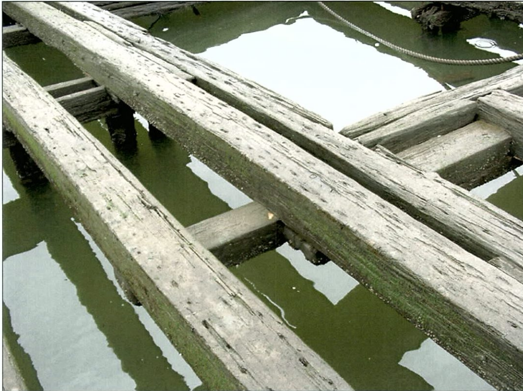
Figure 6-90. Detail of hatch beams. View to the northwest.
