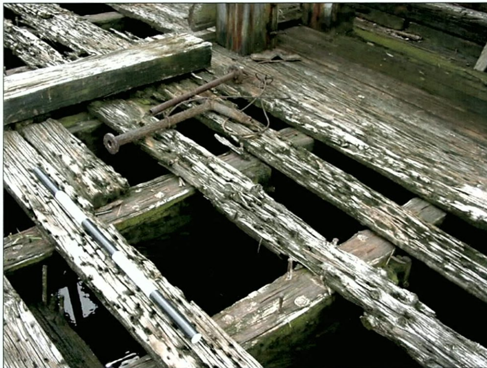
Figure 5-42. Detail of exposed deck beams. View to the southeast (port).
