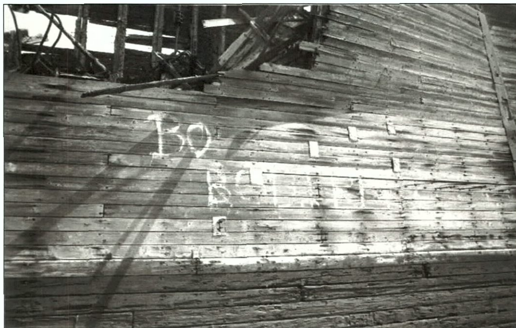
Figure 5-127. Detail of port wing, aft corner. Note change in plank sided dimension similar to the inner wing wall. View to the east (starboard).
