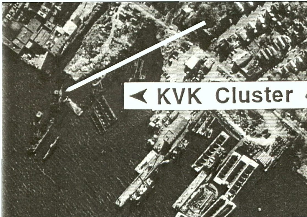
Figure 4-21. 1974 vertical aerial photo of Cluster 4, showing V36 in its current location.
