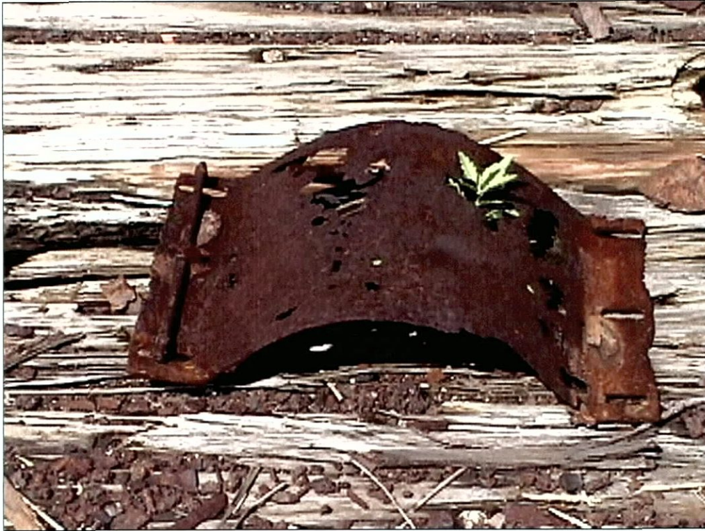
Figure 5-179. Iron or steel vent cover.
