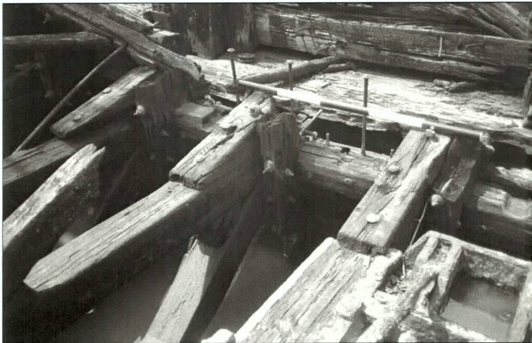
Figure 5-62. Northern exposed end of V1 showing Truss 7 at main deck.
