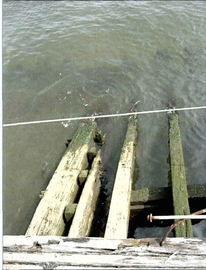
Figure 7-66. Detail of top of aft bulkhead showing support beams and stanchion tops, looking port (east).
