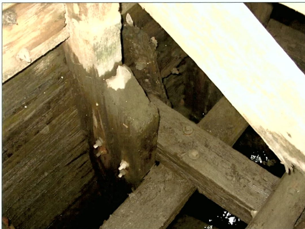
Figure 5-56. Side frame detail just above main deck, port wing. Note termination of inner futtock.
