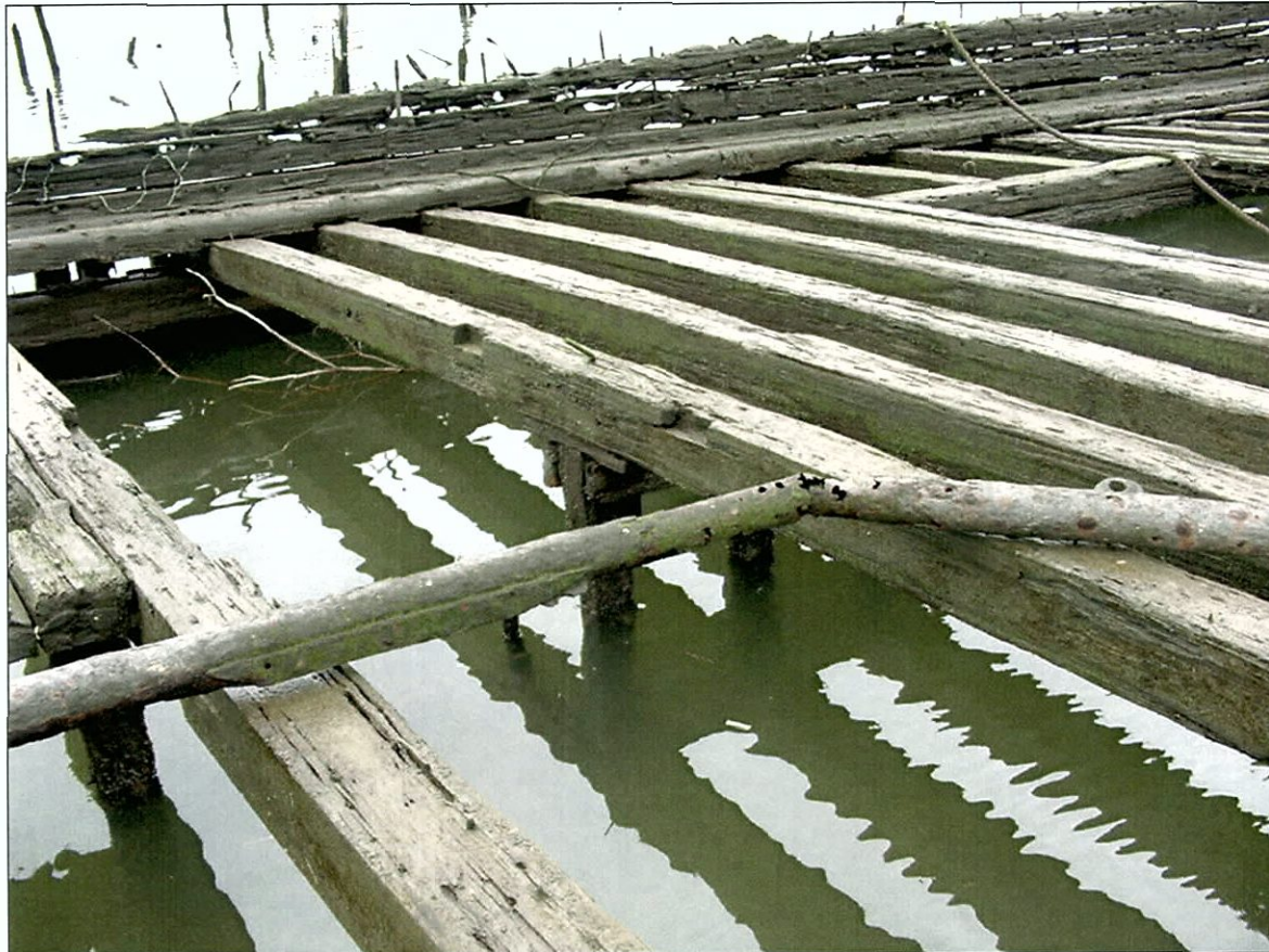
Figure 6-86. Cargo deck midships. View to the west.
