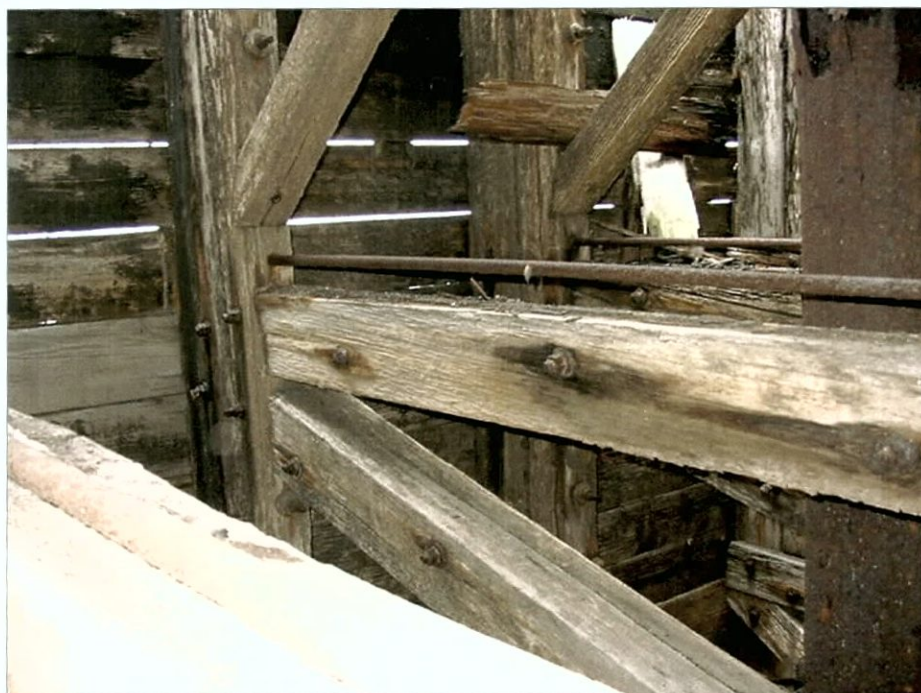
Figure 5-112. View of horizontal truss beam tie rod and joint, outer wall of starboard wing. This joint is directly opposite that shown in Figures 5-109 and Figure 5-110. View to the northwest (forward).
