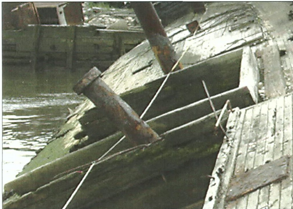
Figure 7-92. Fish Hawk from port side looking forward (south). Note remaining vent stack and main mast.
