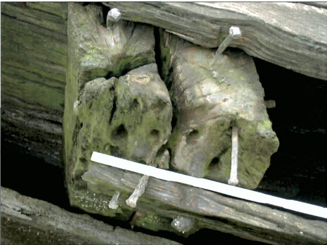
Figure 7-54. Close-up of the fifth canted frame.
