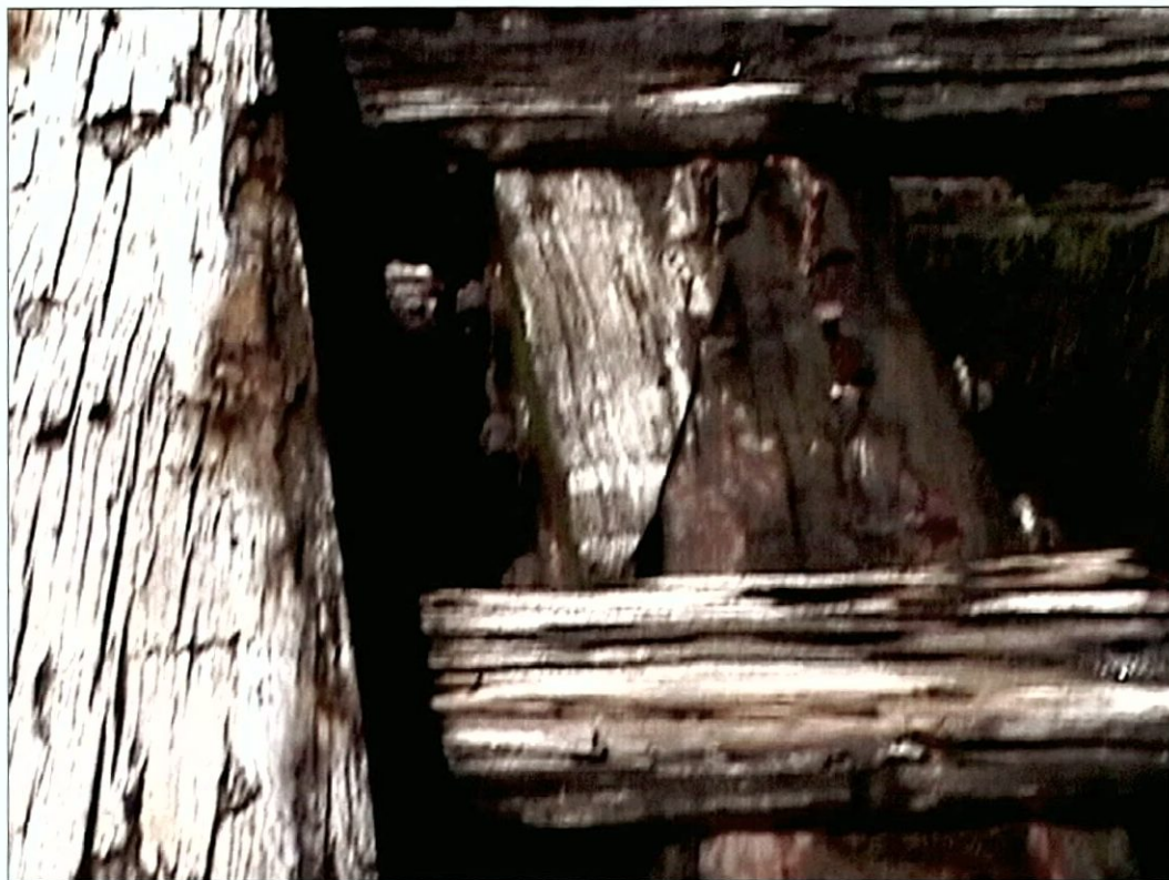
Figure 5-39. Top end log scarp joint, fastened with four bolts. View to the west (port).
