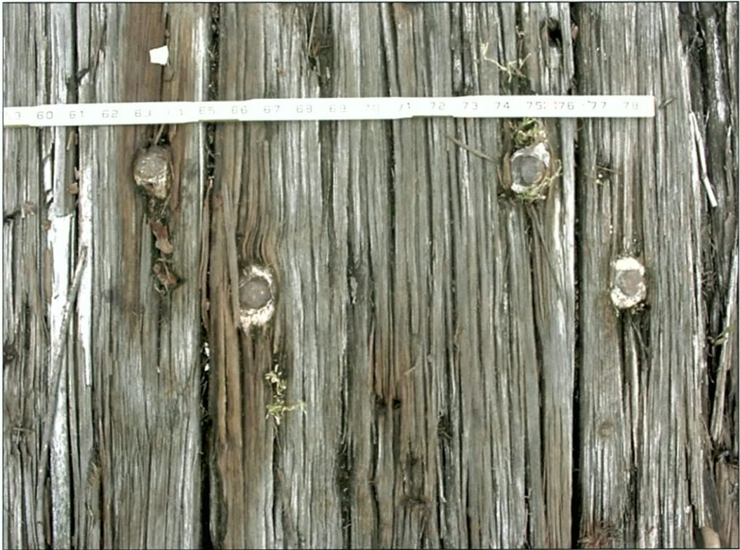
Figure 5-77. Deck plank fastener pattern detail.
