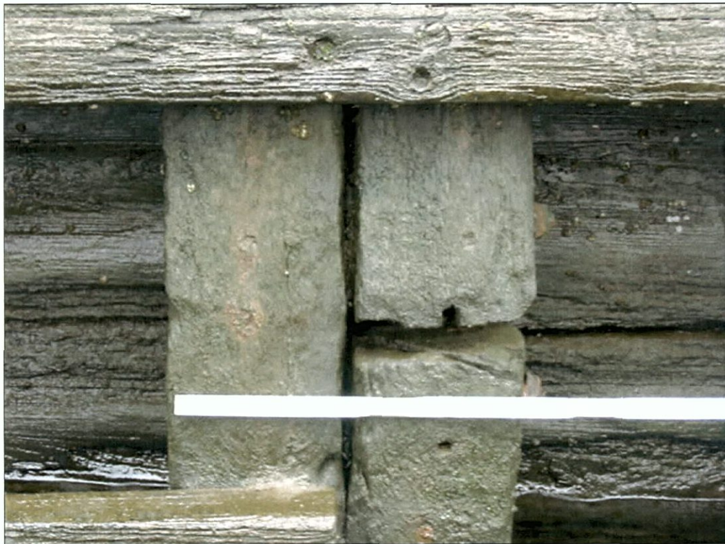
Figure 7-50. Close-up of exposed framing in Figure 7-49. Starboard side, looking east.
