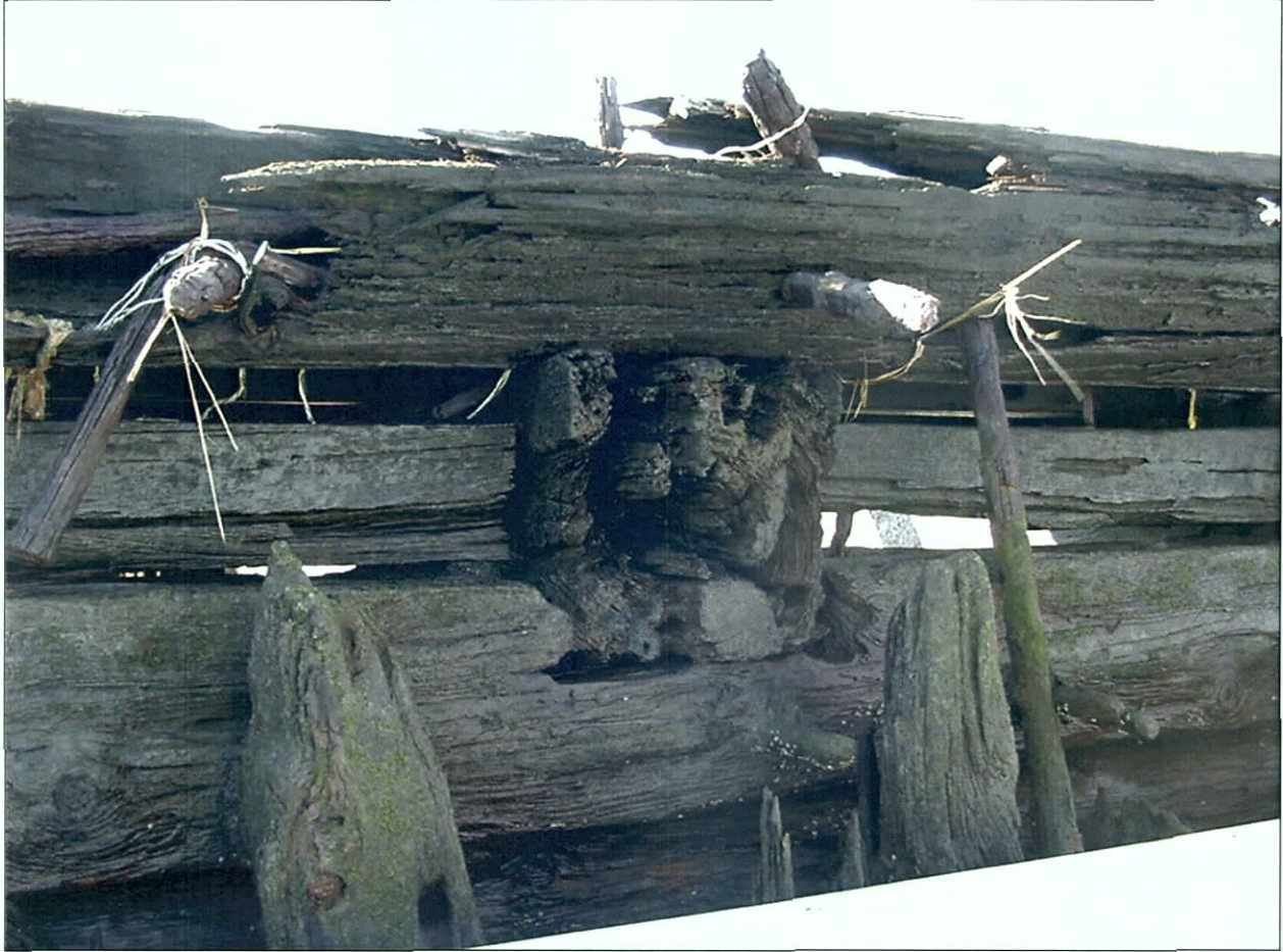
Figure 6-87. Starboard midships showing cargo deck beams in relation to clamp and frames. View to the south.
