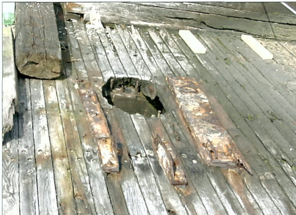
Figure 7-72. Close-up of deck planking along forward edge of cargo hatch coaming. Note king planks at right and slight varying in size of planking.
