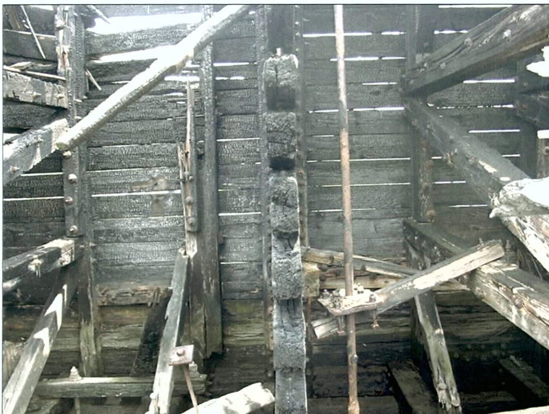
Figure 5-46. Bulkhead timbers. View to the east (starboard).
