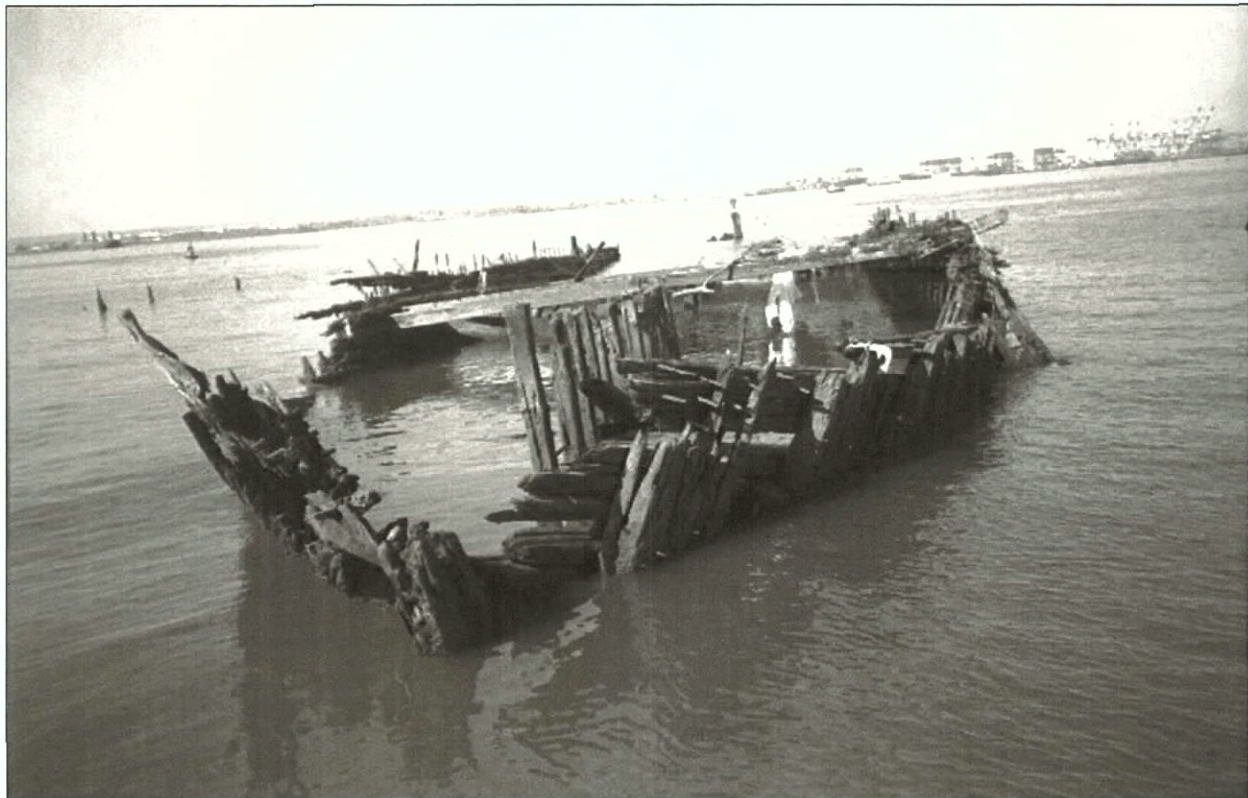
Figure 6-80. General view to the north.
