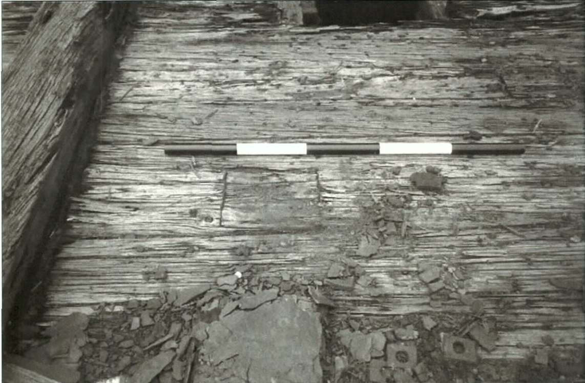
Figure 5-172. Small plug repair on main deck.
