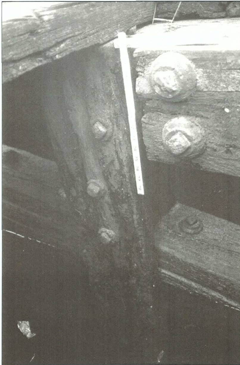
Figure 5-173. Truss and stanchion showing 1-inch and 5/8-inch bolts.
