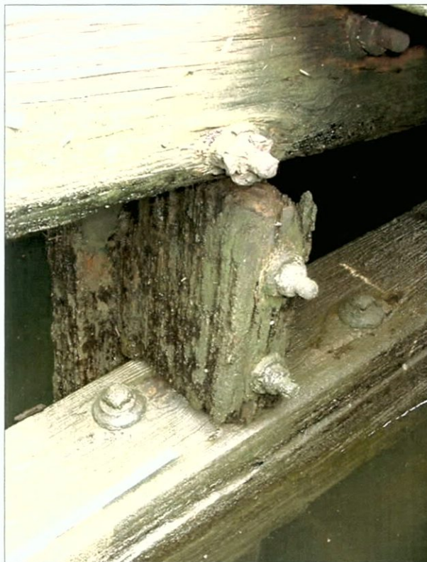
Figure 5-51. Example of chock between hull structural members.
