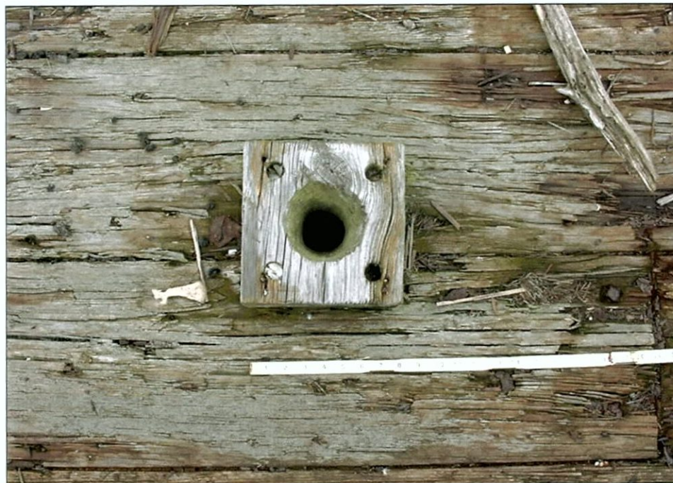
Figure 5-87. Deck fitting with tapered hole.
