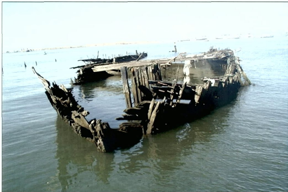
Figure 6-85. Cargo deck. View to the north.
