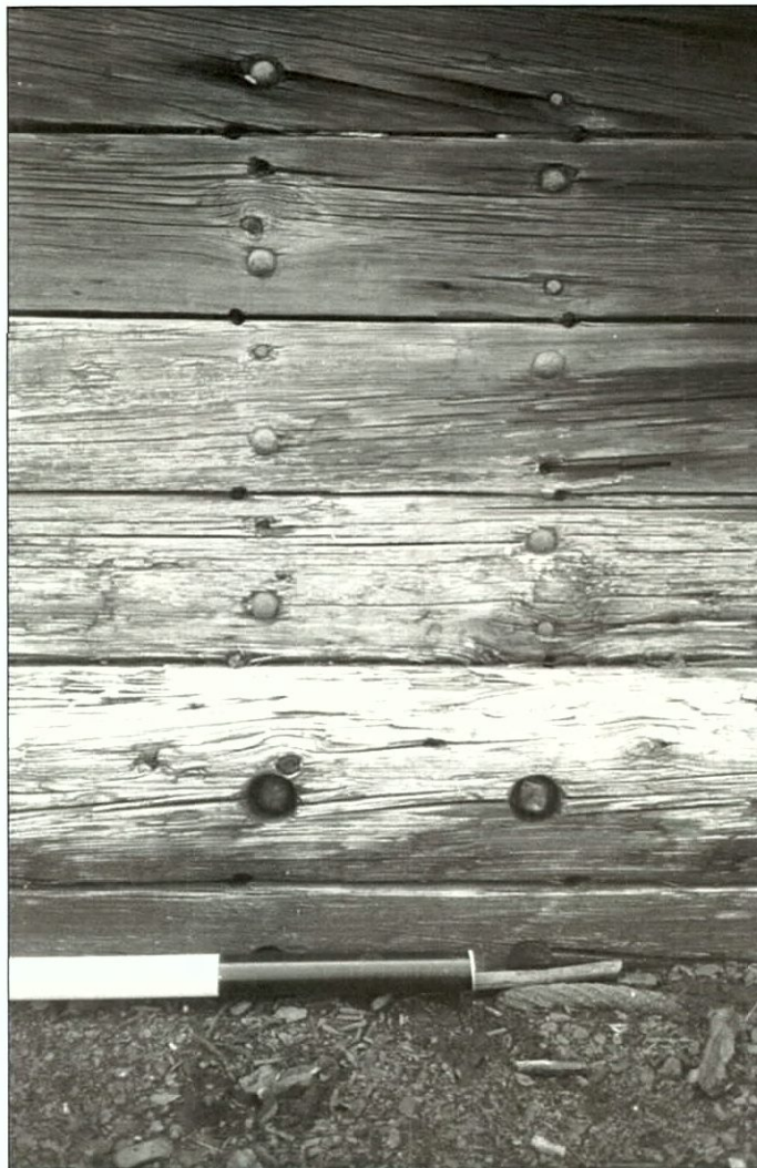
Figure 5-174. Port wing chine logs and outer planking. Note countersunk bolts and carriage bolts. View to the west (port).
