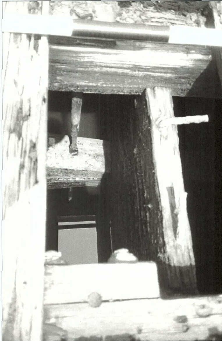
Figure 5-49. Top of longitudinal bulkhead showing exposed fasteners.
