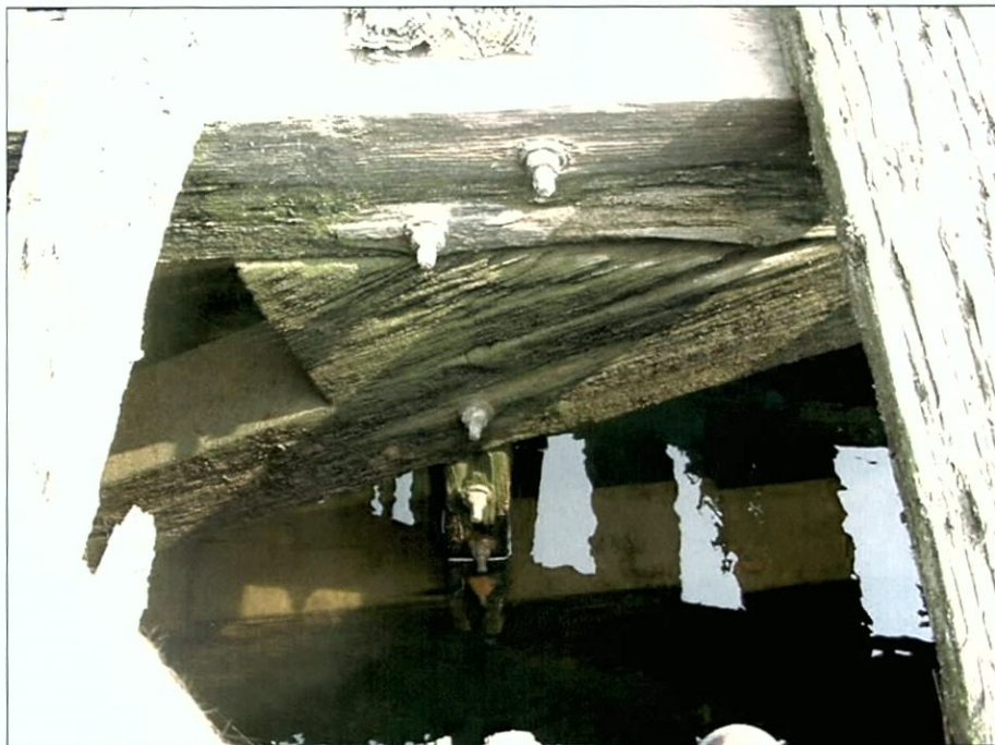
Figure 5-60. Truss 6 at main deck beam. Note triangular chock between truss and beam, and narrow vertical chock below truss opposite stanchion. View to the north (forward).
