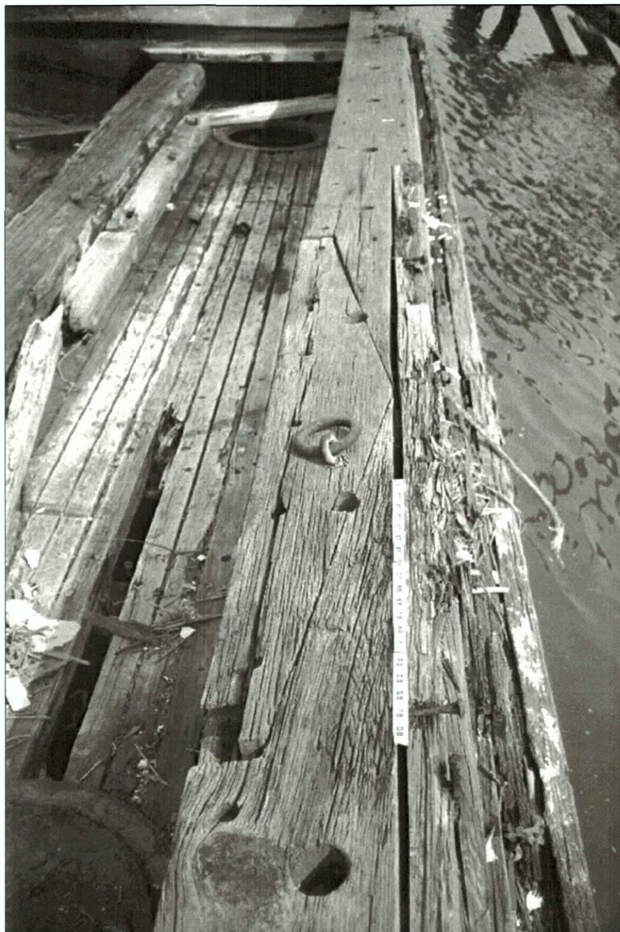
Figure 7-104. Scarph joint used to join sections of the starboard rail.
