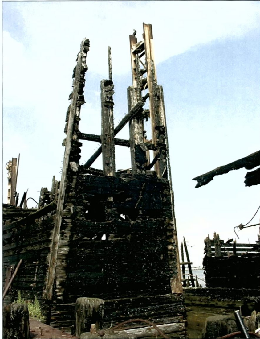
Figure 5-94. Aft end starboard wing. View to the northeast. Note angled inner wall.
