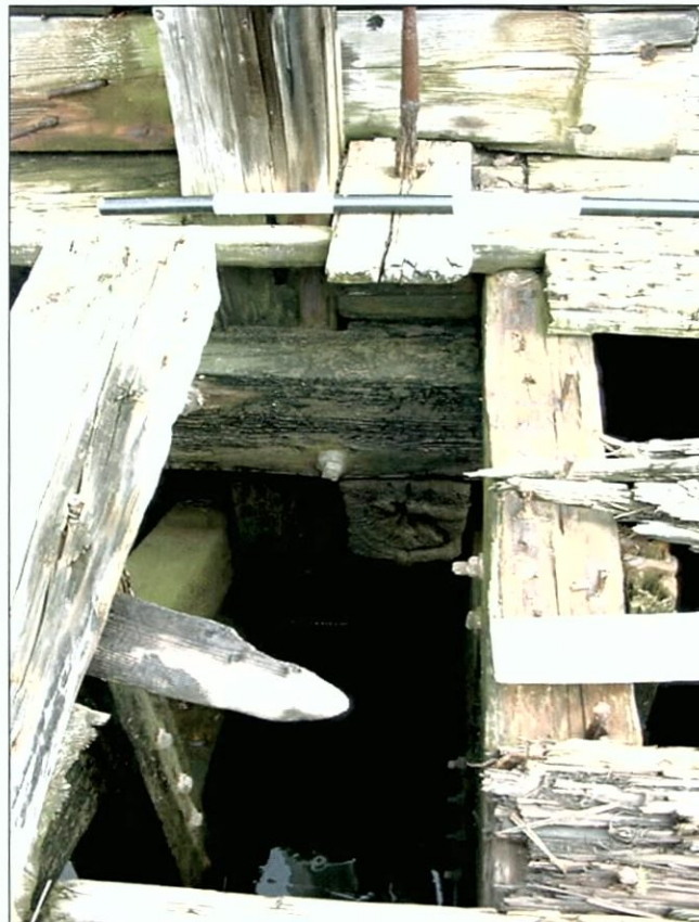
Figure 5-74. Detail of structure of aft starboard bitt showing stringers and, directly below, transverse bracing. View to the east (starboard).
