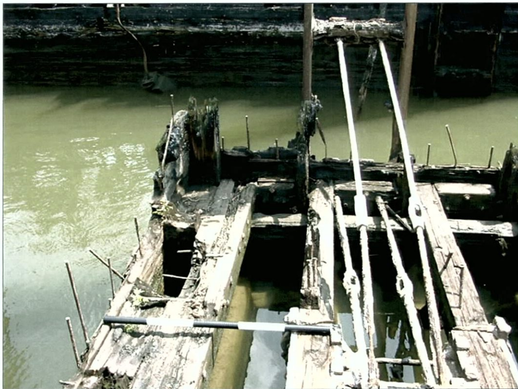
Figure 5-38. Northern exposed end of V1, showing top corner construction. View to the east (starboard).
