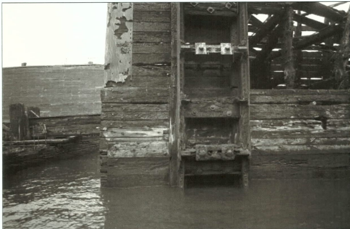
Figure 5-27. Aft starboard quarter, showing transition from the thicker planking of the pontoon to the thinner planking of the wing.
