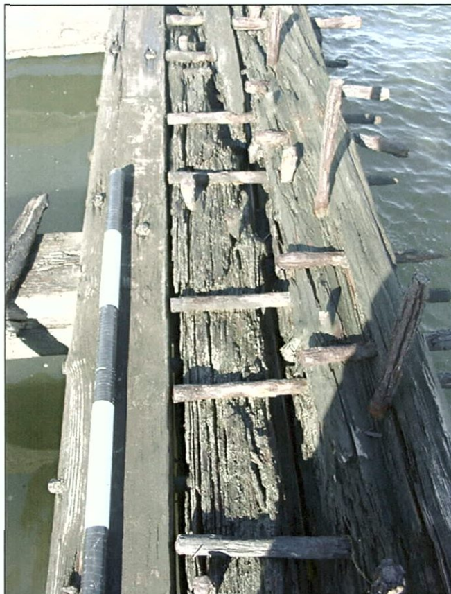
Figure 6-94. Port side view aft (north) showing three-timber waterway of cargo deck. Note pattern of fasteners.
