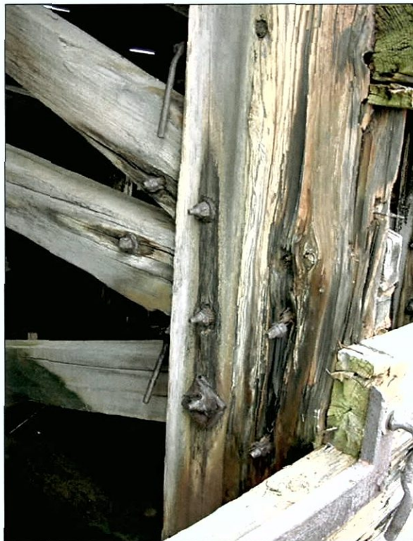
Figure 5-108. View of wing frame directly forward of frame in Figure 5-107, but showing opposite side. View to the north (forward).
