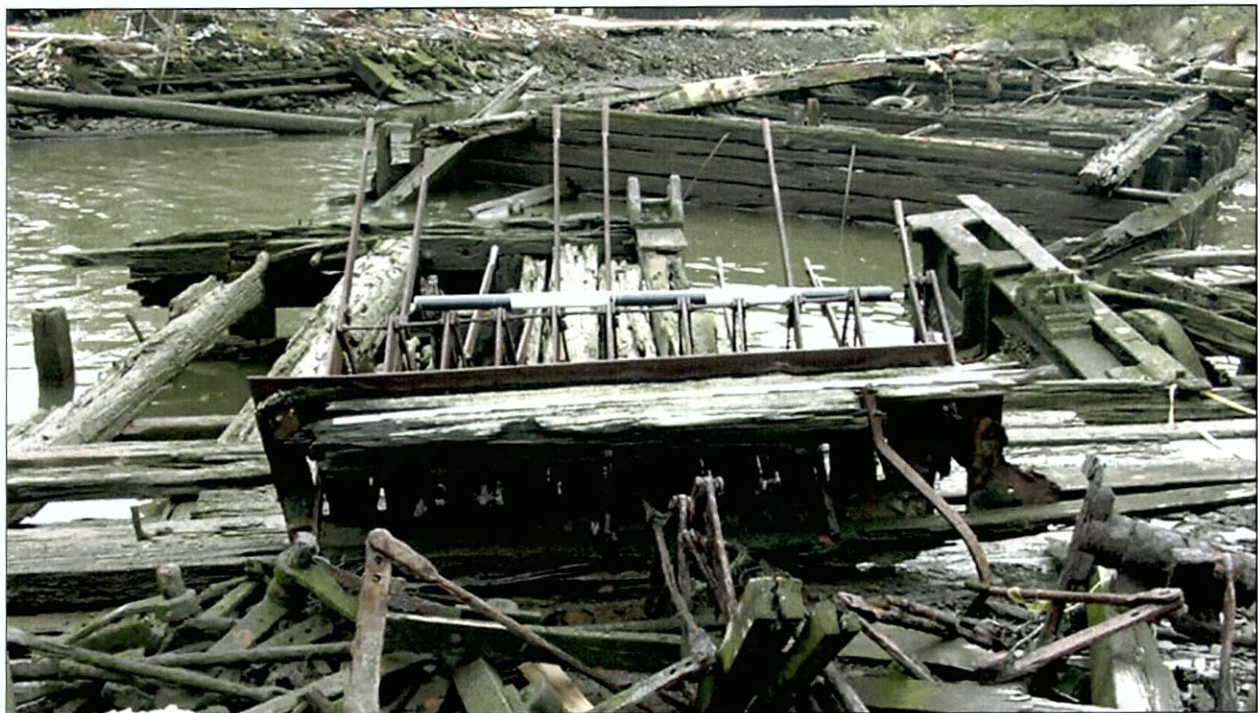
Figure 4-59. Hoisting drum control box. View to the north (aft).
