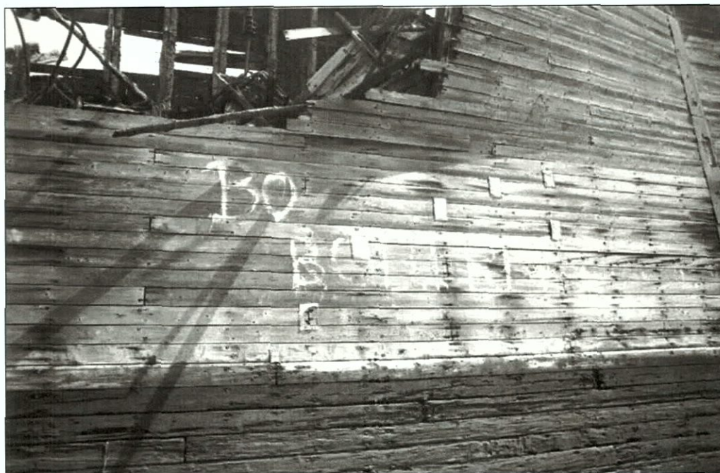
Figure 5-170. Port wing showing tin patches covering plank joints. View to the southeast (starboard).
