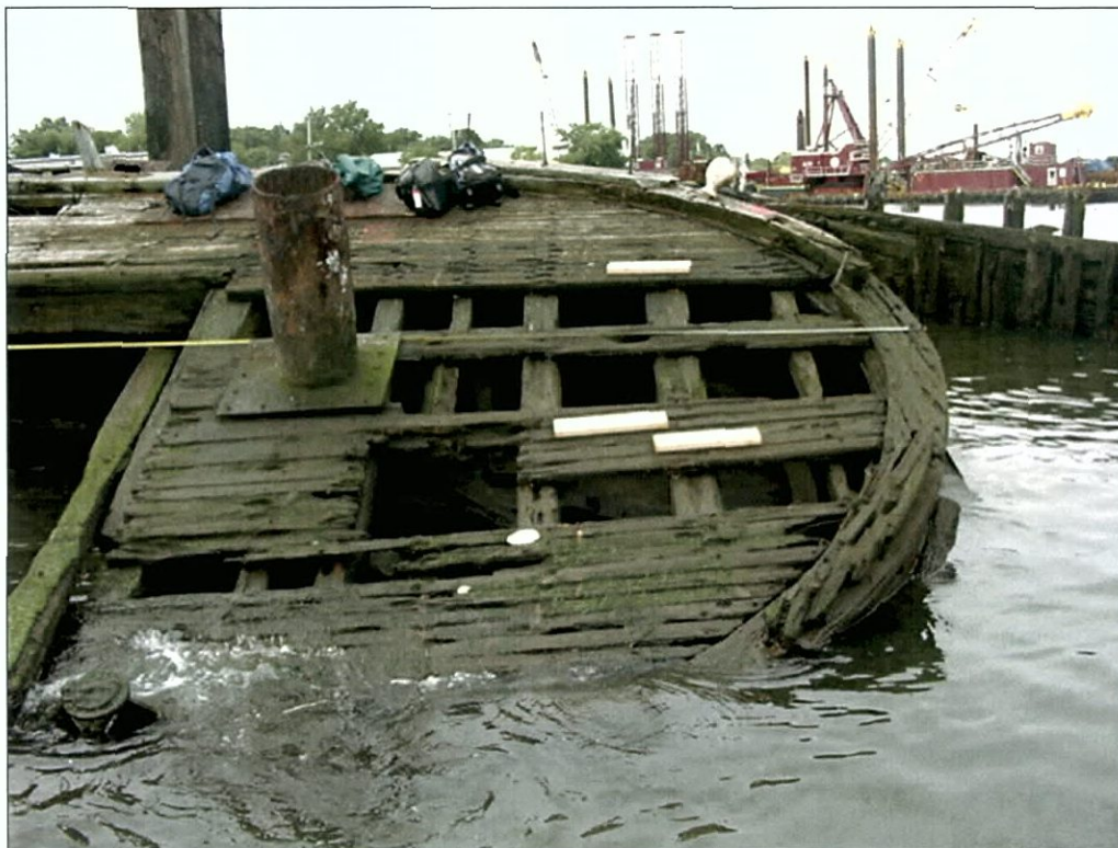
Figure 7-46. Fish Hawk fantail assembly from port side, looking west.
