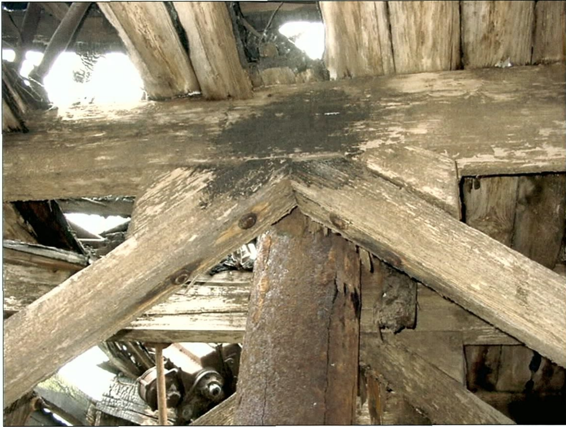
Figure 5-116. Second wing deck beam. Note chocks and fasteners. Starboard wing. View to the north (forward).
