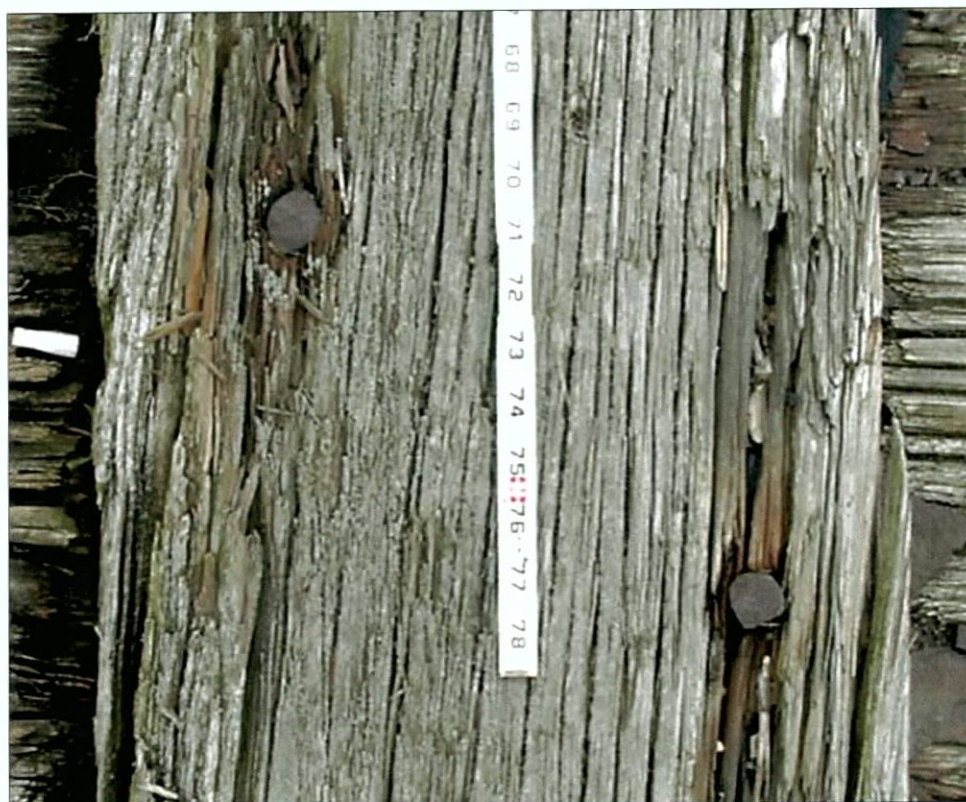
Figure 5-83. Bilge block stringer fastener pattern detail.
