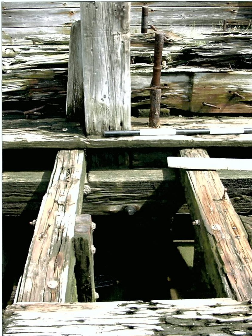
Figure 5-72. Starboard aft bitt structure showing vertical bitt and longitudinal stringer. View to the east (starboard).
