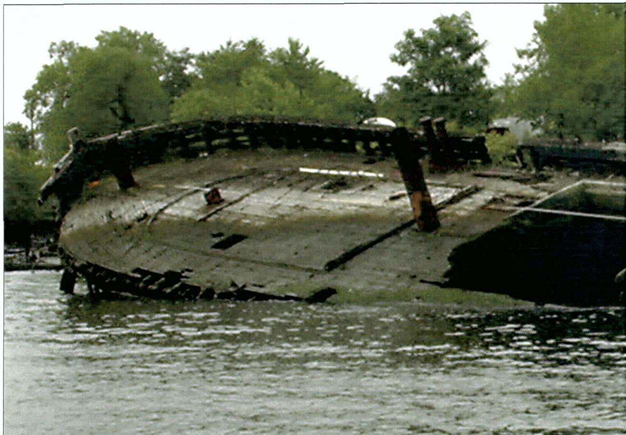
Figure 7-70. Forward third of Fish Hawk , including pilothouse, looking south. Note king plank and sisters along centerline.
