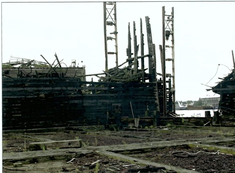
Figure 5-86. Main deck looking starboard (southeast). Note location of drains, bottom center.
