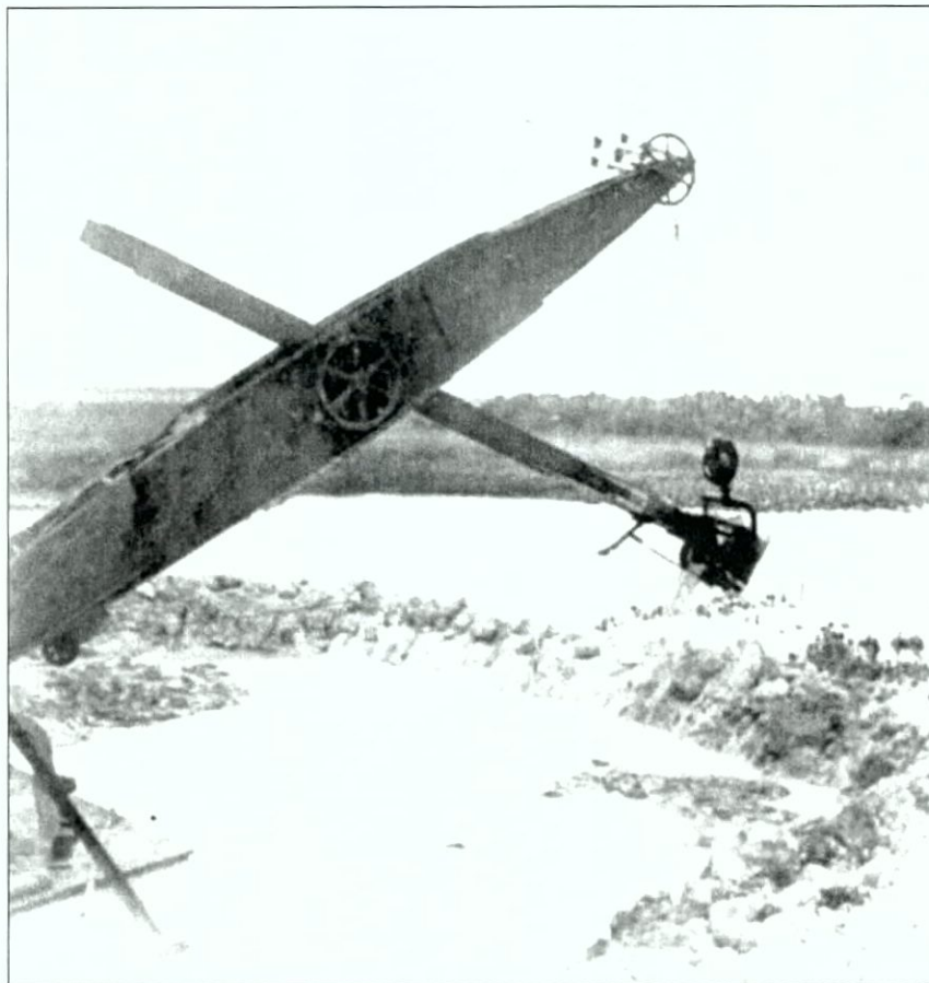
Figure 4-04. Close-up of bucket dredge Miami at work on the Miami River, circa 1910 (photo courtesy of the Florida Photographic Collection).
