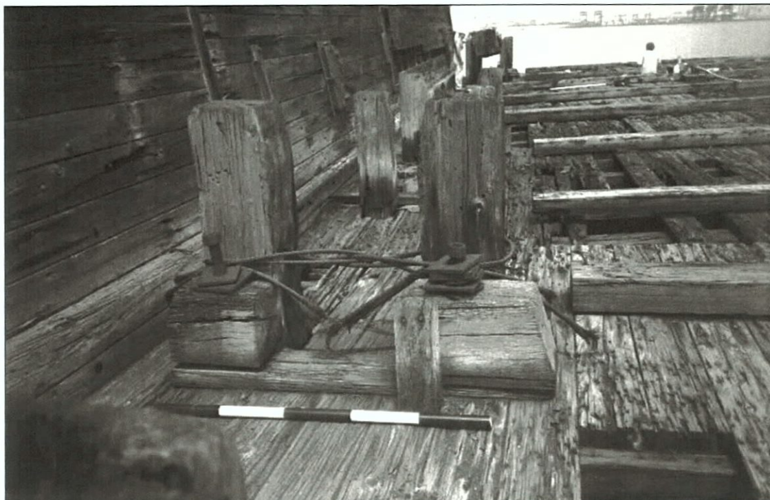
Figure 5-68. Bitt cradle. View to the north (forward).
