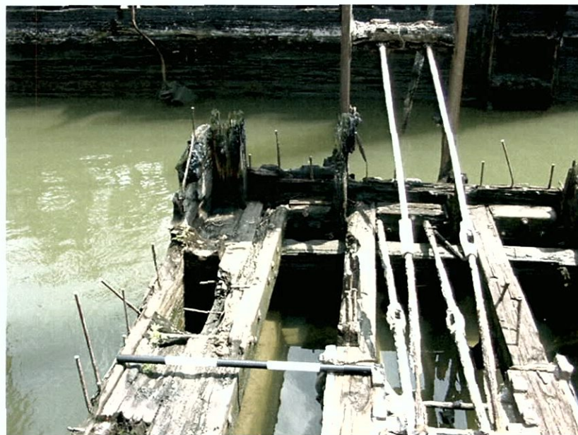
Figure 5-168. Anchor and turnbuckles for starboard forward spud on V1. View to the east (starboard).
