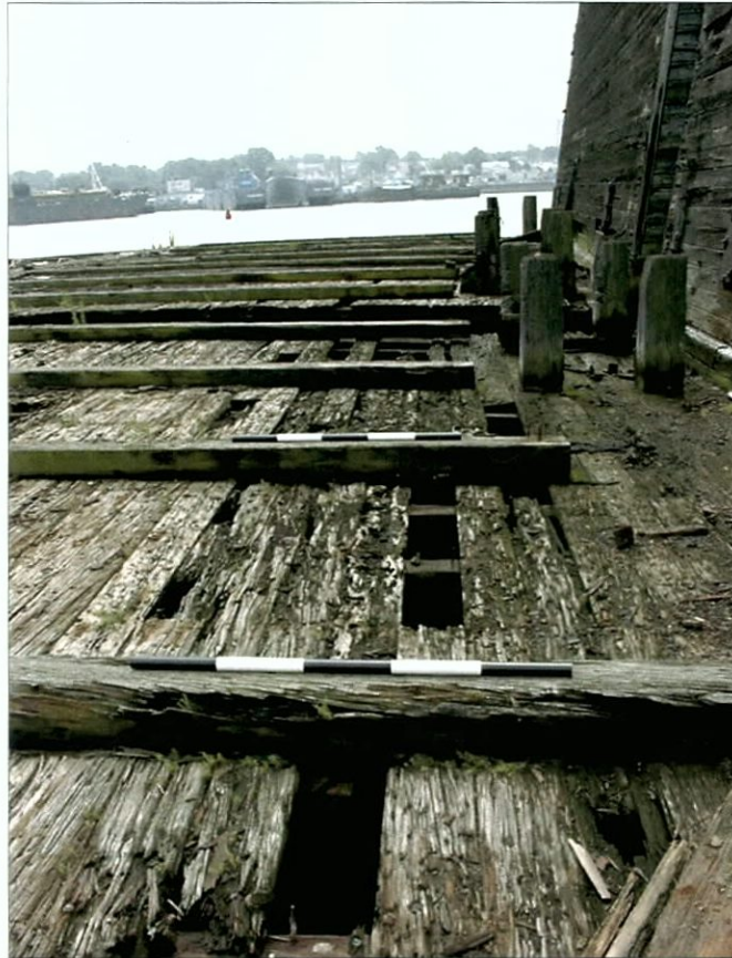
Figure 5-41. Main deck. View to the south (aft). Note exposed deck beams.
