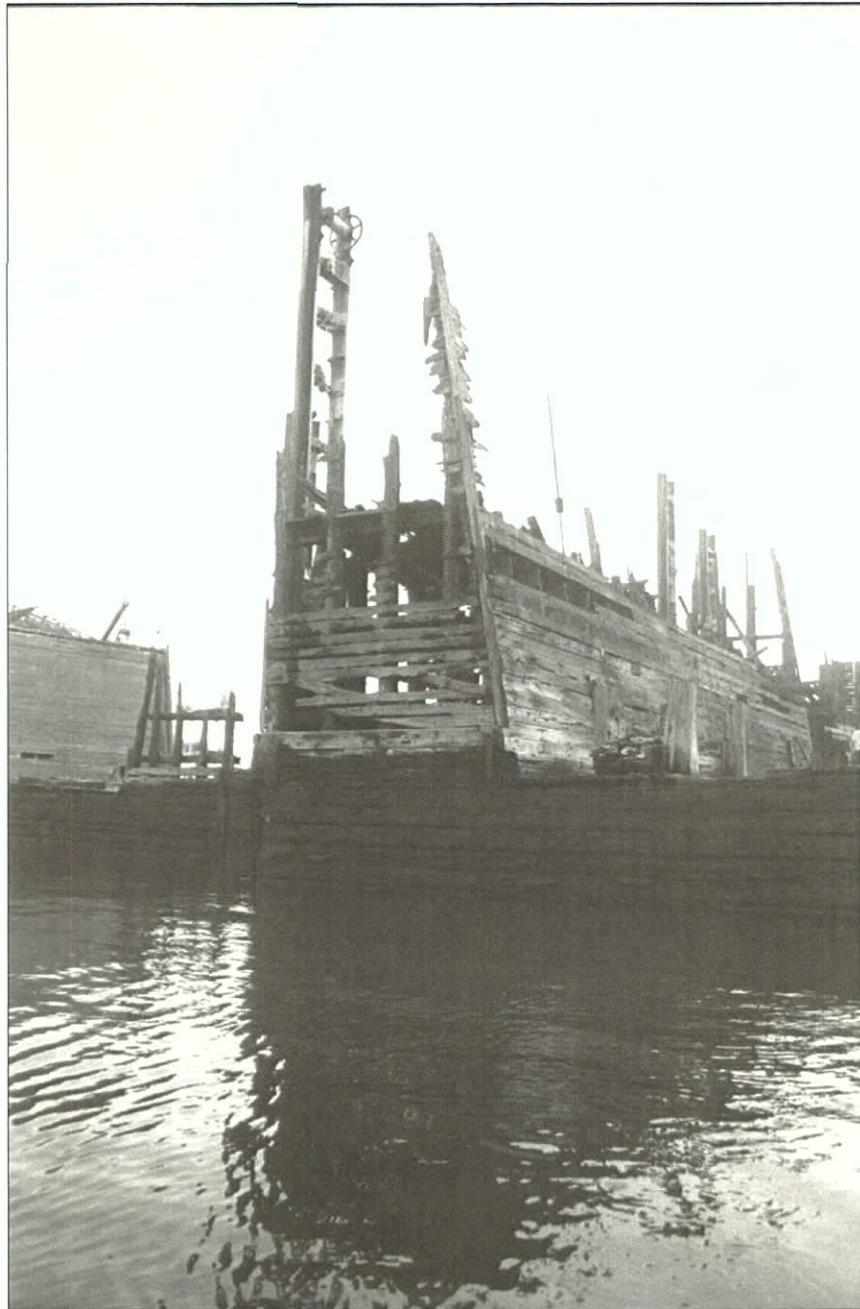
Figure 5-164. Starboard wing showing spuds. The rightmost spud belongs to another dock. View to the northeast (starboard forward).
