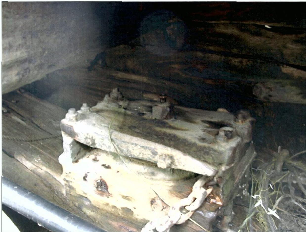
Figure 7-105. Starboard steering pulley, looking southwest.
