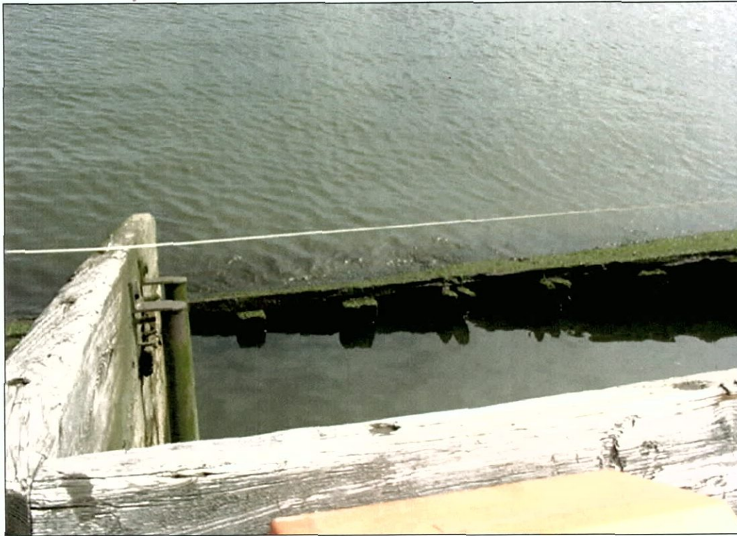
Figure 7-59. Exposed main deck beams along port side of main cargo hatch, looking east.
