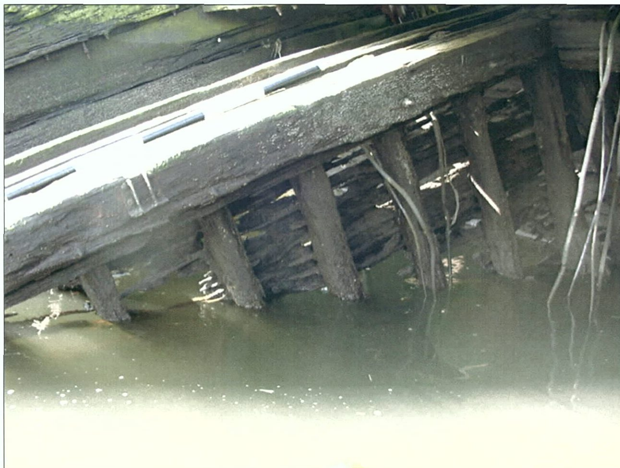
Figure 7-65. Detail of aft bulkhead showing stanchions and facing planks, starboard side, looking south (forward).
