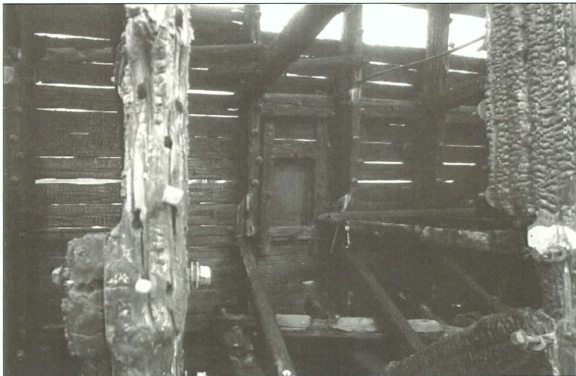
Figure 5-141. Small hatch reverse side. Starboard wing, view to the west (port).
