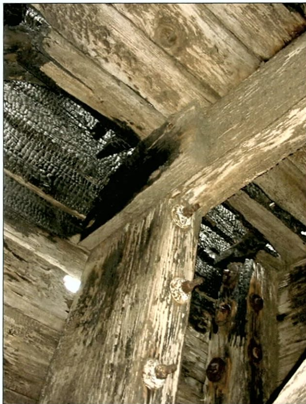
Figure 5-97. Outer wing frame at second deck, port wing.
