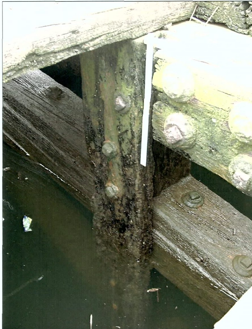
Figure 5-58. Main 16-inch laminated arched truss (T1). View toward southeast (aft starboard corner).
