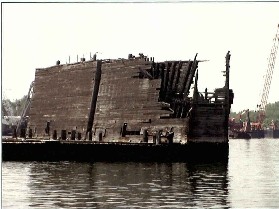
Figure 5-22. Main deck port side. View to the north.
