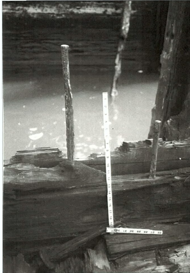
Figure 5-175. One-inch drift pins in outer hull timbers.
