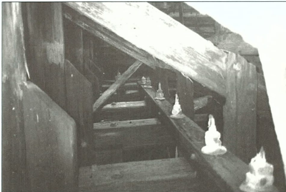
Figure 5-159. Longitudinal stringer providing stability to vertical supports, which, bolted to the wing truss, support the weight of the vertical discharge pipe. Note vertical tie rods, which fasten the stringer to the pontoon framing. Port wing, view to the north (fore).
