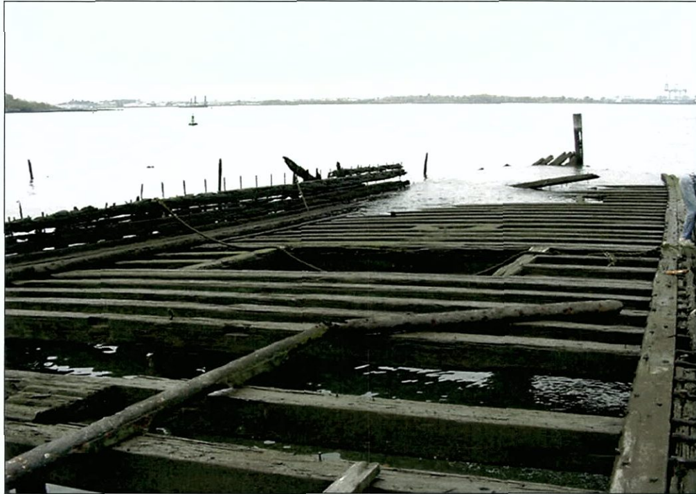
Figure 6-84. Cargo deck. View to the north. Note sternpost, left center.
