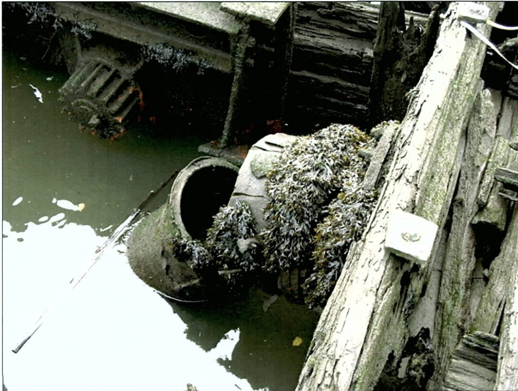
Figure 4-45. Remains of suction pipe. View to the southwest (starboard).
