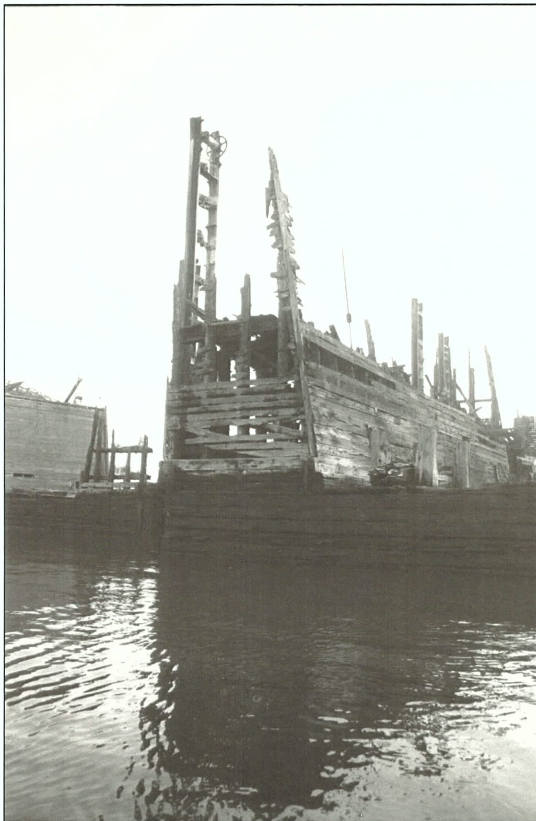
Figure 5-23. Main deck starboard side. View to the south.
