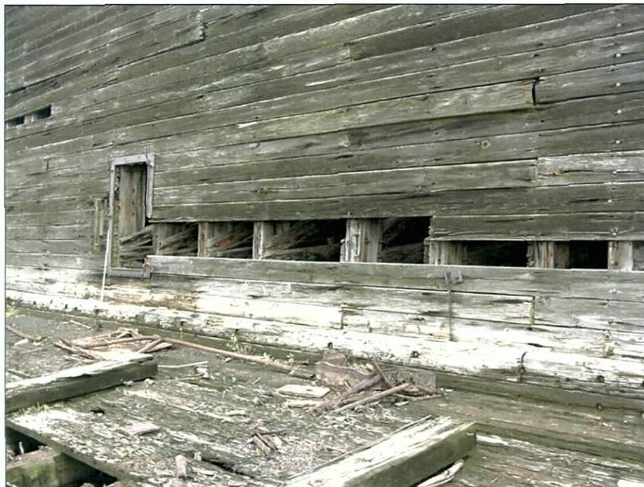
Figure 5-119. Port wing showing wider inner wing plank below level of middle deck. Note also chine logs. View to the southwest.
