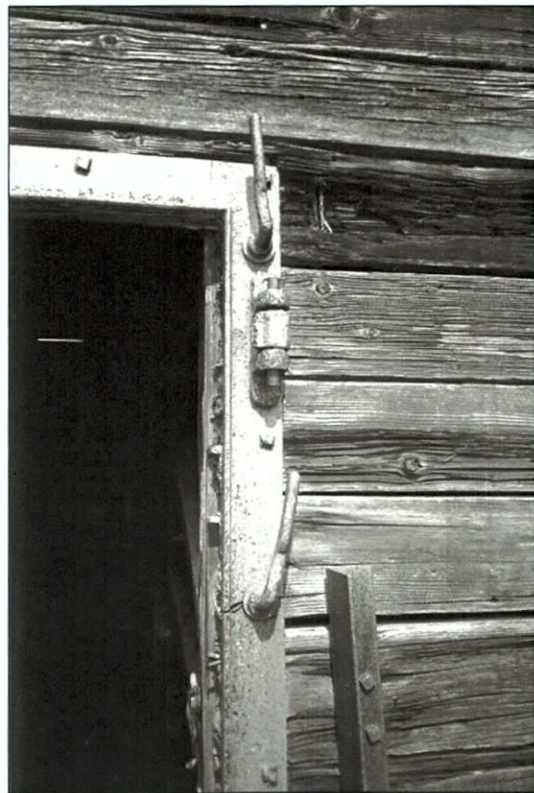
Figure 5-138. Hatch frame detail. Note hinge, hatch dogs, and fasteners. Port wing, view to the west.
