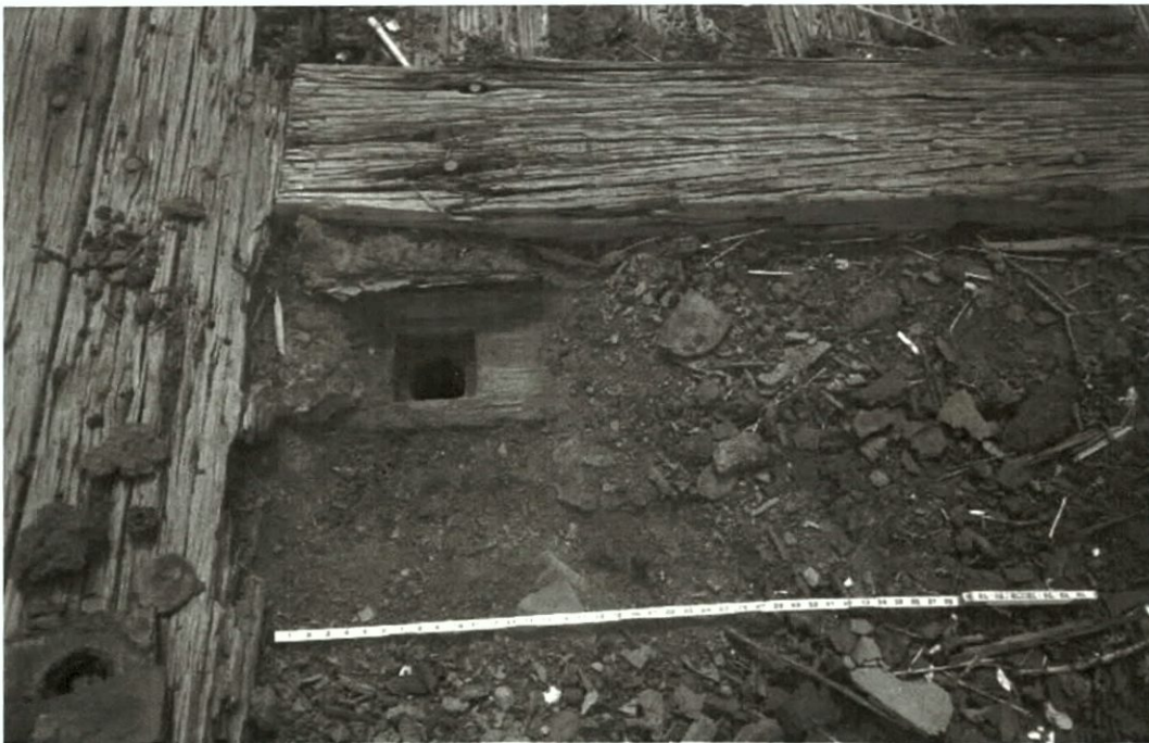
Figure 5-85. Deck drain with cover and straining screen removed. View to the south (aft).
