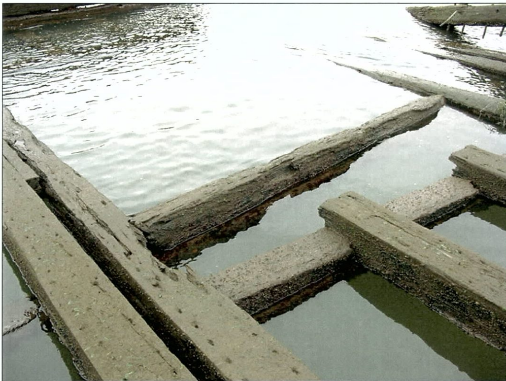
Figure 6-91. Detail of foreward cargo hatch with separated carling. Note notching of partial deck beams into carling and over rider carling. View to the northwest.
