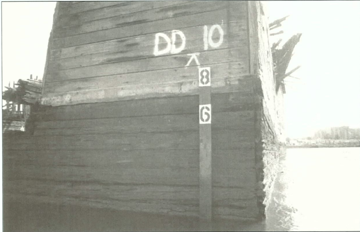
Figure 5-26. Port forward corner, view to the south, showing thicker pontoon planking.
