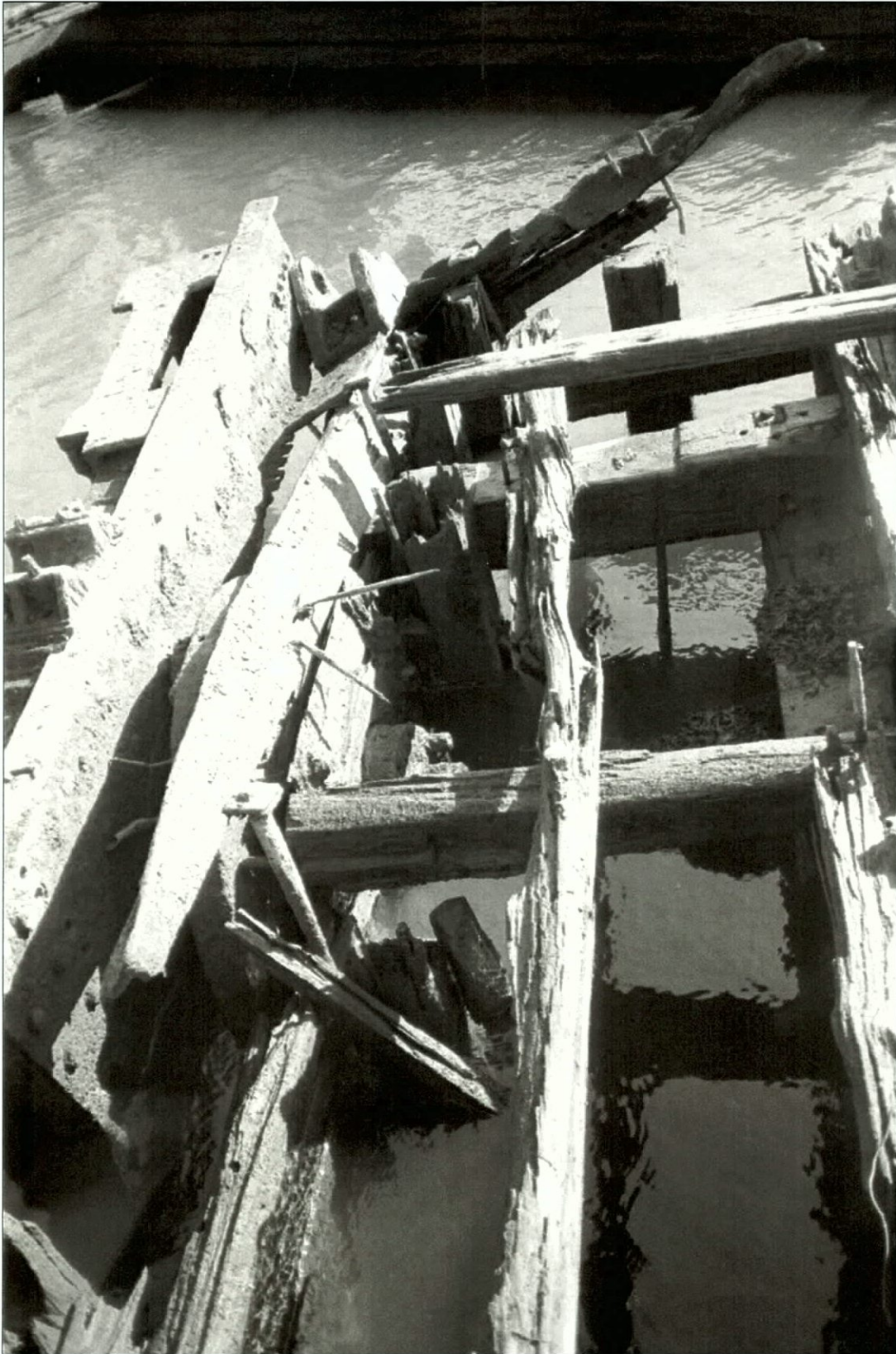
Figure 4-36. Starboard hull extension framing. View to the south (forward).
