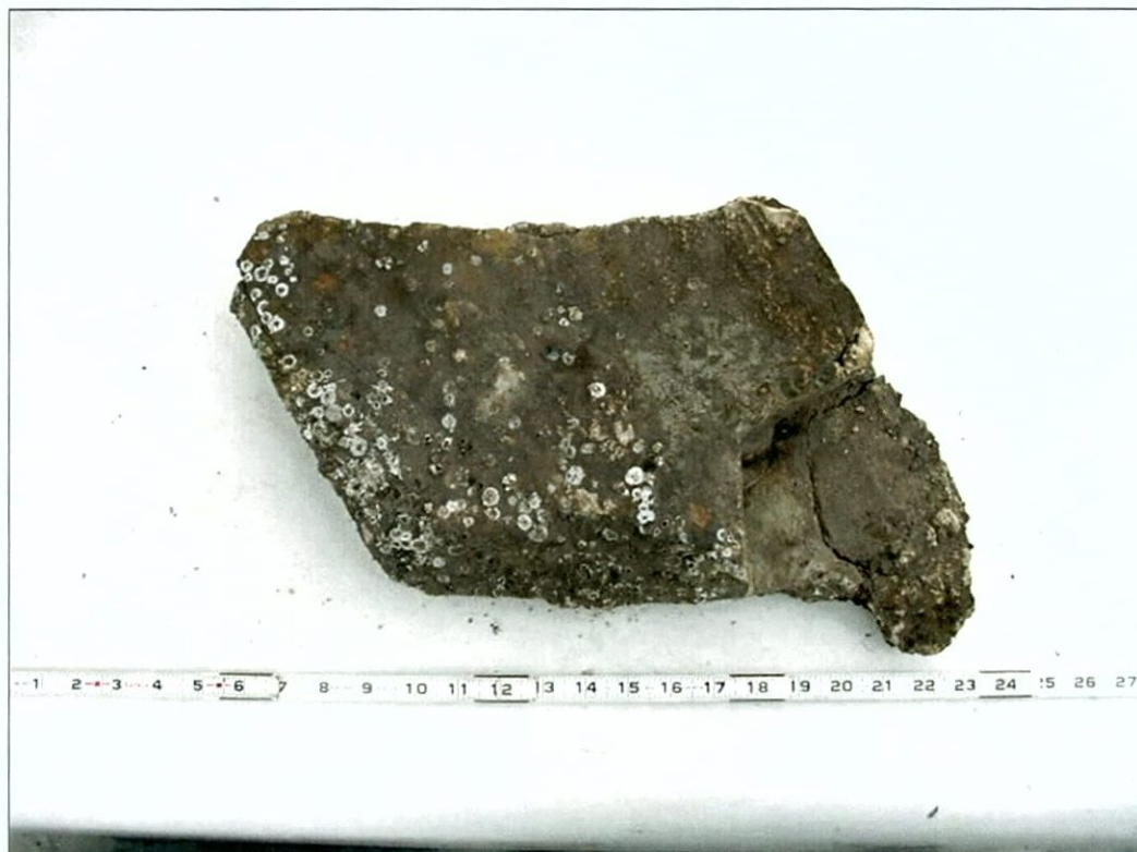
Figure 8-31. Section of concrete boiler bed.
