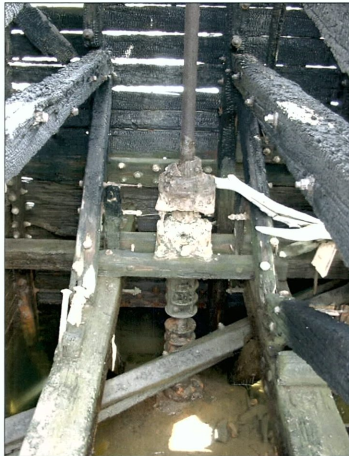
Figure 5-153. Impeller drive shaft.
