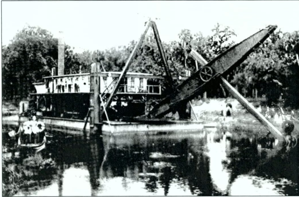
Figure 4-03. Bucket dredge in operation on the Caloosahatchie River, circa 1909 (photo courtesy of the Florida Photographic Collection).
