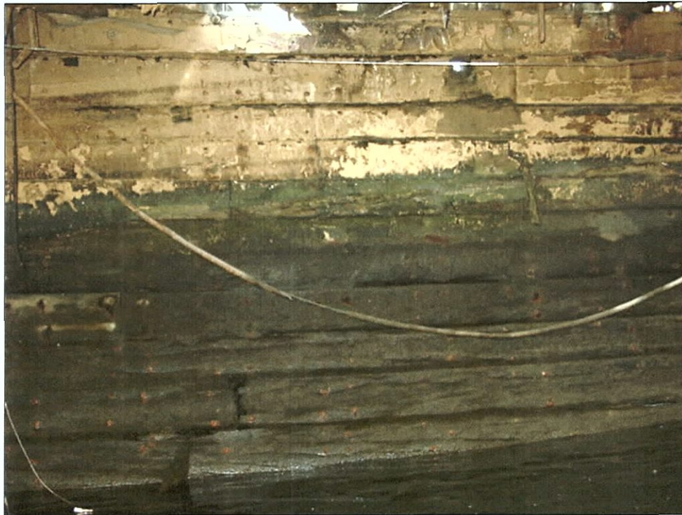
Figure 6-67. Close-up of ceiling planking in crew compartment, looking starboard (west). Note tan paint.
