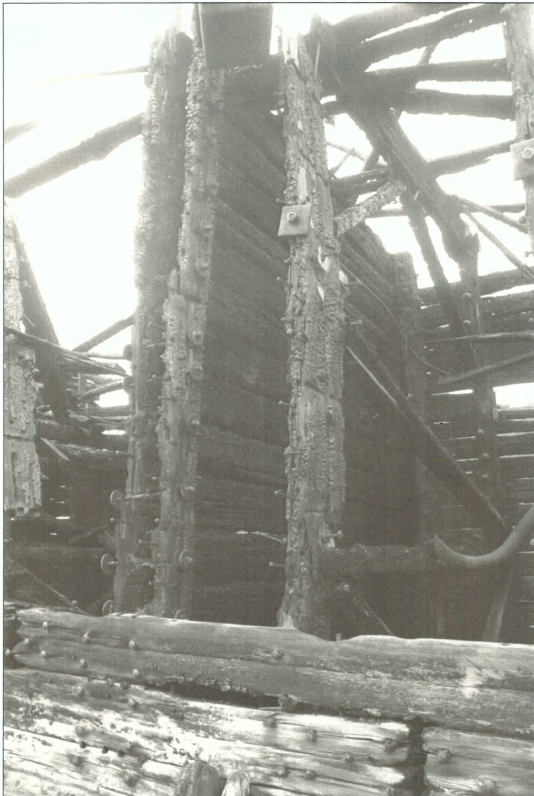
Figure 5-44. View of forward side of watertight bulkhead in starboard wing. Pontoon bulkheads are of similar construction.
