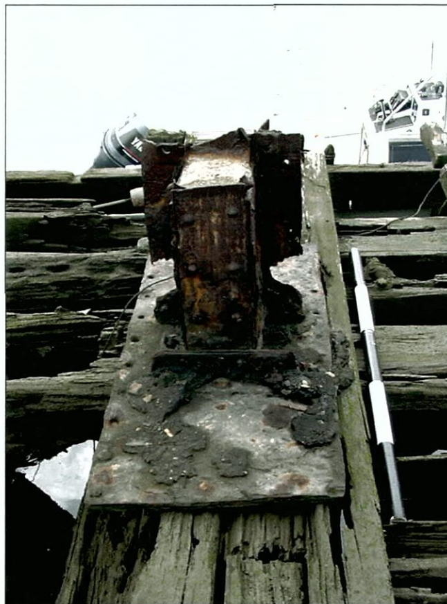
Figure 4-49. Starboard H-frame mount. View to the west (starboard).
