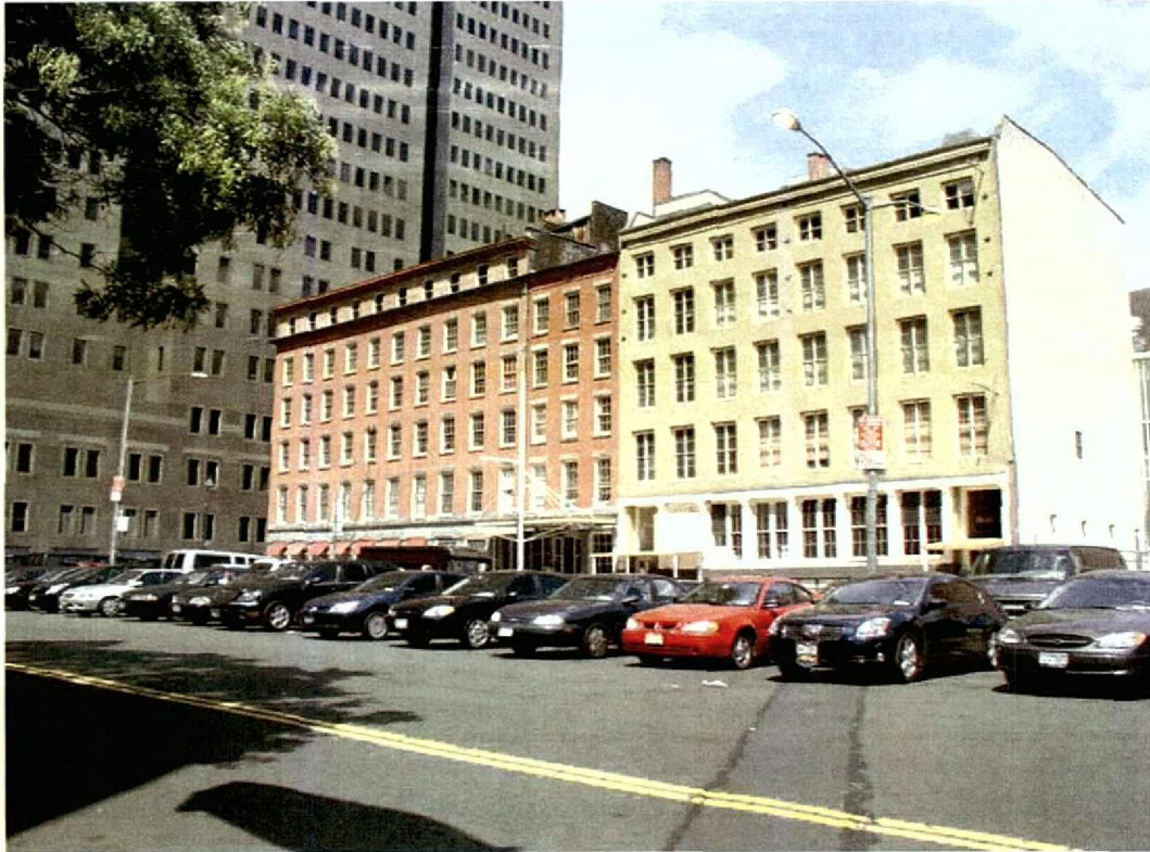
Photograph 1: Burling Slip APE facing north from the corner of South Street and John Street. Note: John Street is in the foreground.
