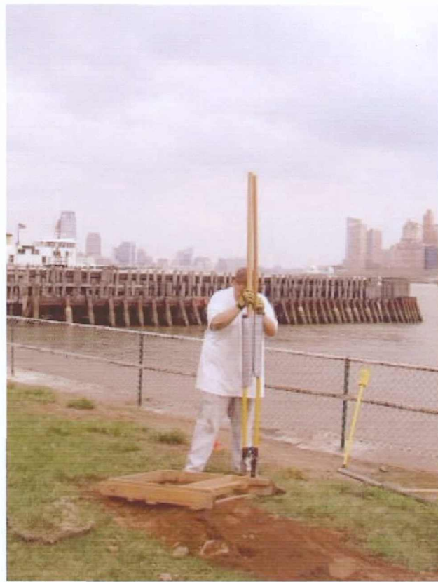
Photo 1 EP 5 in progress, facing northwest.
