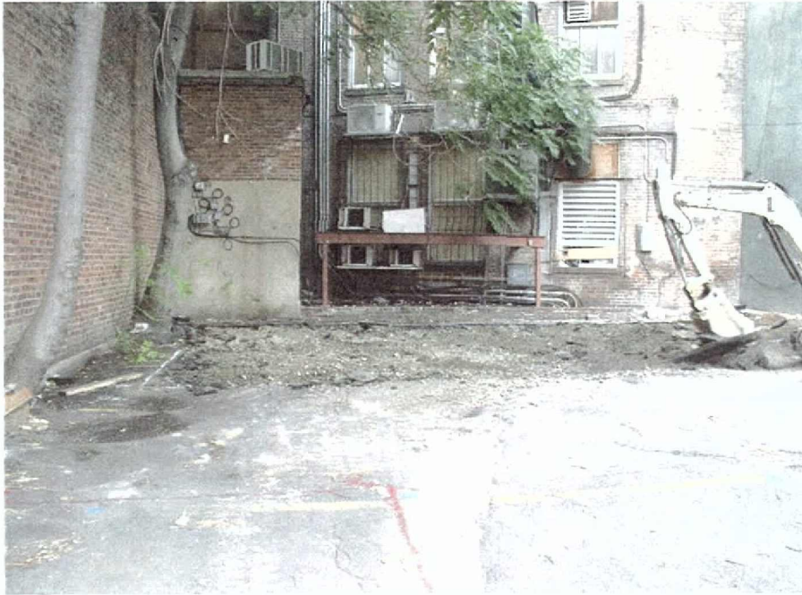
Photograph A. View of the 240 West Broadway Project Site, facing north.
