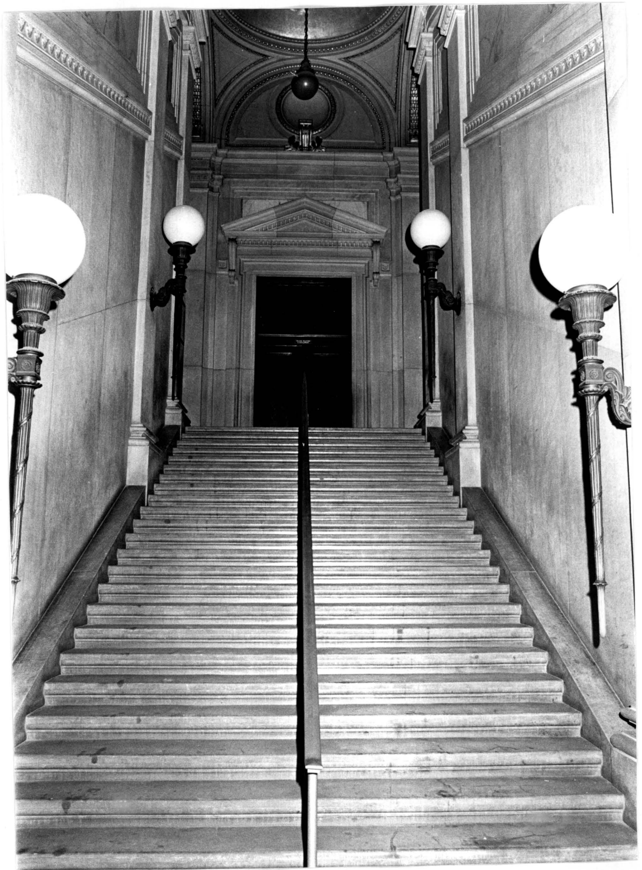
GOULD MEMORIAL LIBRARY MAIN STAIRCASE Former New York University Campus, University Heights, The Bronx
