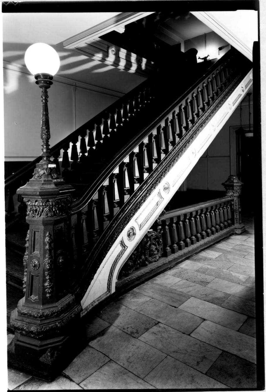
TWEED COURTHOUSE INTERIOR detail, west stairway, first floor
