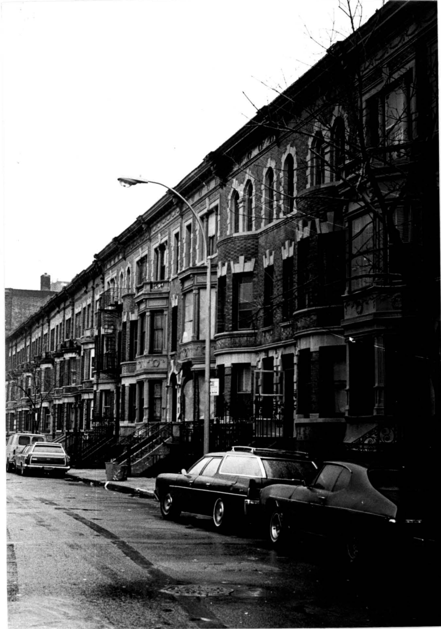
Forest Avenue, west side, between between East 166th Street and Home Street Photograph: LPC
