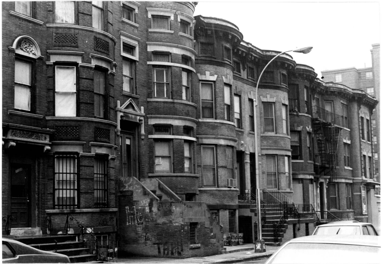
Jackson Avenue, east side, between East 166th Street and Home Street Photograph:LPC
