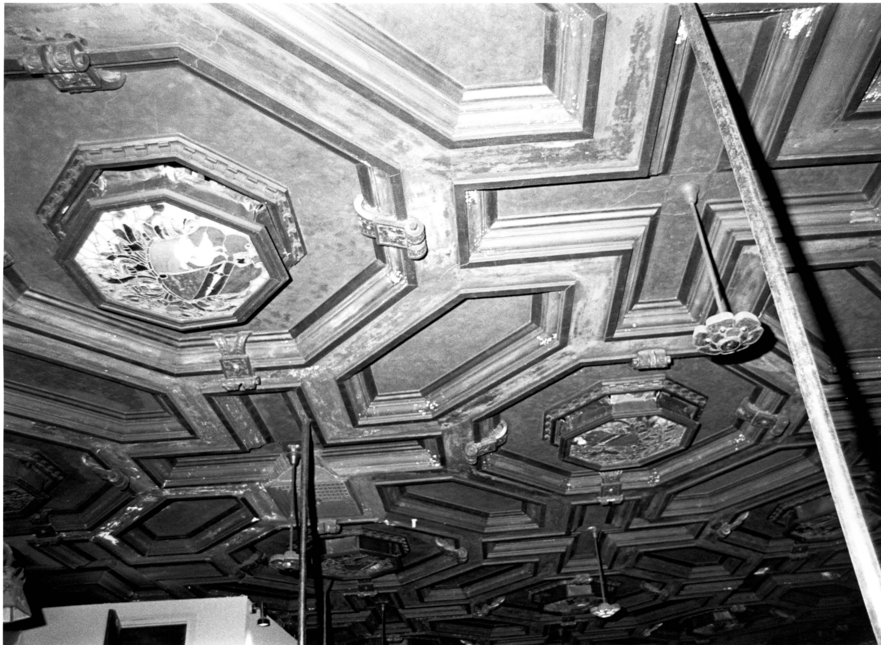
Belasco Theater Interior Ceiling
